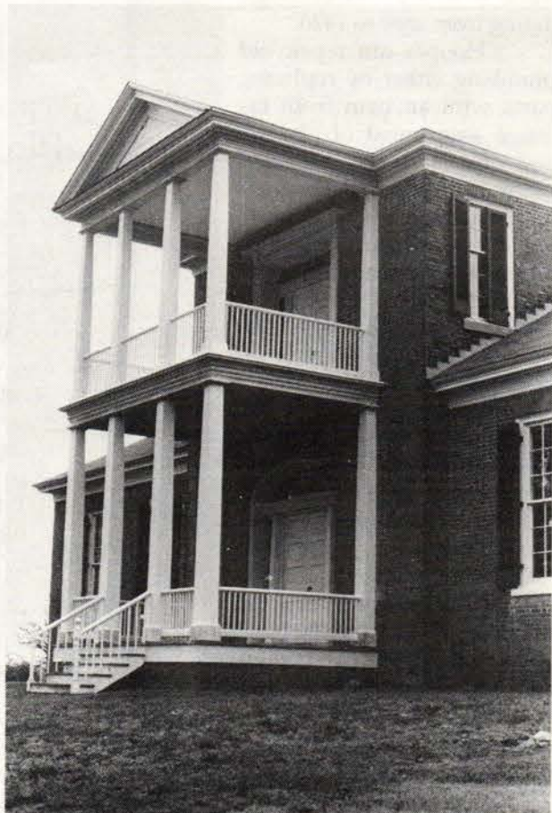
The Belle Mont portico was pulled back from the brink of collapse. Wherever possible, original material was kept — and repaired or patched as necessary.
