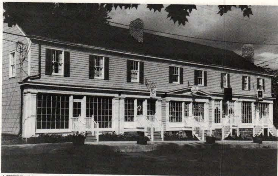
AFTER: New wood windows, storefronts, and millwork were custom-produced to Meadows' drawings by Millwork Specialties of Brooklyn, N.Y., preserving the traditional character of the building.
