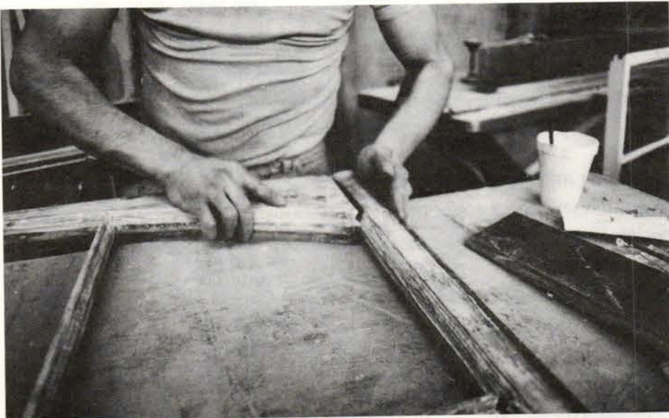
Loose joints were taken apart, glued with epoxy, and repinned. Rotted or damaged wood was restored with epoxy consolidant and filler. When an individual rail was beyond repair, a new "dutchman" was spliced in. If more than 35% of a sash was beyond repair, a whole new sash was manufactured.
