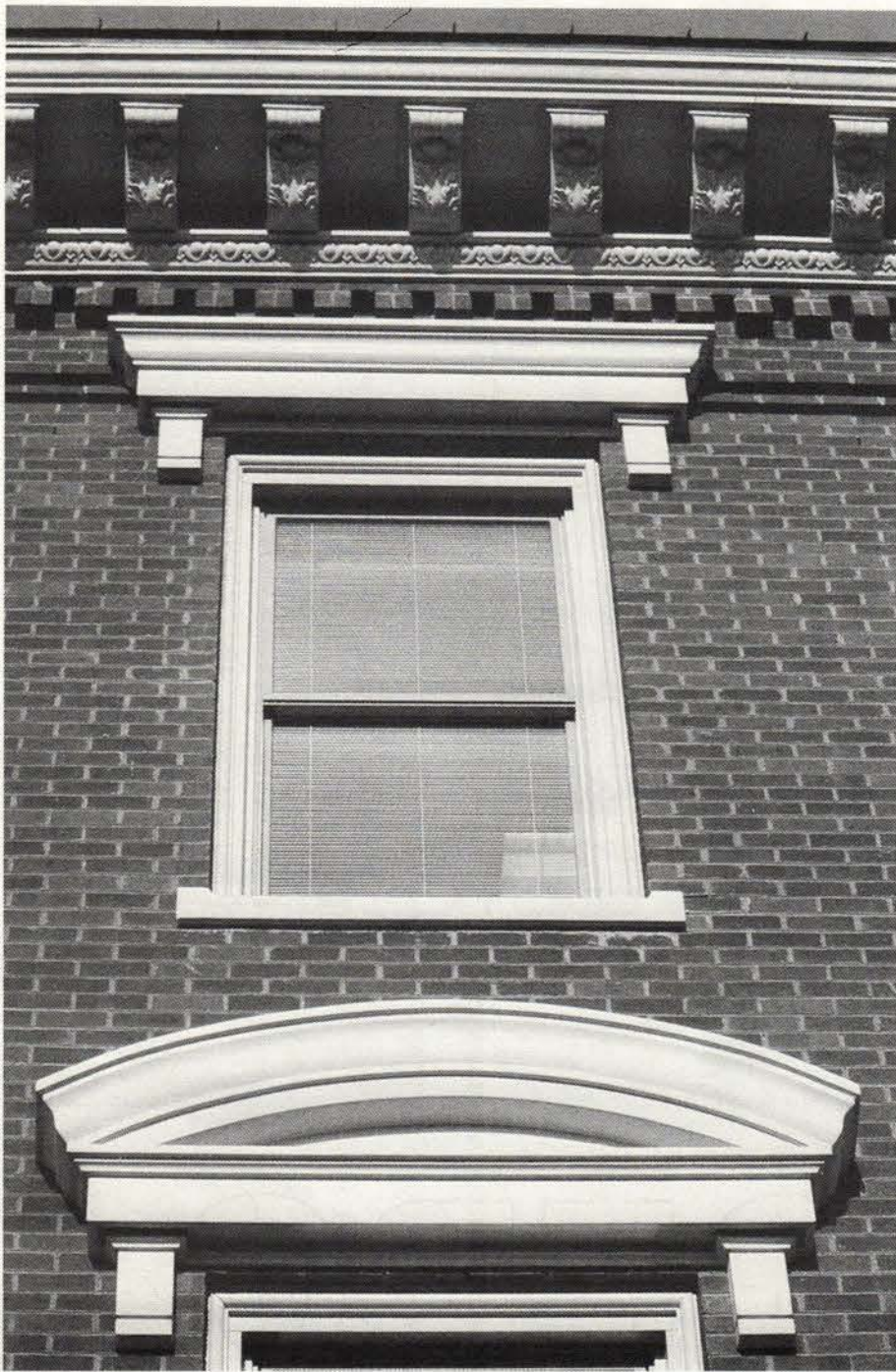
For this exterior restoration, window hoods and cornice were replicated in white FRP by FIBERTECH CORP.
