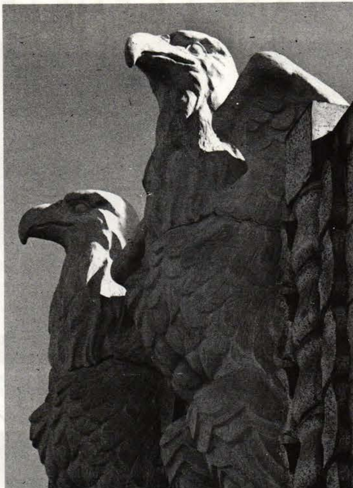
These 13-ft. eagle sculptures were recreated by Manuel Palos from 1924 drawings of the originals that once adorned the Pacific Telephone Building in San Francisco. Weighing only 1,500 pounds (half as much as the terra cotta originals), these enormous creatures were cast in fiberglass and framed with reinforced stainless steel.
