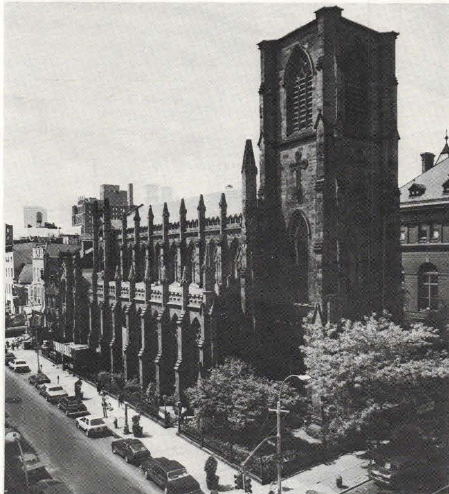
The Church of St. Ann and the Holy Trinity (1847) has lost, among other things, its original 100-ft. spire and numerous crockets and finials because of sandstone deterioration.
