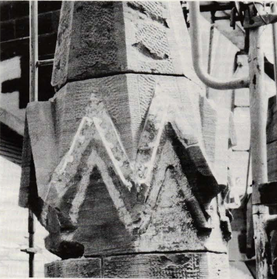
Workers remove deteriorated stone using hand-held hammers and chisels along with the same pneumatic carving heads they use to rake mortar joints for repointing. They then drill the stone wherever armatures will be required.
