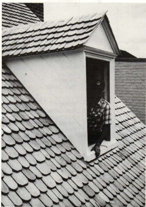
A roof restoration with 3/4-in. thick, 18" long, round butt, Tidewater Colonial Shingles custom-cut in white oak by Shamokin Trail Shingle Co.
