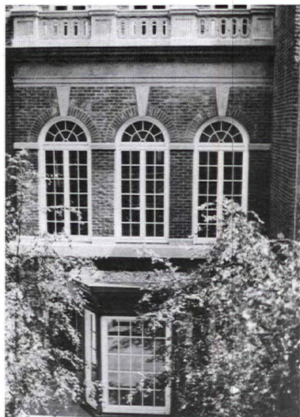
The rear elevation, which overlooks the back garden, uses carved limestone elements to punctuate the red brick. A copper-sheathed bay window provides additional space and light for the ground floor
