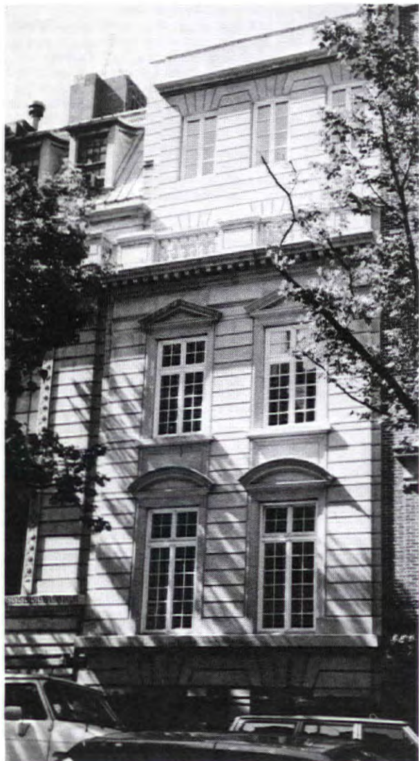
The new Indiana limestone facade as construction is being completed. Carved stone elements are set in a thin mortar bed — and held to the front wall with stainless steel anchors
