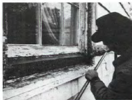
Craftsman from CONSERVATION SERVICES applies epoxy repairs to a badly deteriorated windowsill and frame. Write in No. 175
