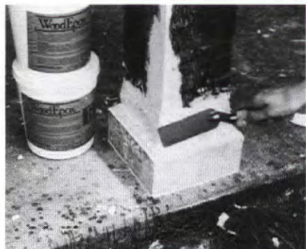
ABATRON's WoodEpoxy rebuilt the base of this timber column. Write in No. 130
