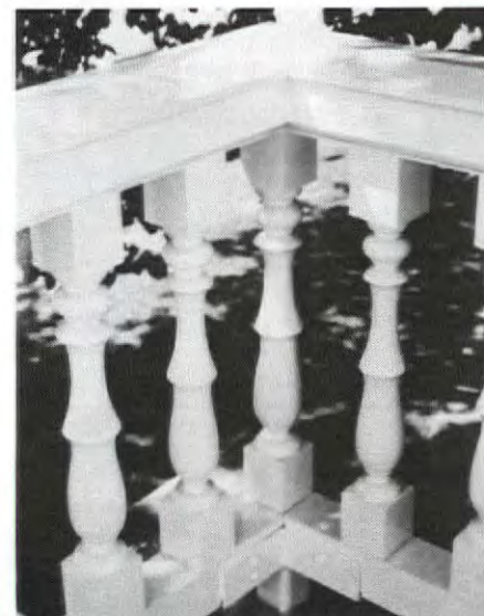
Close-up of balusters recreated as part of the reconstruction of the Hamilton County Bandstand in Aurora, Nebraska. SACO MANUFACTURING & WOODWORKING
