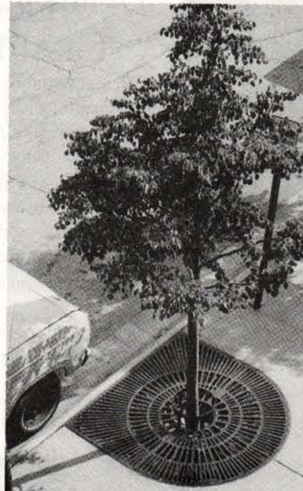
NEENAH FOUNDRY's tree guards and grates range from utilitarian to High Victorian and are designed to accommodate tree expansion.
