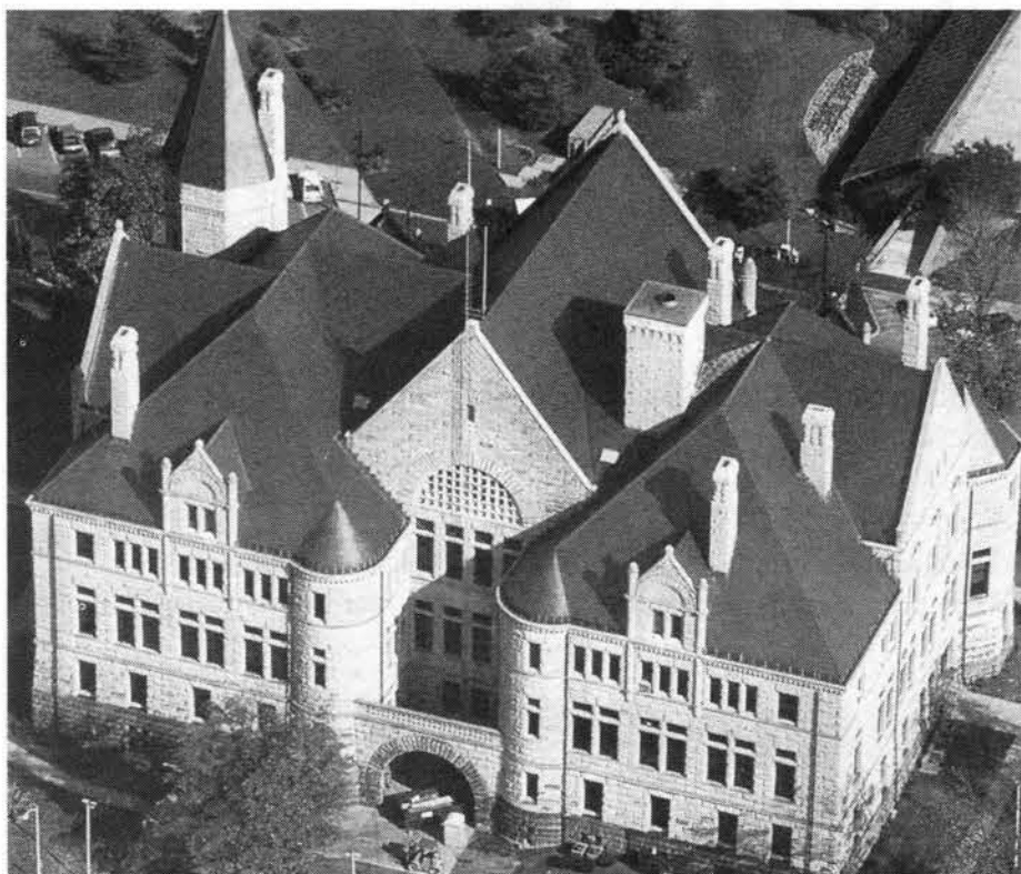
Complete restoration of the roof of the Wayne County Courthouse — including new Vermont slate, sheet metal, structural carpentry, masonry, and lightning protection — was carried out by workers from MIDLAND ENGINEERING. Write in No. 742
