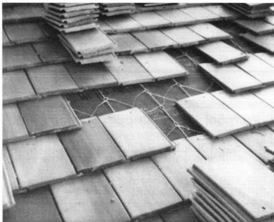
The twisted-wire "Tyle-Tye" system from NEWPORT FASTENER secures all types of roofing tiles to any type of roof deck material and any slope. Write in No. 391
