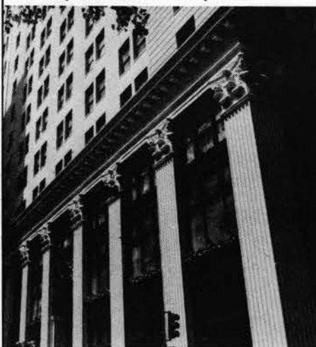
Restored facade of Widener Building. Capitals and horizontal ornamentation were made of fiberglass reinforced polyester resin in Polytek Rubber Molds.
