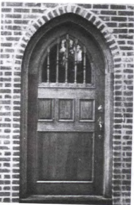
A custom-designed, Gothic mahogany door with Baldwin hardware, hand-turned spindles, insulating glass, insulated raised panels, and applied moldings. WOODSTONE COMPANY Write in No. 843
