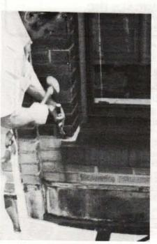
A craftsman from GENERAL RESTORATION CO. removes existing deteriorated sealant from construction joints, prior to recaulking with a longlife acrylic terpolymer sealant. Write in No. 238
