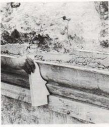
Exterior molding is repaired with Conpro-set — a polymer-modified all-purpose patching cement that can be shaved to final form. CONPROCO makes a wide range of masonry repair and restoration products. Write in No. 481
