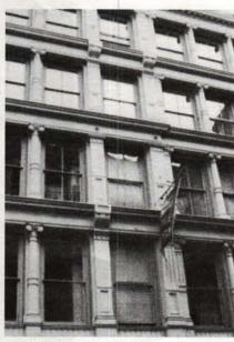
THE WOODSTONE CO. replaced all the weight-and-pulley, double-hung wood windows with true divided insulated glass in this landmark cast-iron building in NYC's Soho section. Write in No. 986
