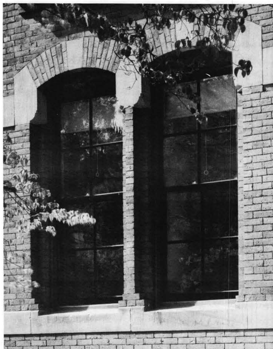
Architectural Components, Inc., fabricated this replacement window in Eastern white pine and mahogany sash, insulated glass, and 1-in. muntin bars for Weld Hall, Harvard University.
