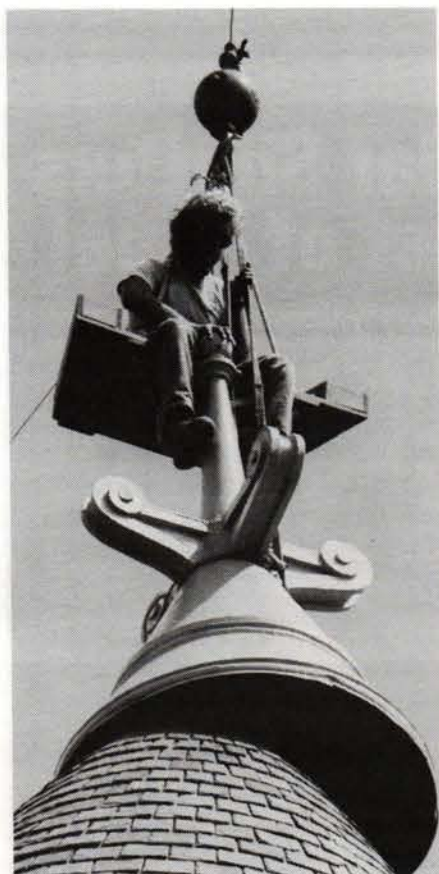
MIDLAND ENGINEERING CO. refurbished and reinstalled 4 turret caps at the University of Notre Dame's 1889 Sorin Hall. The sheet-metal caps, historic ornamentation that had never been properly maintained, suffered serious deterioration due to rust, bird excrement, and lightning. Write in No. 742
