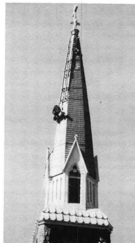
A steeplejack with The JACK HASSLER COMPANY replaces missing slate on the steeple of St. Dominic Catholic Church in Philadelphia.
