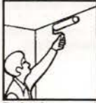
7. Apply second coat of saturant to wet mat
