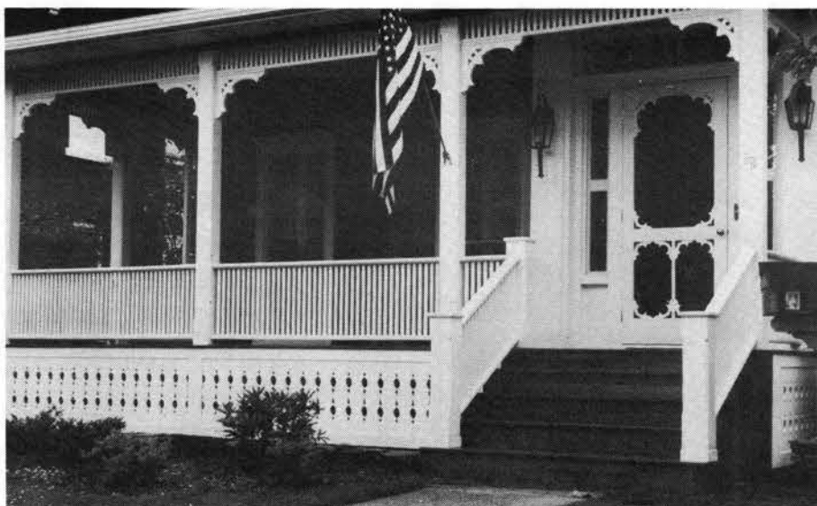
Complete porch parts were done by J.A. DAWLEY FINE WOODWORKING: Brackets and porch skirt were custom made; posts were splined, then chamfered; and the railing system was designed to direct water away from seams. Write in No. 420
