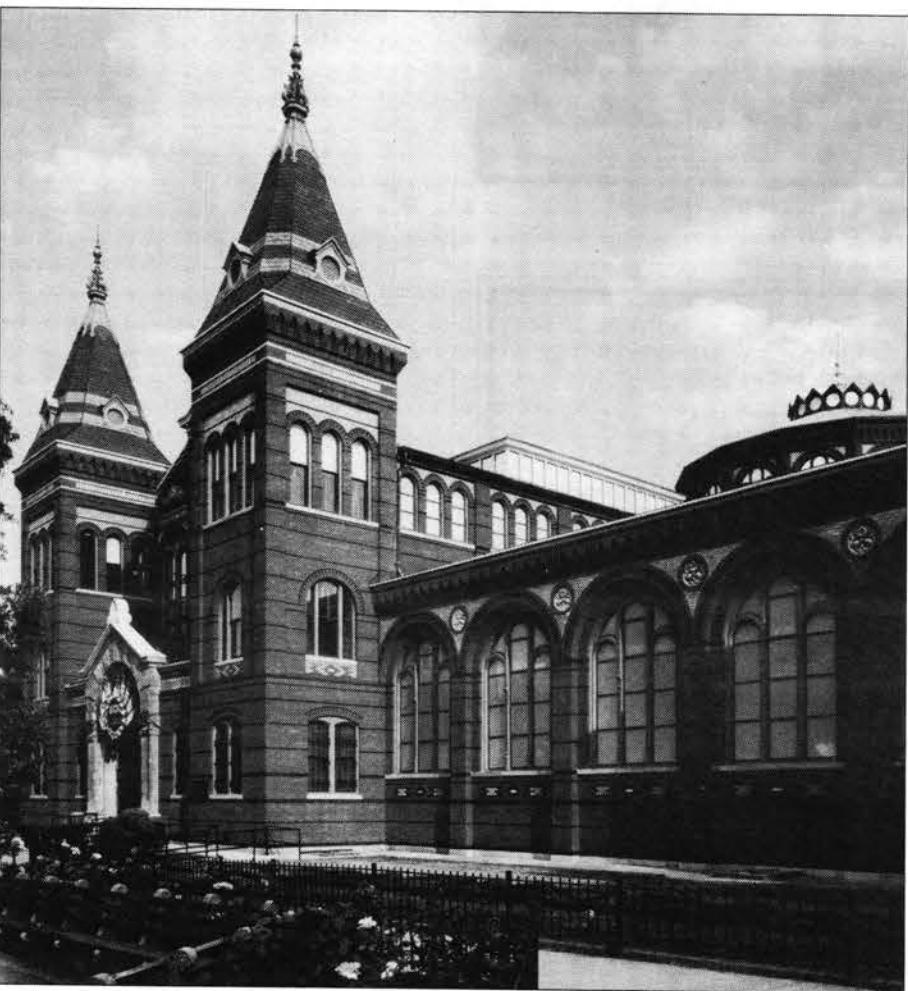
The $15 million renovation of the Smithsonian Institution's Arts and Industries Museum included roof replacement, masonry restoration, and replication of 500 windows. (Photo: Harlan Hambricht)
