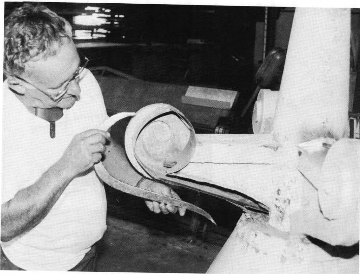
Inspection, maintenance, and repair of sheet metal ornament, such as this monumental tower finial, is part of an organized roof management program. (Photo: Midland Engineering)
