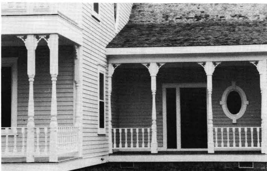
The above porch turnings were duplicated by CINDERWHIT & CO. from an original period design. Write in No. 788
