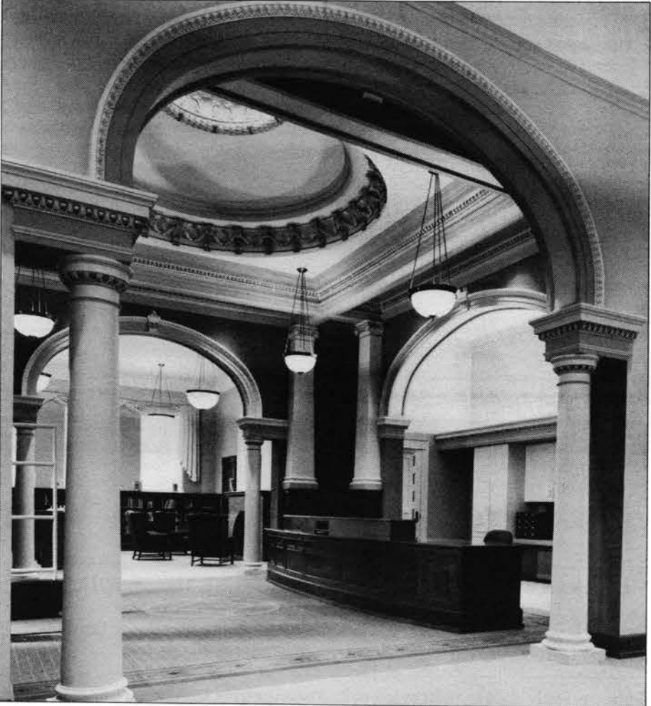
The 16-foot columns and other plaster details at the 1906 Howell Carnegie Library in Howell, Michigan, had all been either removed or water damaged and had to be recreated, and a triple switch-back handicapped ramp was added to the facade to maintain this rotunda as the main entryway. (Photo: Fred Golden)
