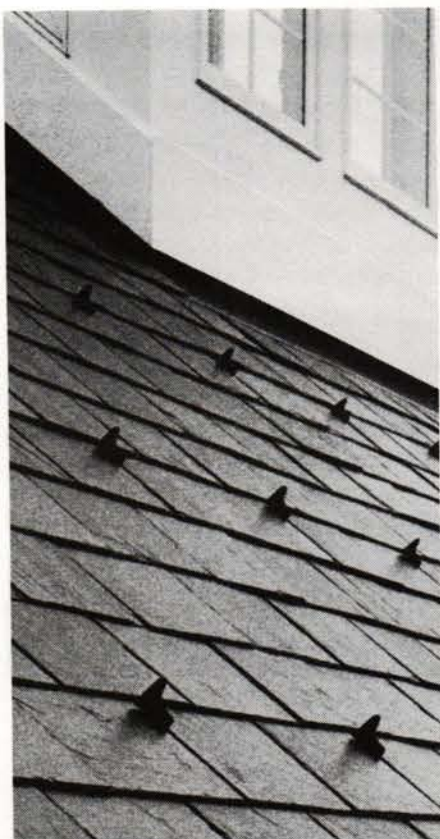
Cast bronze snow guards in a variety of patterns for slate, tile, and shingle roofs are the specialty of MULLANE SNOW GUARDS. Write in No. 56
