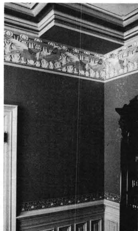
The decorative treatment for this room, part of the former Zen Center Guesthouse, includes a stencilled frieze of pheasants and irises (which required 16 overlays), floral wall powdering, and a stencilled chair rail band. ZAFFLE FINE DECORATIVE PAINTING. Write in No. 837
