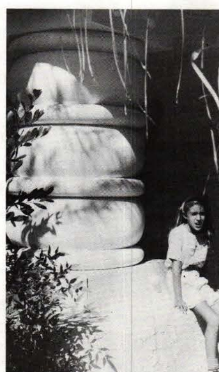
ABAROOT MFG. CO. produced this giant, turned-redwood post (5 ft. tall; 4 ft. in diameter), one of a pair located at the entrance to a Thousand Oaks, Calif. restaurant. Write in No. 805
