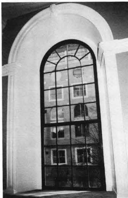
For historic Faneuil Hall in Boston, Mass., ALLIED WINDOW furnished to the National Park Service inside-mounting (Allied One-Lite, standard bronze, with U/V protective laminated glass) storm windows that perfectly match the glazing-bar pattern of the exterior historic wood sash. Write in No. 69
