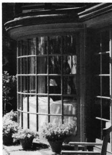
The manufacturing flexibility of ZELUCK DOORS & WINDOWS that enables it to engineer almost any shape window is demonstrated on this custom bow-front true-divided-lite residential window. Write in No. 692
