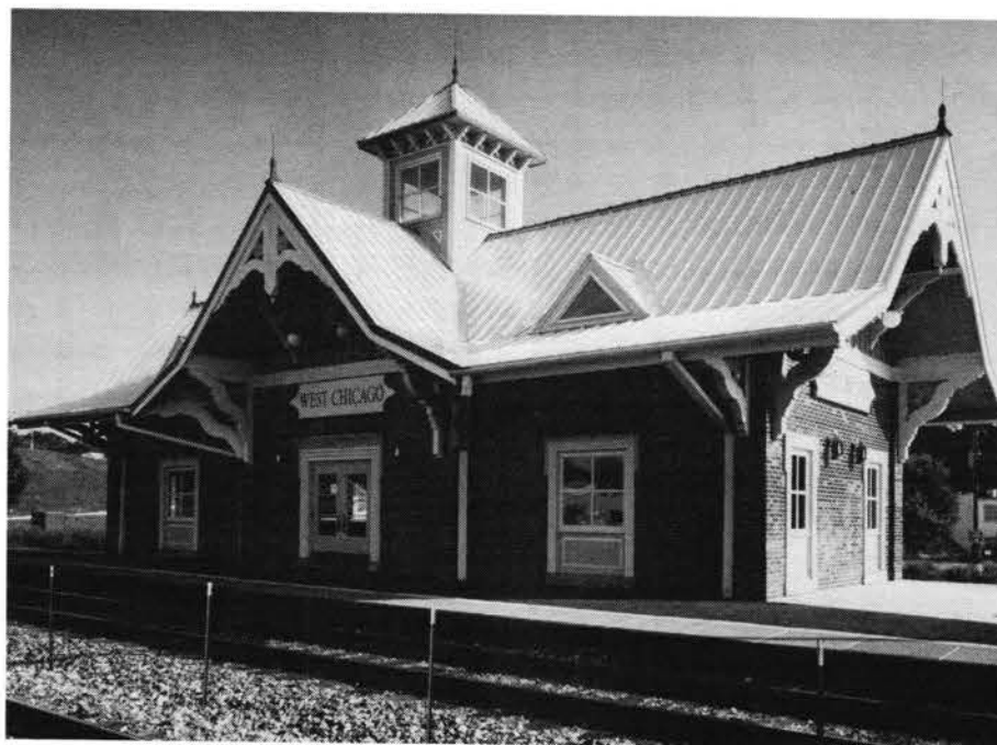
Snap-On standing-seam panels from PETERSEN ALUMINUM were used to re-roof this 19th-century railway station in West Chicago, IL. The Snap-On panels come in both aluminum and hot-dipped galvanized steel.
