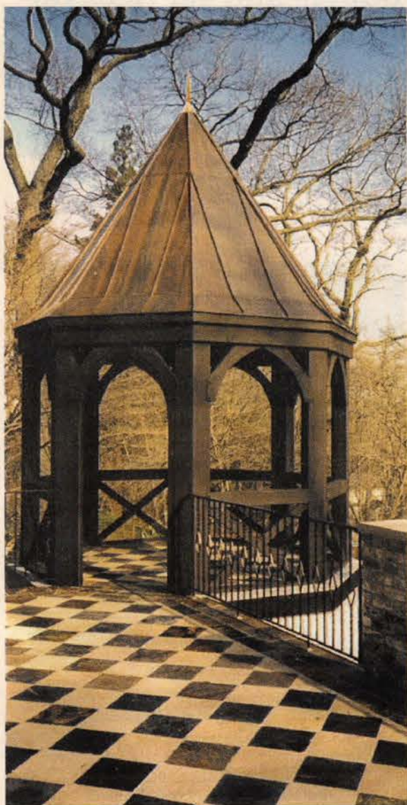
FSW designed an addition to a 1936 Norman-style residence, which included extensive stone terraces and this heavy-timber and copper gazebo. The terrace is surfaced in a checkerboard of cream and lavender Asian slate.
