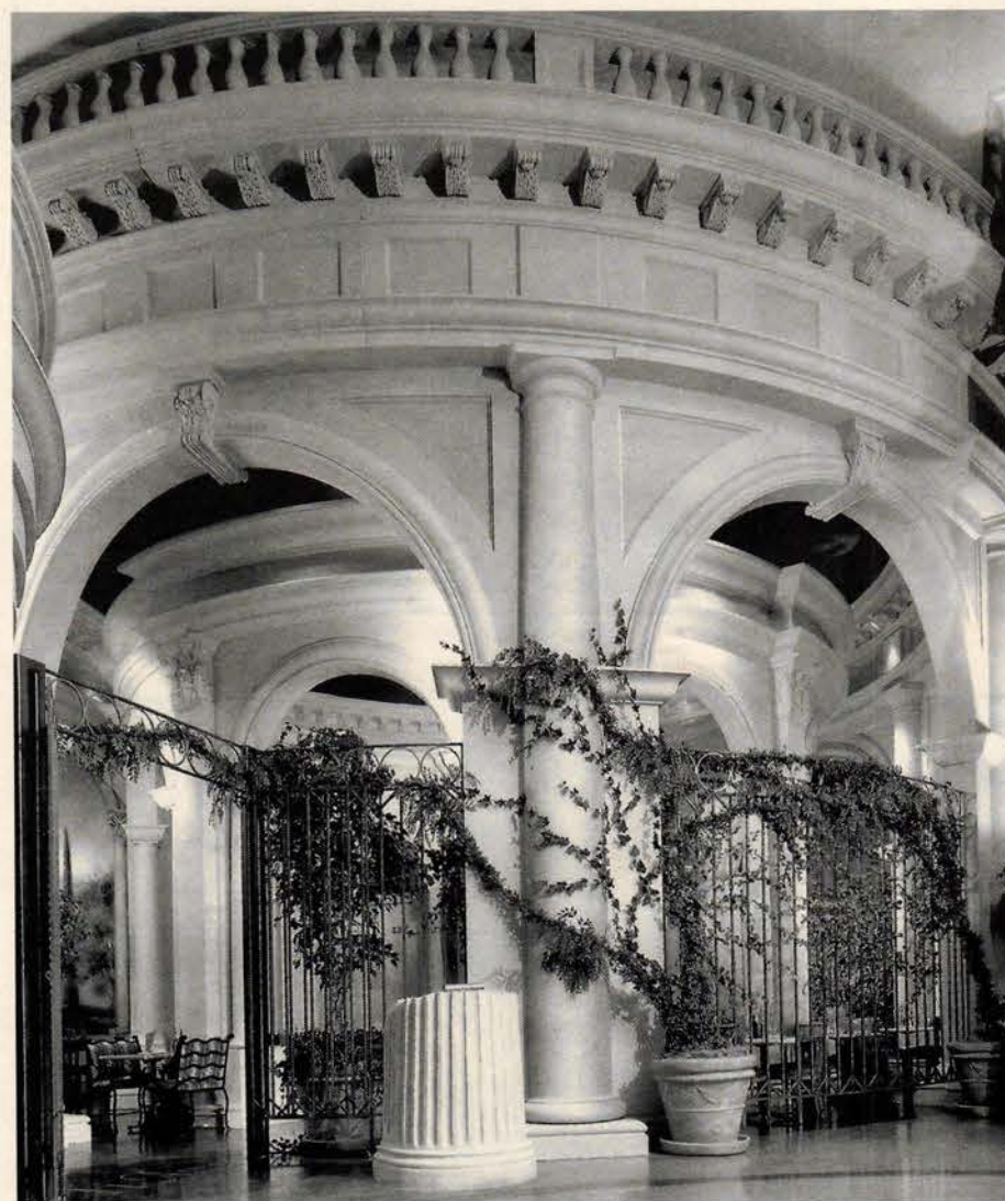
For the restaurant of the Santa Fe Casino, ARCHITECTURAL REPRODUCTIONS produced radiused colonnades with a textured, molded stone, using integral aggregates and pigments in a gypsum-based material. Write in No. 6130
