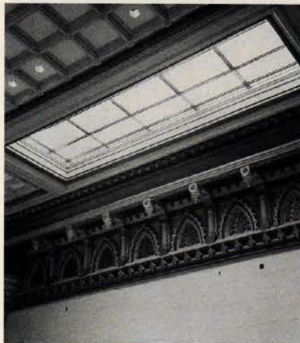
NIKO CONTRACTING repaired the elegant cornice in the lobby of the South Carolina State House (see Project Report on p. 90) and installed a new cornice and pressed-metal ceilings, along with a new bronze skylight, mullions, and trim.. Write in No. 8500
