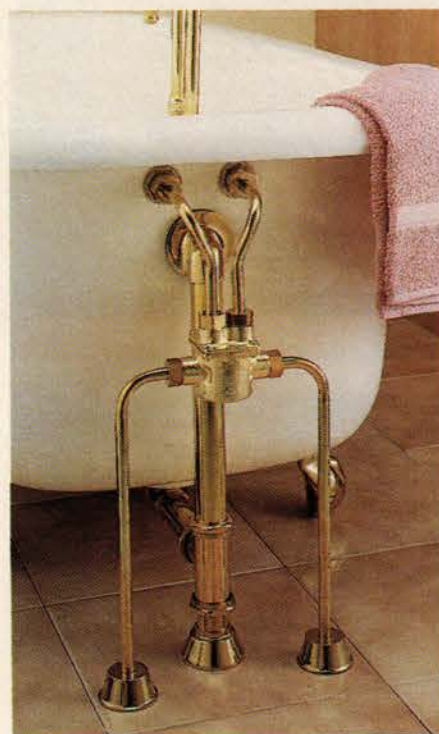
The pressure balance valve for clawfoot tubs from AFFORDABLE ANTIQUE BATH & MORE keeps bathers from getting scalded when someone flushes the toilet: The valve automatically reduces the hot-water flow to maintain the set temperature. Write in No. 817
