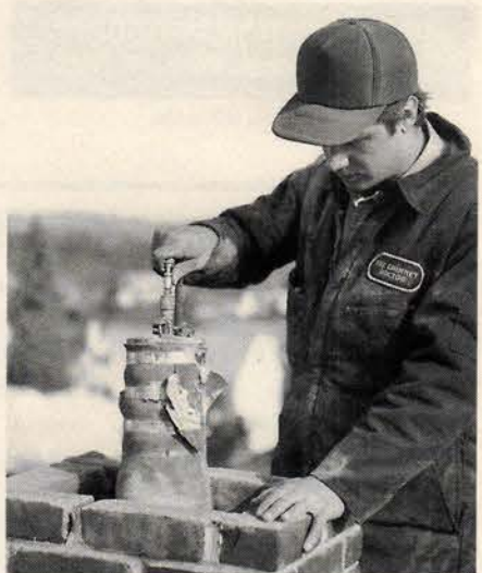
Working with the inflated flue-former, this worker from NORTH AMERICAN SUPAFLO is installing an efficient, safe chimney liner. Write in No. 5290
