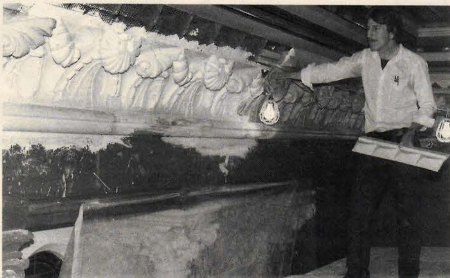
Restoration of the House of Representatives Chamber at the Connecticut State Capitol included SHELL BEACH STUDIO's plaster replacements for missing sections of the cornice.
