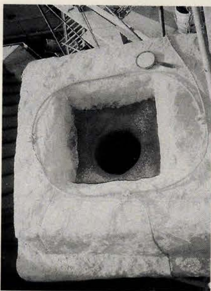
Here, the Cathedral of the Madeline in Salt Lake City, Utah, gets its AHRENS CHIMNEY TECHNIQUE "First Liner," a poured-in-place flue liner that will help strengthen and insulate the chimney. Write in No. 2440
