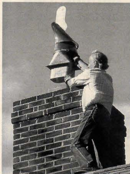
BELDES supplies an easy-to-install BELCAP Chimney Guard for woodburning fireplaces, which eliminates the infiltration of downdrafts, rain, and snow, and deflects the wind in different directions to improve the draft. Write in No. 822
