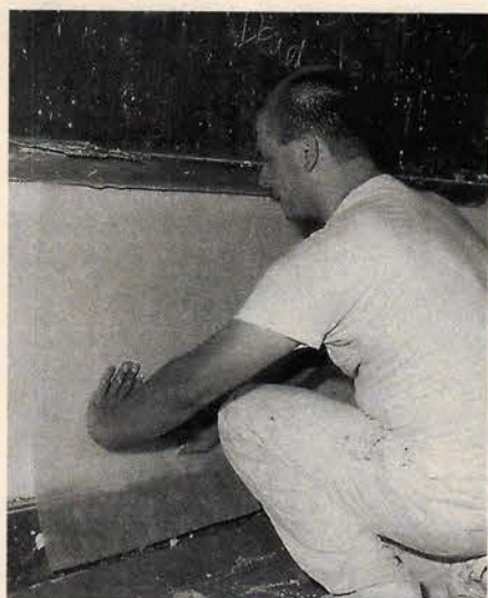
With the Nu-Wal system from SPECIFICATION CHEMICALS, a saturant is applied to the damaged wall surface and then a fiberglass mat covers the wet saturant, as shown here. Later, a second coat of saturant is used to cover the mat. Write in No. 1550
