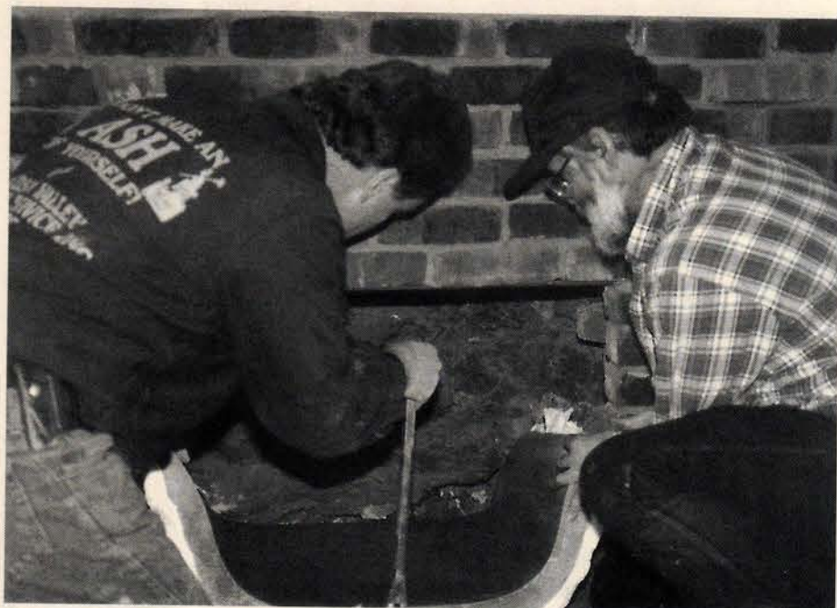
The apex-shaped component in a "Bellfire" system from SLEEPY HOLLOW CHIMNEY SUPPLY, LTD., creates a hot spot that radiates heat back into the room. This system can be retrofitted into an existing conventional fireplace. Write in No. 8500
