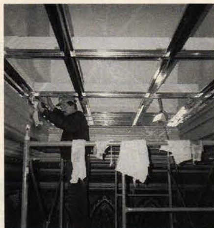
The gleaming bronze cornice, mullions, and trim in one of the State House skylights are adjusted by a NIKO worker.
