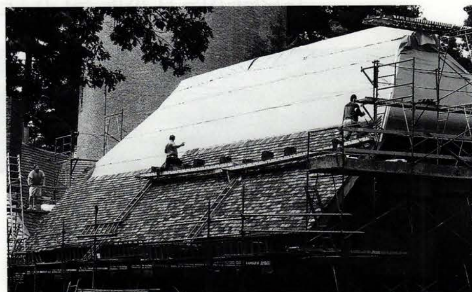
Daltex Roofshield, a breathable underlayment distributed by LINER ROLPANIT, is shown being used with clay roofing tile. Write in No. 5025
