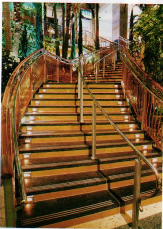
The success of the finishes brought Ritins to the Casino's steel stair railings. The finish specifications called for silver on brass paint. So Ritins mixed pewter flakes in an acrylic suspension that was brushed on. (Had the stair rail not been installed they might have sprayed the finish on.)
