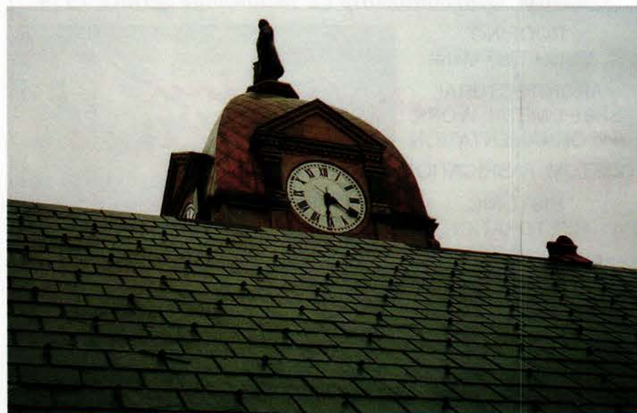
The dome on the clock tower of the Hancock County Courthouse in Findlay, Ohio, was sheathed in new copper by NIKO CONTRACTING, who also replaced the slate roof as part of a complete restoration. Write in No. 8500
