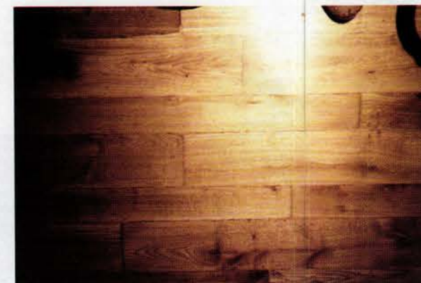
Christian Brothers' sister company, Olde Good Things Antique Wood Salvage, milled the wood into 4-, 6-, and 8-in. widths to replicate the pattern of the original floor. The fumed oak was finished with Christian Brothers' own polyurethane mixture.
