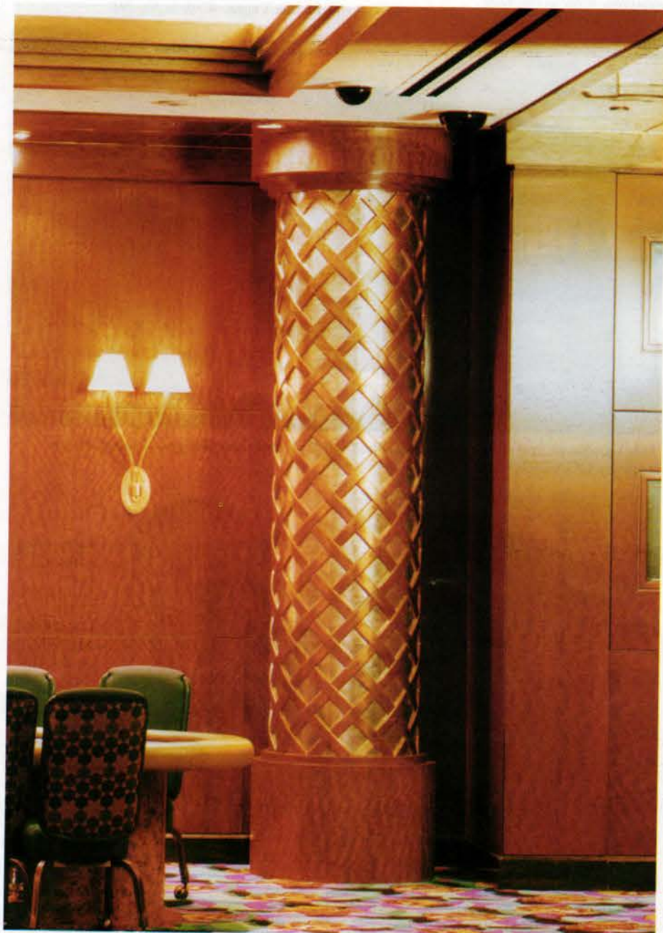
This GRG column was cast in halves (see top photo) and given a foil finish.
