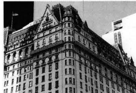
THR CAST STONE & GFRC replicated the terra-cotta ornament on the facade of New York City's Plaza Hotel using cast stone. Write in No. 545
