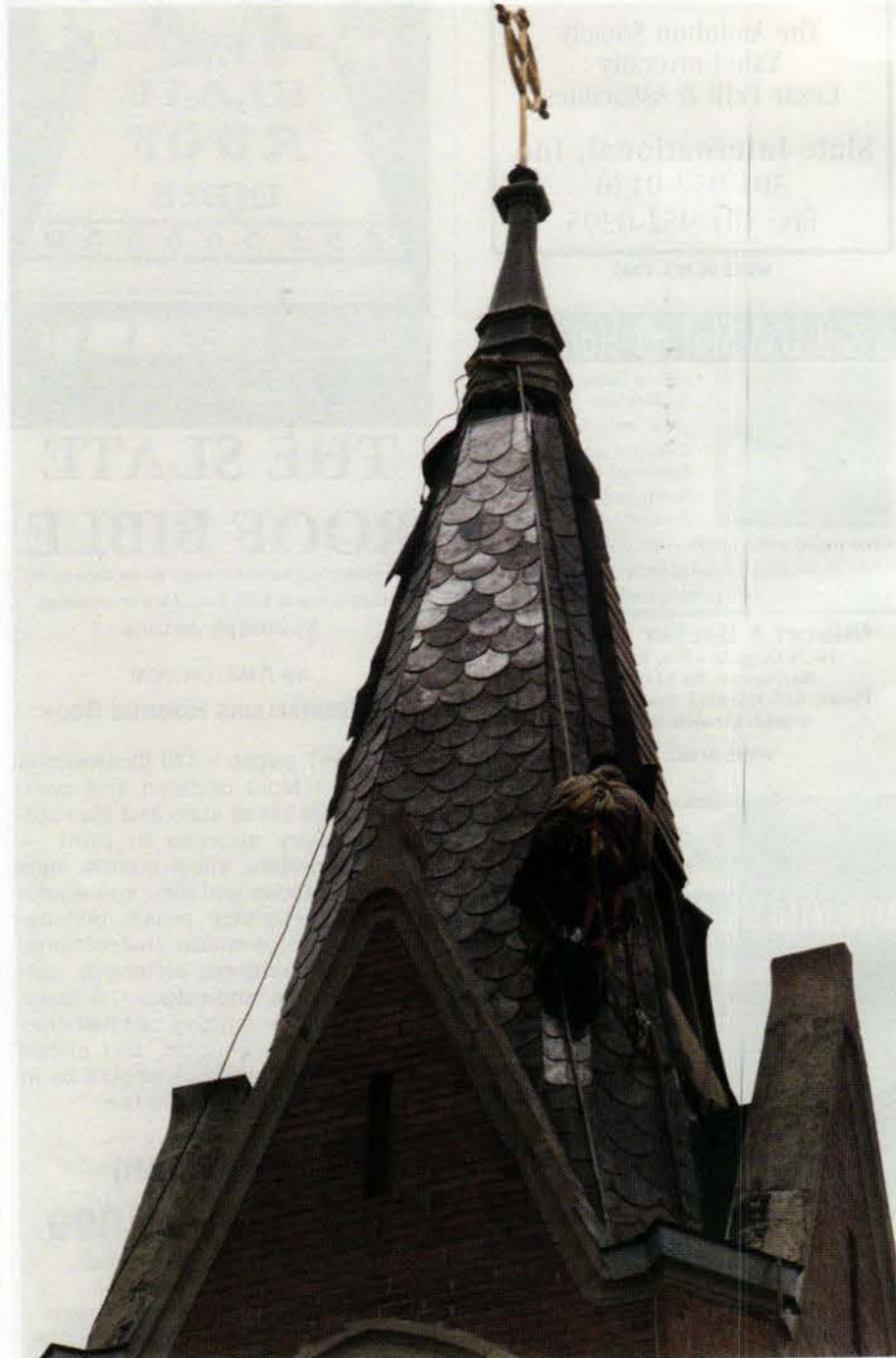
An installation specialist from L.W. Thomas Roofing Company hangs in a boatswain's chair while fastening lead shingles to the Church spire. Two copper nails were used for each shingle and approximately 3,000 shingles were installed.
