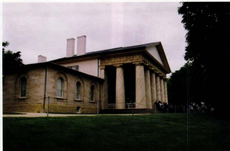
In this post-restoration photo of the facade and front portico, note the exuberant veining on the columns and the "over-the-top" quality the faux finish gives to the house. The base of the house has a pebble-dash finish resembling unpolished Sienna marble. The portico columns and facade are painted to resemble Aquia sandstone, an indigenous sandstone quarried at the Aquia Harbor near Washington, D.C. Aquia sandstone was commonly used during the 1800s on many federal buildings, including the White House. Not a particularly durable material, the sandstone was usually painted for stability. The restoration was based on archival photographs; paint analysis provided the colors and tones. (Photo: Shannon Cobalan)
