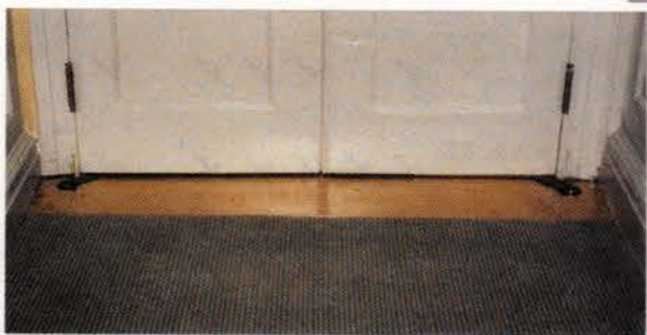
Besides concealing the operating mechanisms and all but an inch or two of the metal arms, the 12-in.-wide brass plate at the thresholds of the doors also matches the existing kickplates.
