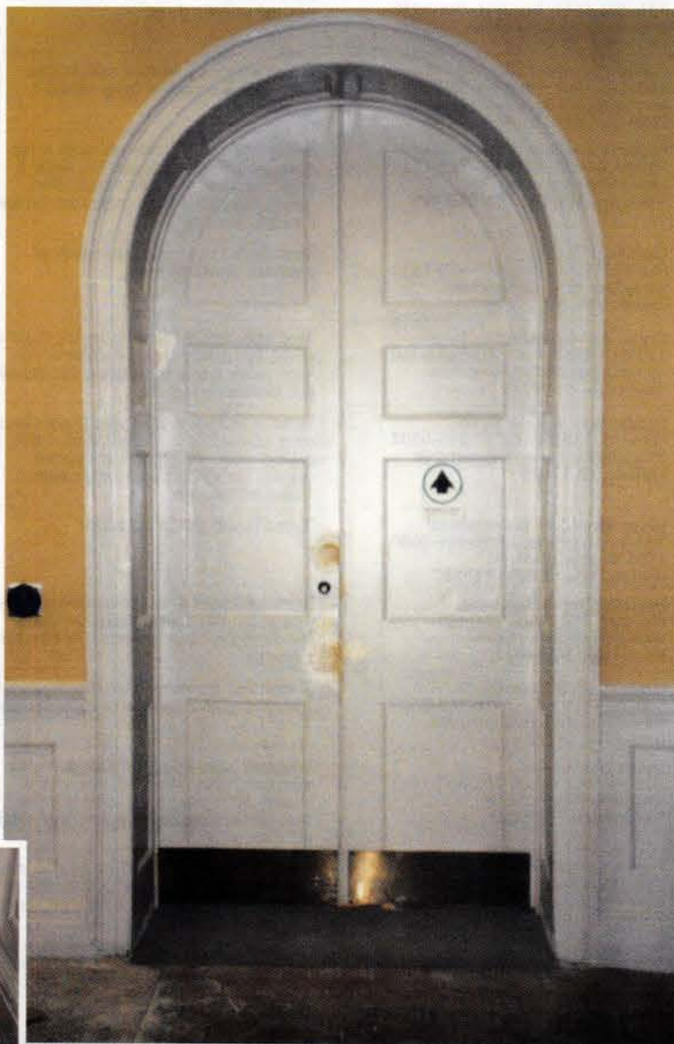
Besides concealing the operating mechanisms and all but an inch or two of the metal arms, the 12-in.-wide brass plate at the thresholds of the doors also matches the existing kickplates.
