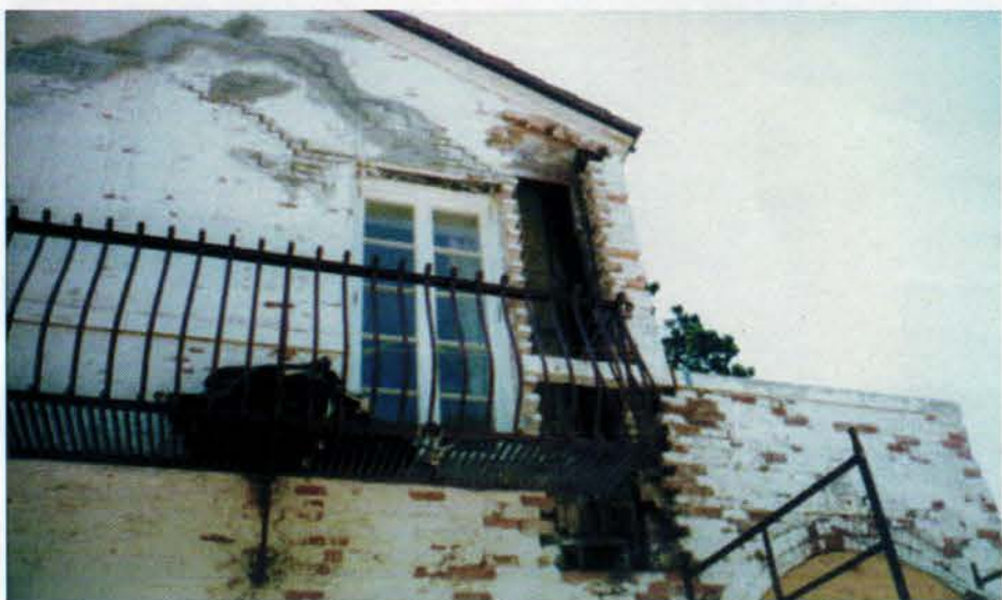
Before: These photos are examples of typical exterior conditions found on Crane Cottage at the outset of refurbishment. Warren Murphey of the JIA was very concerned about even touching the original brick. The building envelope was in extremely fragile condition due to the use of Georgia Brick, a very soft, porous material with a low iron content. Years of exposure and neglect led to cracking and severe water damage. Photos courtesy of Blanchard Caulking and Coating
