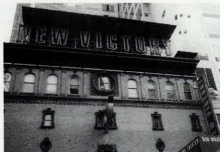
IDEAL ROOFING fabricated and installed a new copper cornice for New York City's New Victory Theater, replicating the design of the original.
