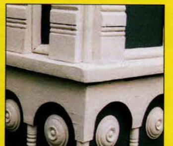
Antique window sash is salvaged, consolidated with LiquidWood & rebuilt with WoodEpoxy .
