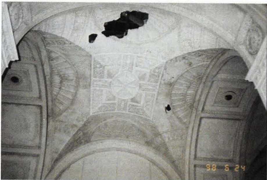
The extreme conditions that IFACS faced at the outset of the project included the Georgian Room/North Ballroom, where 80 percent of the plasterwork had to be re-created with careful casting and moulding. Here we see a detail of the damaged groin vault in the Georgian Room/North Ballroom prior to restoration.
