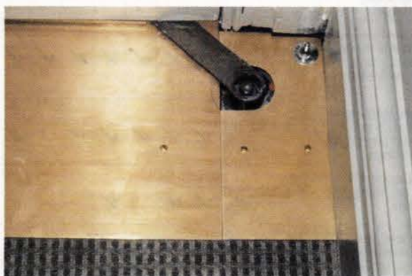
F.E. Ciccone's mechanisms for automating the internal doors in University Hall at Harvard University consist of an electro-hydraulic operator (top) and custom-fabricated metal arm (middle). The mechanisms were installed beneath the floor and covered with an 1/8-in.-thick brass plate (above).
