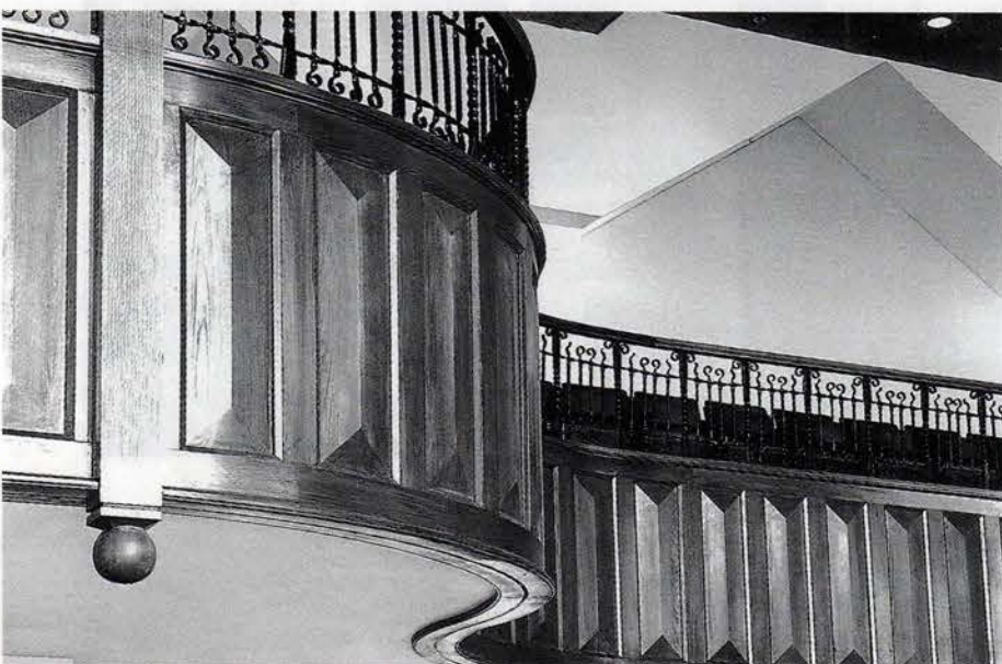
HULL HISTORICAL MILLWORK employed 60 ft. of longleaf yellow pine paneling, curved on both sides, to create this paneled balcony. Write in No. 5016
