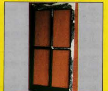
Antique window sash is salvaged, consolidated with LiquidWood & rebuilt with WoodEpoxy .
