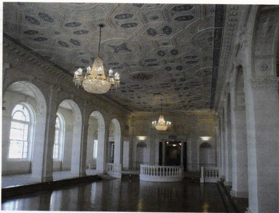
This image shows the Imperial Ballroom (South Ballroom) after completion. This room had less damage than the North Ballroom and was where International Fine Art Conservation Studios (IFACS) began their work. The procedure began with the plasterer who assessed the restoration and consolidated the 40 elements to be recast or replaced — more than a third of the plasterwork in this room is new. With the scaffolding in place and the delamination of previous coatings removed, the painters followed behind with a paint method devised to fast-track the job. First, a stain-resistant primer was applied, followed by two coats of semi-gloss base color. On top of that came a contrasting base color that was wiped off, leaving a trace for shadows and definition. (All interior photographs provided by Geoffrey Steward of IFACS.)
