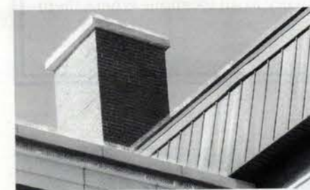
Stainless-steel strips from NIXALITE were used to render the roofline of the East Chicago City Hall uninhabitable for birds. Write in No. 570
