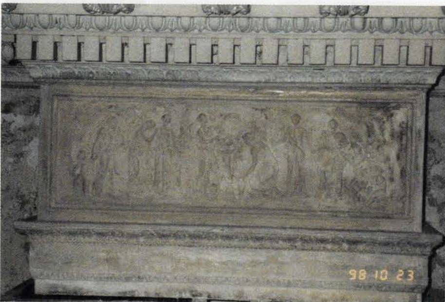
This detail in the Georgian Room/North Ballroom forms part of the frieze above the cornice and a column capital. The existing paint was removed to allow a mould to be taken. Many elements were reproduced in this fashion to replace portions that were missing or too severely damaged to be restored. The plaster restoration was carried out by a highly skilled team from WCC, Inc.
