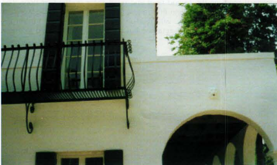
After: Dennis Blanchard of Blanchard Caulking & Coating in Jacksonville, Fla., provided his expertise for the tricky removal of all existing coatings and paints; brick repair and replacement; restoration of all wooden surfaces such as shutters and windows; and rehab for metal components such as hinges, shutter clips, and lintels. Window lites were reglazed and the roof soffit and rafter tails were scraped, puttied, sanded, and primed prior to the application of two finish coats. The ornamental metal handrails, balconies, and iron gates in the courtyard were also repaired and reattached as necessary. Blanchard Caulking and Coating were the recipients of the Associated Builders & Contractors Award for their contributions to the rehabilitation of the Crane and Cherokee cottages. Photos courtesy of Blanchard Caulking and Coating
