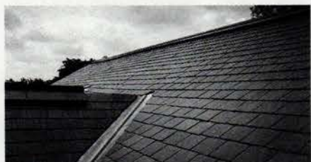
CASTLE METAL PRODUCTS' "Top-Slate" system of ridges, hips, and vents strengthens a slate roof's weakest areas and provides a permanent, watertight finishing course. Write in No. 2901
