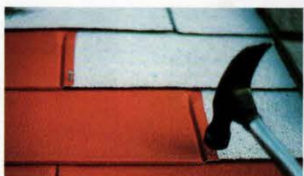
Lightweight, aluminum 3-Tab Covers from REINKE SHAKES can be installed on a roof with just a hammer or air stapler, a tin snips, and maybe a 1x2x10-in. block of wood. Write in No. 1546
