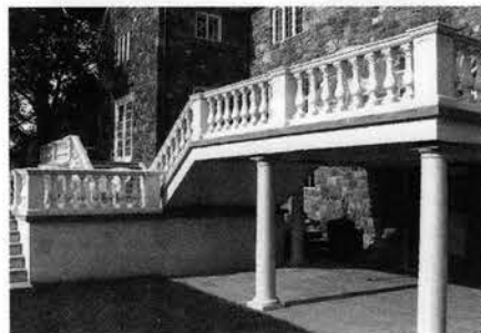
These balustrades, rails, and columns were made with "duoMatrix-C" polymer additive for concrete, using SMOOTH-ON's "Brush-On" 50 molds backed with "Plasti-Paste" support shells. Write in No. 650
