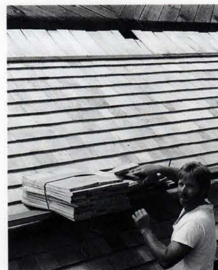
This worker is applying LIBERTY CEDAR's Alaska yellow cedar taper-sawn shakes with a cedar breather underlayment over solid-pineboard sheathing. Write in No. 6550
