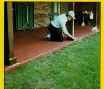
Rotted & infested base of a loadbearing column is completely sawed off & replaced with WoodEpoxy .
