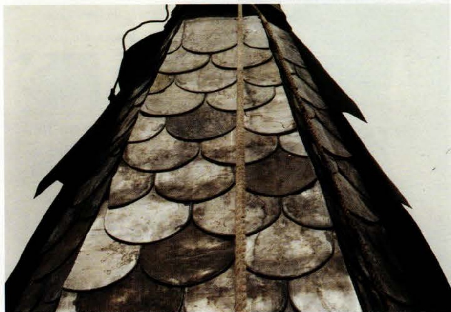
The lead shingles were fitted in the traditional plain-tile and slate technique, but are fixed directly to the substrate without batten. Because of lead's malleability, the shingles can be nailed to the substrate without any risk of cracking.
