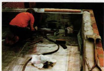
AMERICAN EAGLE ROOFING installed a new flat lead membrane roof on the First Presbyterian Church in Babylon, N.Y. Here, a lead burner seals a joint on a parapet capping. Write in No. 405
