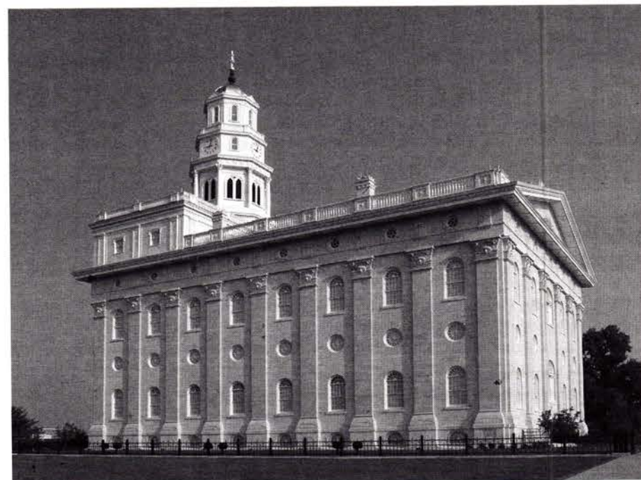
KEPCO+ installed the architectural stone-cladding system of Alabama limestone for the Nauvoo Temple in Nauvoo, IL. Write in No. 1492
