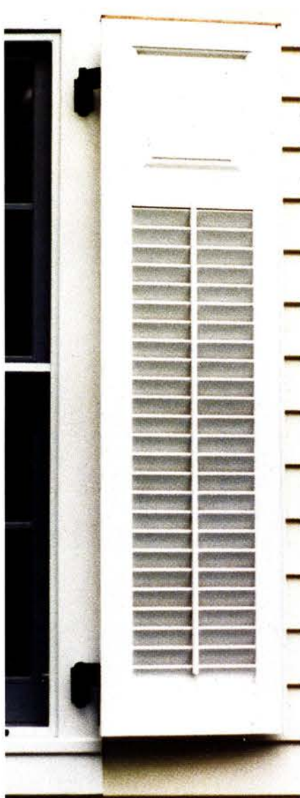
KINGSLAND CO. SHUTTERS fabricated this Honduras mahogany shutter using mortise-and-tenon joinery. Write in No. 196
