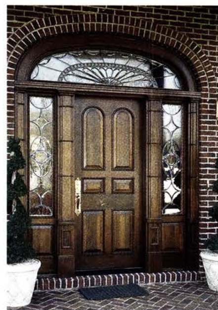
This solid mahogany door from JACK WALLIS STAINED GLASS & DOOR features leaded and beveled glass with interior-mount thermo-panels and a custom radius transom.
