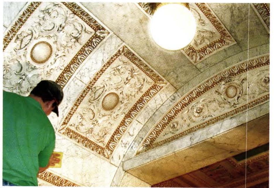
EVERGREENE PAINTING STUDIOS developed the methodology to clean tobacco-stained Italian marble in the three-story-tall double grand staircase of the Allen County Courthouse in Fort Wayne, IN. Write in No. 2460
