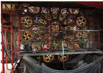
This 52-panel rose window, approximately 40 in. in dia., was fully restored by ATG STUDIO.
