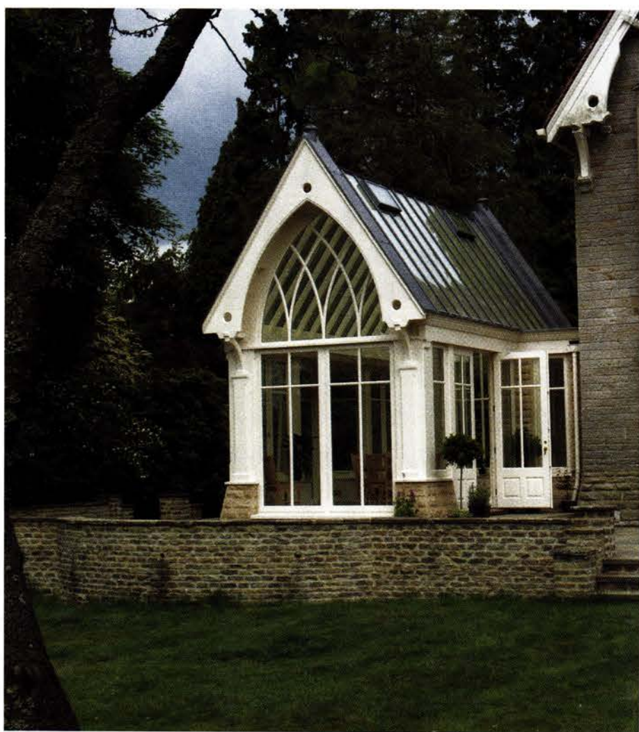
This design by OAK LEAF CONSERVATORIES complements the existing home with a steep-pitched gable roof featuring Gothic gable ends and matching bargeboards and brackets. Write in No. 6860
