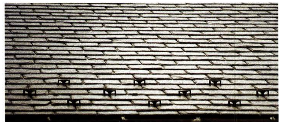
GOUGH SNOGUARDS & ACCESSORIES supplies snowguards made of heavy copper, seen here installed on a slate roof. Write in No. 2612
