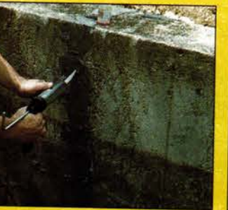
AboJet series for structural crack-injection
