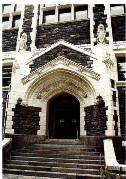
GLADDING, McBEAN, re-created the terra-cotta elements for the façade of Wingate Hall at the City College of New York. Write in No. 6010
