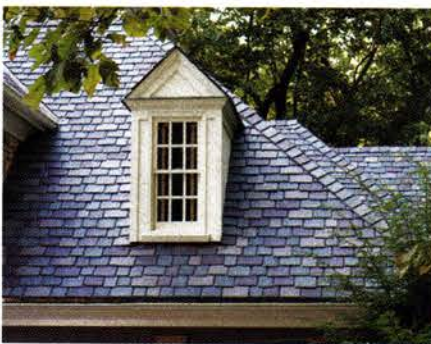
This roof from DAVINCI ROOFS-CAVES is made of factory-collated color blends that replicate the traditional multi-colored slate look.
