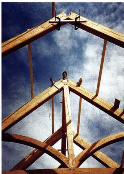
Glenn James of CRAFTWRIGHT is sitting on one of the 40-ft. trusses for the Saint Paul's Boy's School Chapel in Baltimore, MD, waiting for the next ridge piece. Write in No. 645
