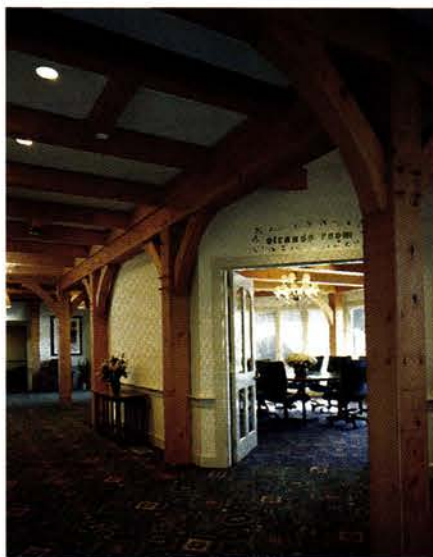
VERMONT TIMBER WORKS created a timber-frame addition and conference center for the von Trapp family lodge in Stowe, VT, using a Douglas fir octagon frame. Write in No. 927
