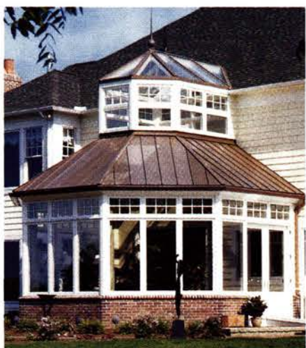
This two-story conservatory in Rochester, NY, built by RENAISSANCE CONSERVATORIES, incorporates a copper roof with a glass lantern. Write in No. 578
