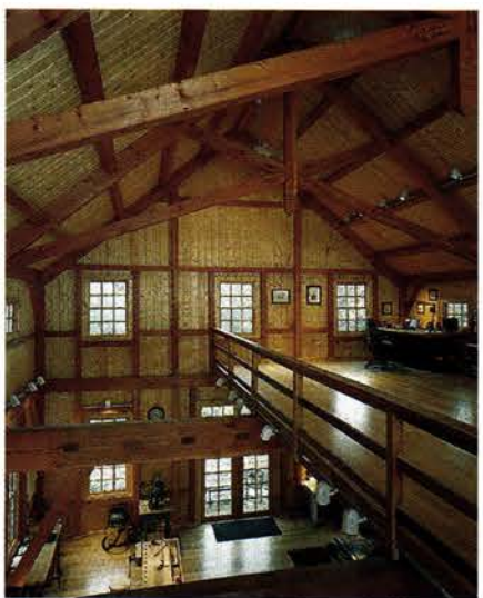
Dramatic scissor trusses that allow clear spans with no support posts were used by TIMBERPEG in the framing of this workroom. Write in No. 8570
