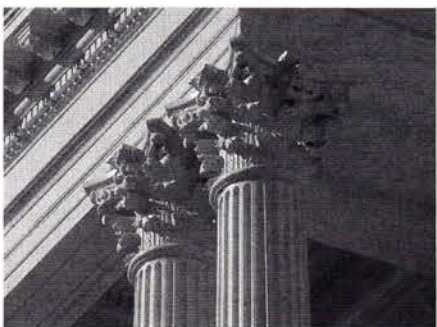
DEANGELIS IRON WORKS supplied and installed 12 2,200-lb. cast-iron capitals for the Massachusetts State House, which recently underwent an extensive exterior restoration. Write in No. 1025
