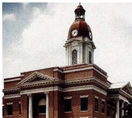
CAMPBELLSVILLE INDUSTRIES fabricated the 56½-ft. aluminum cupola with a 6-ft.-dia. clock and aluminum cornice for the Worth County Courthouse in Sylvester, GA. Write in No. 2750
