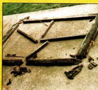
Antique window sash is salvaged, consolidated with LiquidWood & rebuilt with WoodEpoxy .
