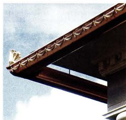
CLASSIC GUTTER SYSTEMS fashioned this elaborate half-round copper gutter with gold-patinated, solid-brass trim and a decorative rain deflector. Write in No. 1280
