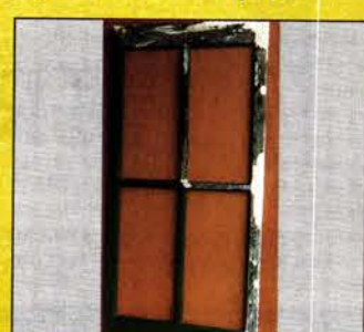
Antique window sash is salvaged, consolidated with LiquidWood & rebuilt with WoodEpoxy .
