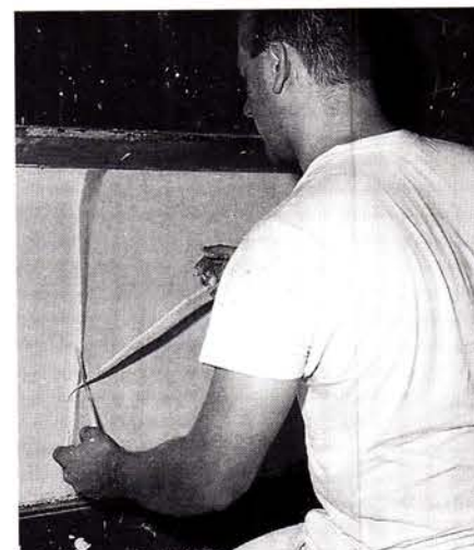
The Nu-Wall system from SPECIFICATION CHEMICALS is designed to restore cracked plaster walls and ceilings; the workman here is cutting and removing the overlapping strips before applying a second coat of saturant. Write in No. 1550
