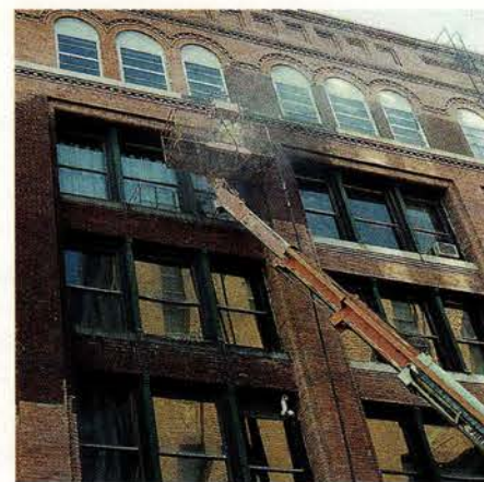
ArmaKleen supplies baking-soda-based cleaners that remove a variety of contaminants from brick, stone, wood, glass and metal.
