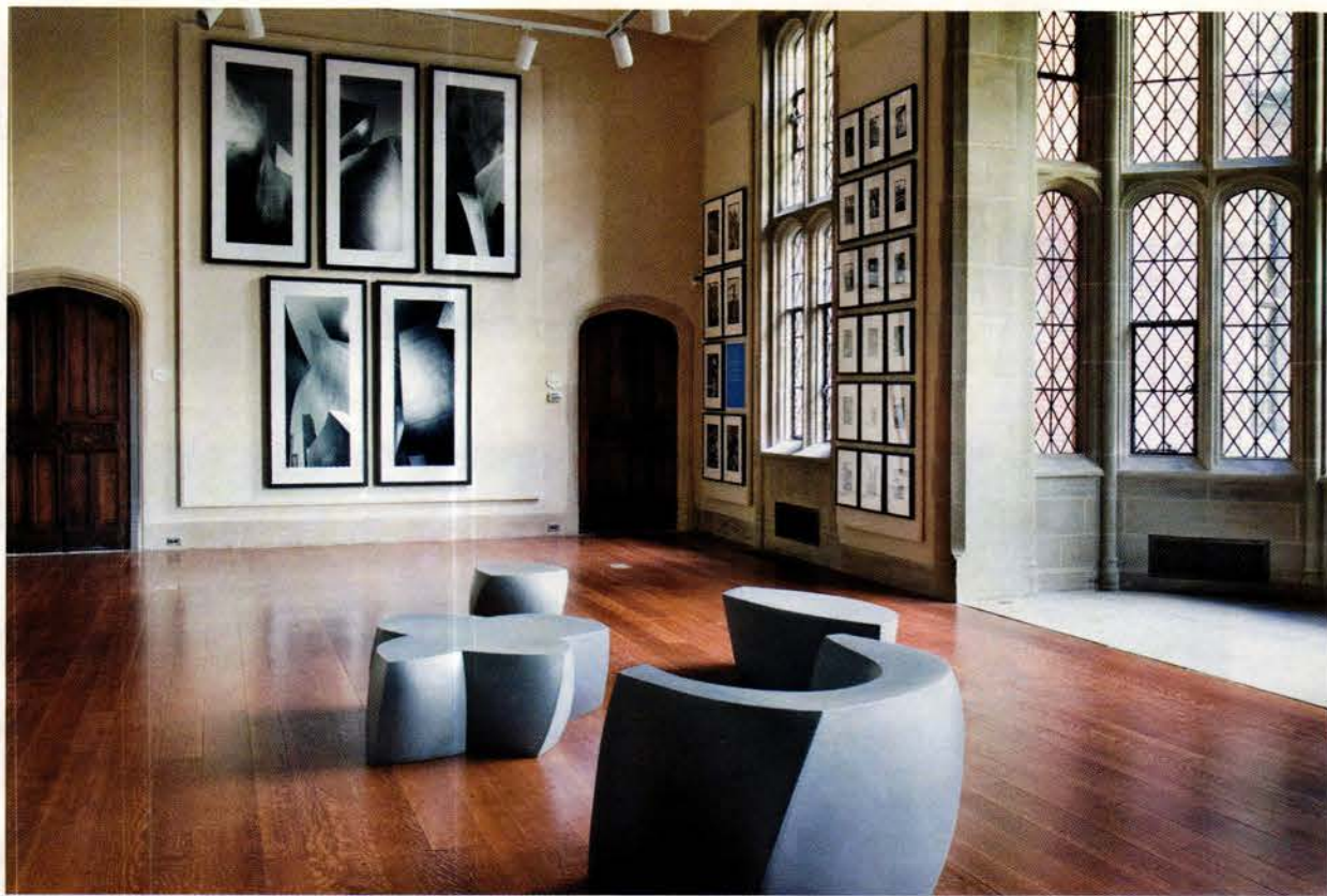
In front of one gallery's stone bay window (right) new vintage-looking sandstone flooring was installed. Original hardwood flooring was recycled to patch missing sections elsewhere in the 28,000-sq.ft. house.
