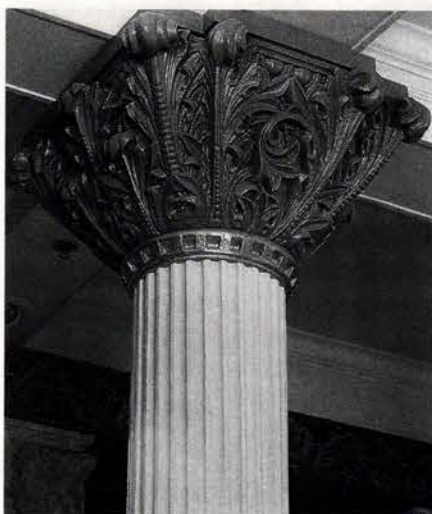
Architectural Reproductions used rubber molds to form this GFRC reproduction of an original cast-iron column capital and fluted shaft.
