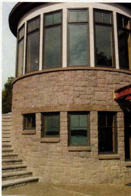
Dakota Granite's custom split-face ashlar, which has smooth top, bottom and ends, was used in the construction of this building.
