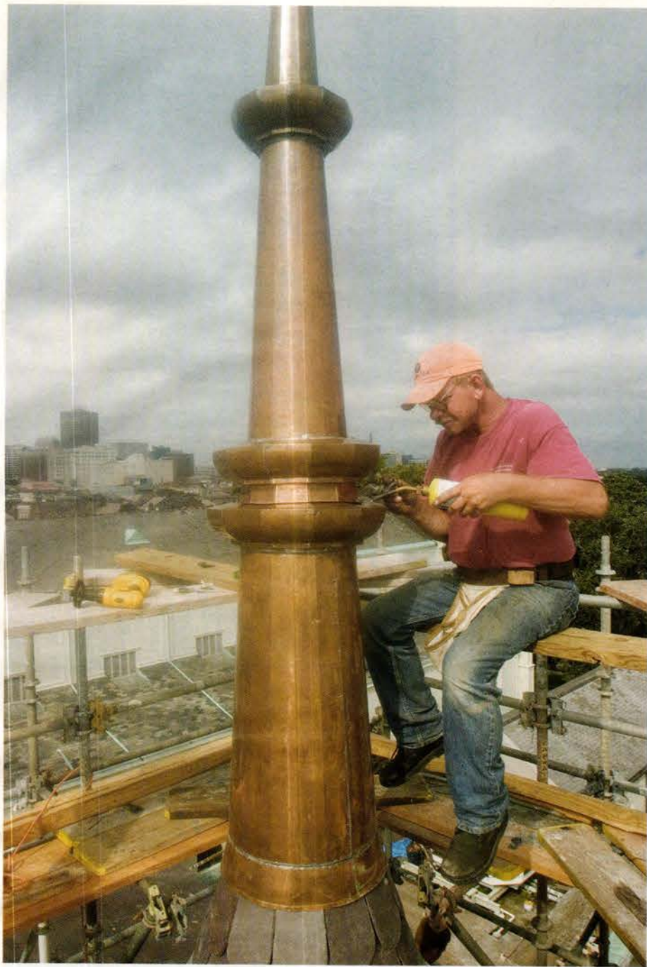
A brave metalsmith soldered the copper finial on top of the Presbytere's new cupola, the day before Katrina arrived. Built 1797-1813, the building, now a museum, had been without a cupola since it was toppled by a category 4 hurricane on September 29, 1915. This time, it survived the storm.
