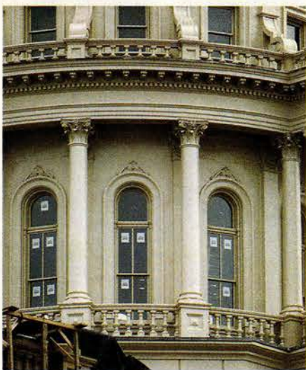
Adams Architectural custom manufactured these mahogany windows with insulated glass.
