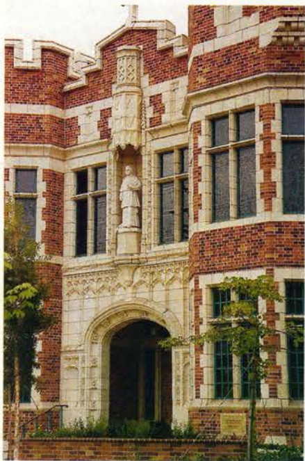
A&M Victorian cast new concrete ornamentation for the renovation of the Loretto-Conaty High School in Los Angeles, CA.
