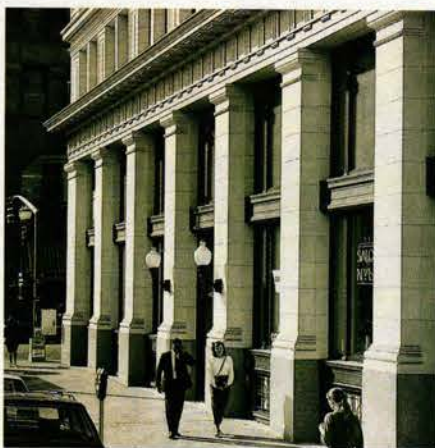
The original limestone columns of this 1919 building were replicated in GFRC by Architectural Reproductions.
