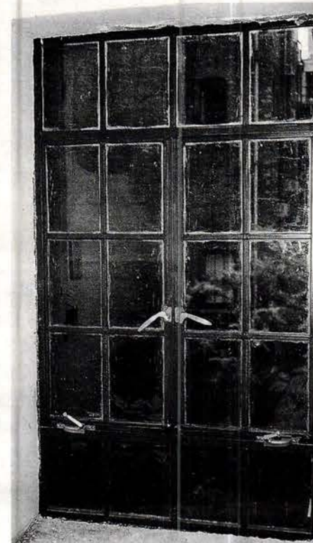
This vintage 1930s steel casement window was restored and installed by Seekircher.
