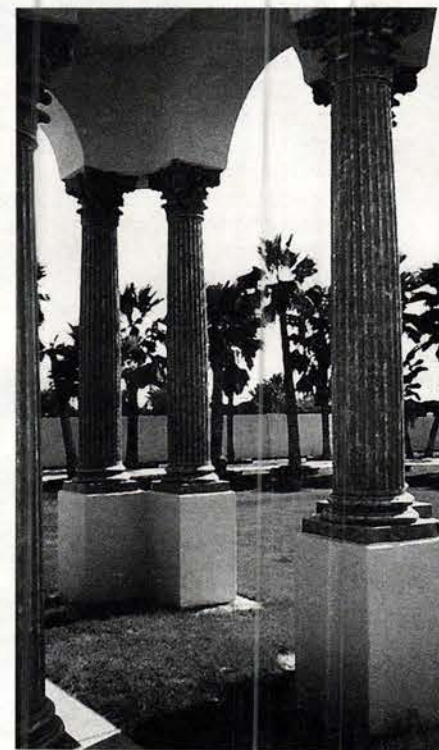
These 10-ft. fluted Corinthian columns with faux finishes were fabricated by Aristone.
