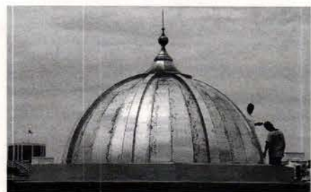
This 16-ft. copper dome and finial were designed and fabricated by C&J Metal for a building in Newport Beach, CA.
