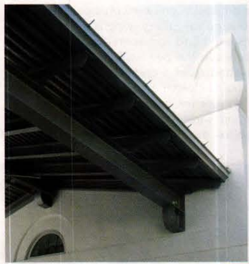
Above: The gallery wing is separated from the octagon by a delicately-scaled, gable-roofed breezeway, in which the steel roof structure is exposed to exterior view. The overhanging webs of the wide-flange steel rafters are shaped to resemble timber rafter tails. Photo: Steven W. Semes
