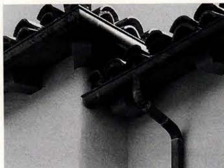
C&J Metal fabricated this 3-in.-dia. downspout and 5-in.-wide half-round gutter with radius surface in 16-oz. copper.
