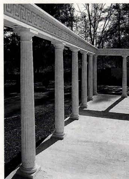
Manor Style's load-bearing, fluted fiberglass-composite columns and custom-fabricated PVC Greek Key-patterned beam adorn this patio.
