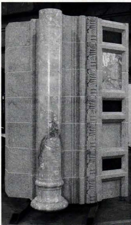
KEPCO+ attached three types of marble and Englishman Bay gray granite to a galvanized-steel frame to create this detail.
