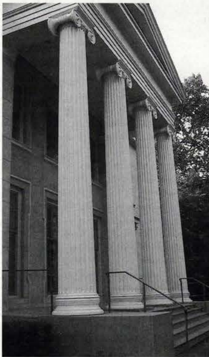
Fagan Design replicated this 30-in.-dia. x 20-ft.-tall fluted column (foreground) to match the existing columns.
