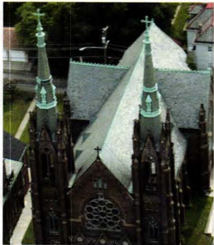
The Durable Slate Co. repaired the slate roof and replaced copper valleys, the ridge roll and the copper work at the base of the steeples of this century-old church and rectory in Ohio.
