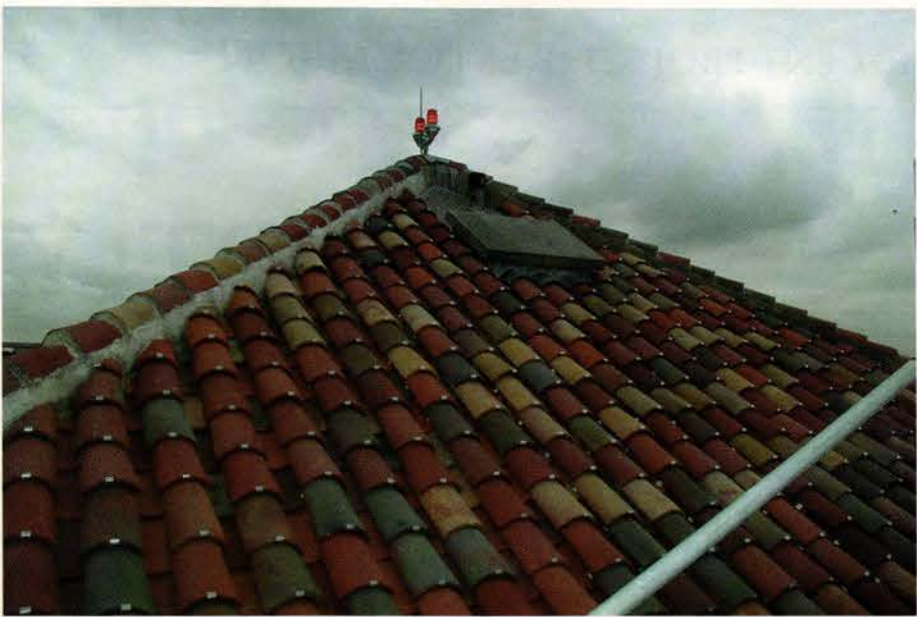
The stainless-steel hold-down clips are faintly visible here, but are rapidly acquiring patination. Photo: Walter B. Melvin Architects
