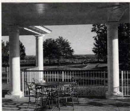
HB&G provided these low-maintenance load-bearing porch columns.
