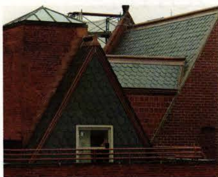
Nicholson & Galloway restored the roof of this historic building, providing the carpentry, coppersmithing, slate, waterproofing and masonry restoration.
