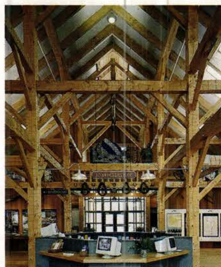
The Southeastern Vermont Welcome Center features a 48x96-ft. timber frame constructed by Vermont Timber Works.
