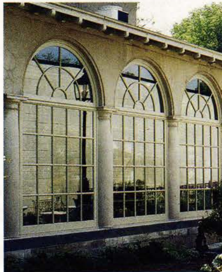
Grabill manufactured these fixed, round-top pine windows for a restoration project.
