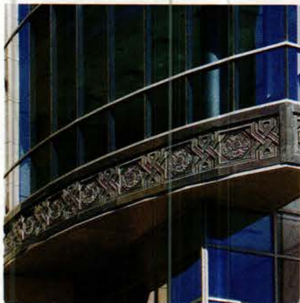
Steptoe & Wife created these stamped-bronze panels to mirror the existing stone frieze of a courthouse in Hamilton, Ontario.
