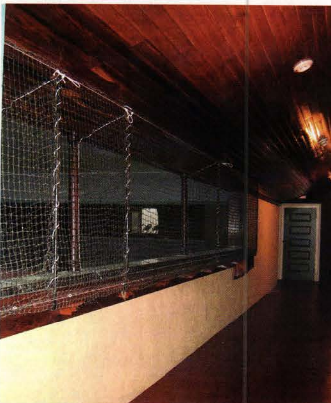
The corridors' tongue-and-groove ceilings have been brought back to their original high-gloss varnish. Sound insulation has been installed above them, where the original builders had stuffed bagfuls of sawdust.
