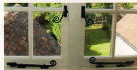
The design of this malleable-iron window hardware, hand cast by Kirkpatrick, was based on patterns that date back to 1855.
