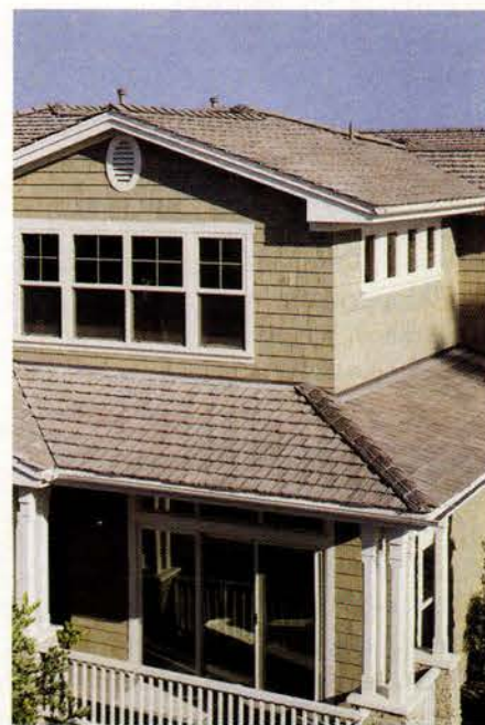
This concrete wood-shake replica from MonierLifetile utilizes random treatment of texture, edges and color for its realistic effect.
