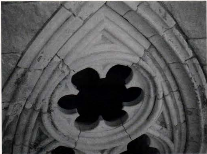
A 13th-century French limestone window had been misguidedly covered with aluminum and glass in the 1960s. A newly carved limestone hexafoil is shown here before it underwent slight distressing to induce patina. Inside will hang the museum's only rotating displays of stained glass. Photo: Walter B. Melvin Architects
