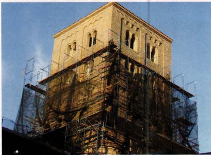
The Metropolitan Museum of Art has kept most of The Cloisters' galleries open throughout the six-year overhaul. Scaffolding has been enclosed and insulated, to minimize dust dispersion and draped on steel frameworks to avoid overloading roofs. Photo: Bernstein Photography
