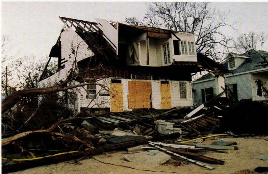
Top left: Volunteers disassembled and documented the Hecker House in Bay St. Louis, MS, salvaging the historic components so it might be reconstructed. They were also able to date the house to the late 1780s-1800, based on the internal structure that was exposed. Photo: World Monuments Fund
