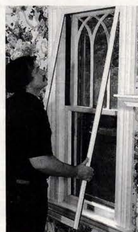
Vinyl-framed interior glass storm windows from Innerglass are designed to be mounted on the inside of the stops of the primary window.
