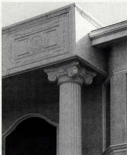
Ball Consulting's Forton MG was used for casting these quoins and columns.
