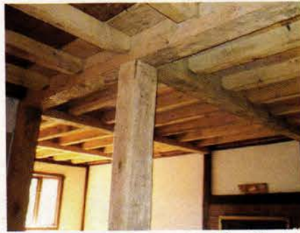
These 8x8 timbers were replaced by Colonial Restorations, under an existing chimney that had four fireplaces and a beehive oven.
