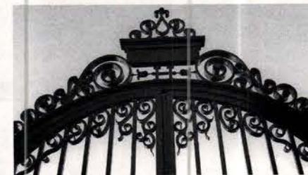
DeAngelis Iron Work fabricated this ornamental metal gate with hand-forged scrolls for a project at Harvard Yard in Cambridge, MA.
