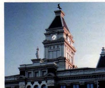
Campbellsville Industries fabricated the clock tower, clock, decorative cornice, modillions, paneled railing and corner pediments for the restoration project at Montgomery County Courthouse, Clarksville, TN.
