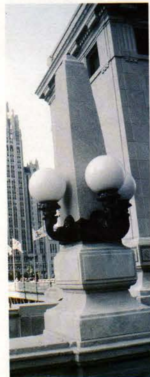
Allen Architectural Metals was commissioned by the City of Chicago to recreate a number of these bronze obelisk light fixtures from original castings.
