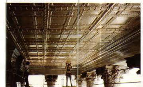
NIKO Contracting replicated and installed the pressed-metal ceiling panels and cornice for the South Carolina State House in Columbia, SC.
