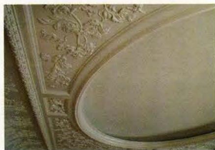
This ornamental plaster ceiling, fabricated by Foster Reeve & Associates, features custom hand-carved sculpture and elliptical trim.
