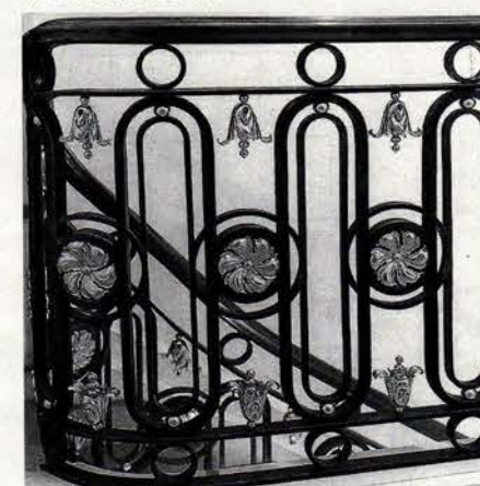
This stair balustrade with gilded repousse leaf work and custom bronze cap was created by Schwartz's Forge & Metalworks.
