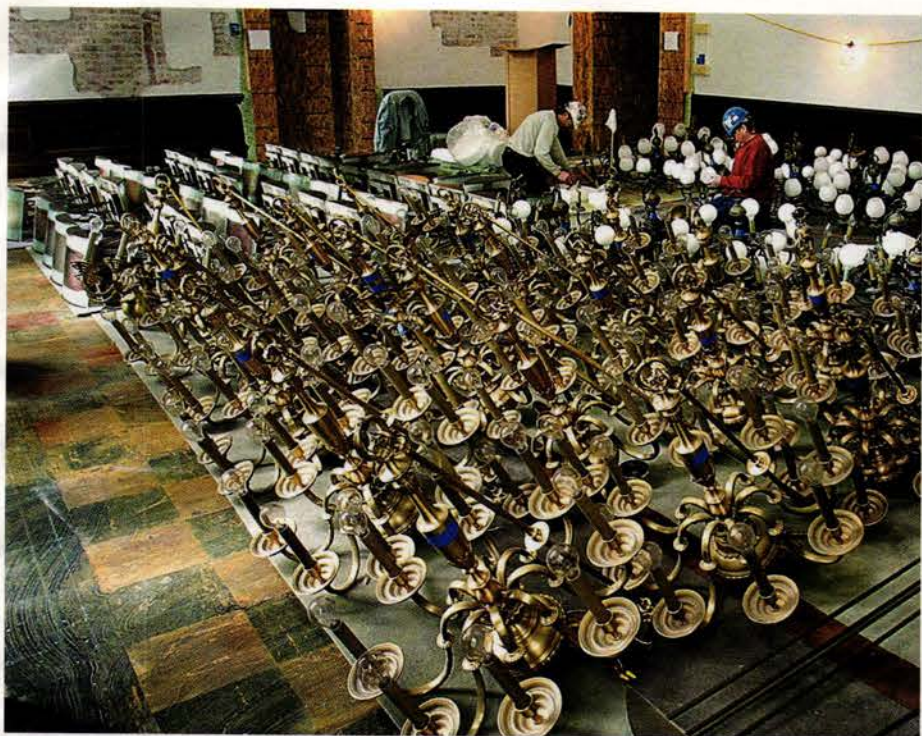
Light fixtures throughout the building were restored and retrofitted with fluorescent bulbs that use 75% less energy than traditional bulbs, saving as much as 73,000 kilowatt hours a year. Where new fixtures were needed, they were salvaged from other buildings or were made to match. Photo: Dick Milligan
