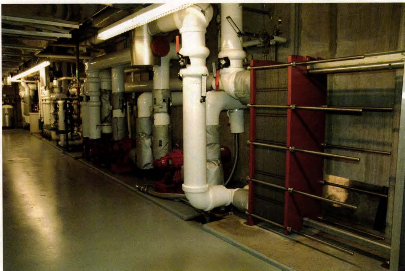
Approximately 400 to 500 gallons of water will move through the geothermal exchange plates supply and recharge system at K.C. Irving Environmental Science Center to cool the building on a typical hot summer day. Photo: courtesy of the K.C. Irving Environmental Science Centre
