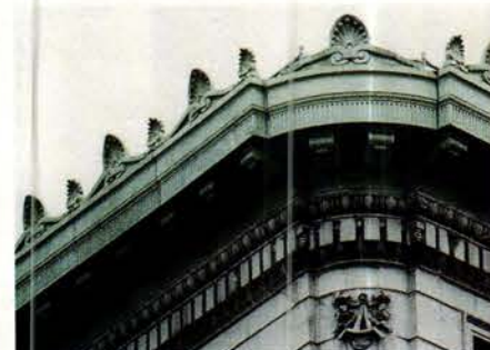
Towne House Restoration replaced the terra-cotta elements on this building with new elements made of cast stone and fiberglass-reinforced concrete.
