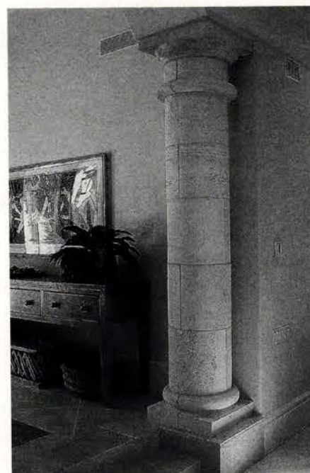
This 8½-ft.-tall Mexican travertine column was manufactured by Cantera Especial.
