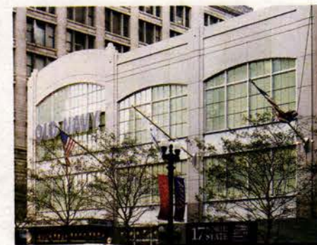
The glass fiber reinforced concrete (GFRC) used to re-clad this building on State Street, in Chicago, IL, was acquired from Ball Consulting.
