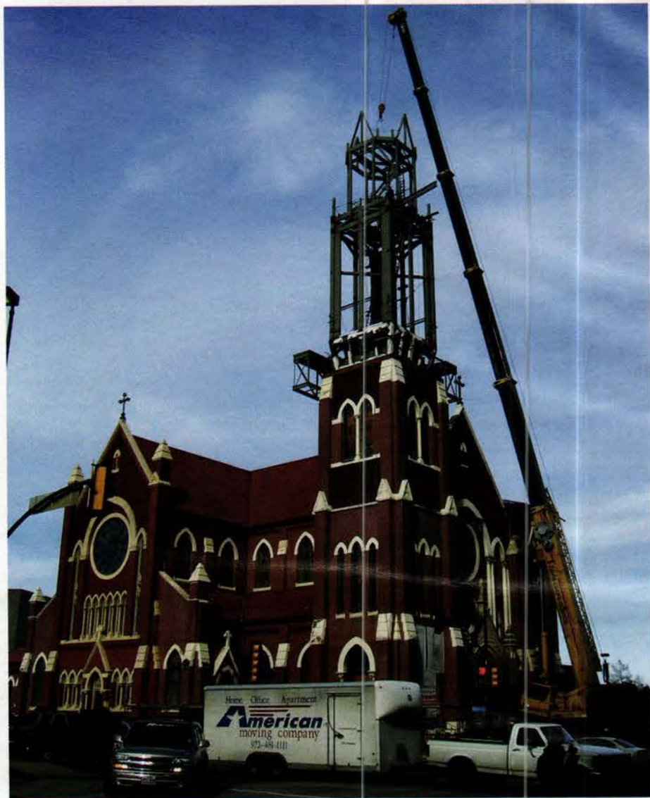
The steel frame for the tower was inserted into the original historic walls, piece by piece. The fourth section reached above the original walls of the historic tower base. Photo: courtesy of Architexas
