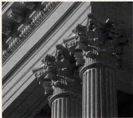
DeAngelis Iron Work supplied and installed 12 cast-iron capitals for the recently completed exterior restoration of the Massachusetts State House.
