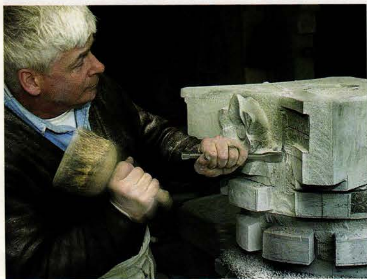
Keith Phillips of the Tenino Quarry carved decorative elements to replace those that had been damaged by the earthquake. Photo: Dick Milligan
