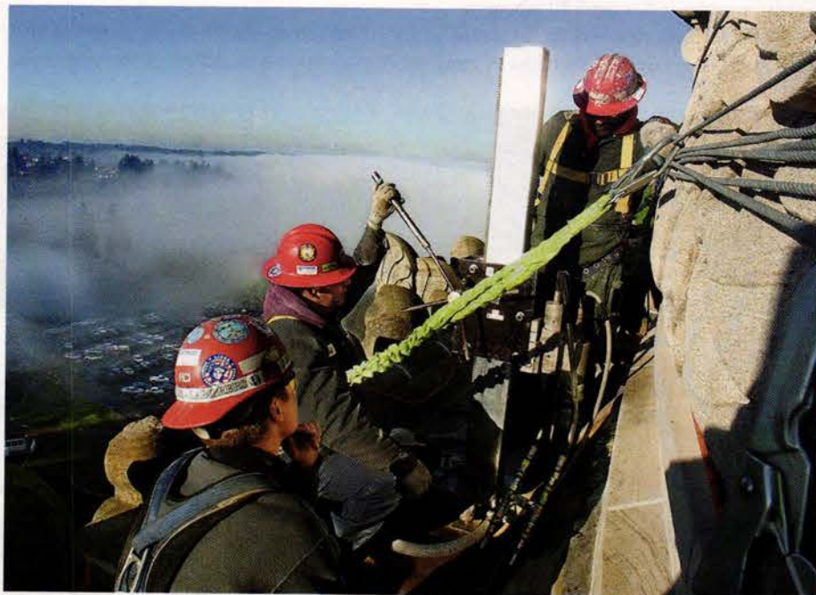
Workmen got a good view from the side of the building as they drilled from the gutter of the dome down through the center of each column to the colonnade base. Steel rods were then inserted into these holes and concrete was pumped into them to tie the dome, columns and base together. Photo: Dick Milligan
