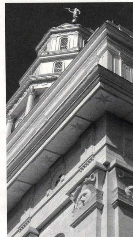
Traditional Cut Stone did the stonework for the Nauvoo Temple in Nauvoo, IL, including the pilasters and capitals.
