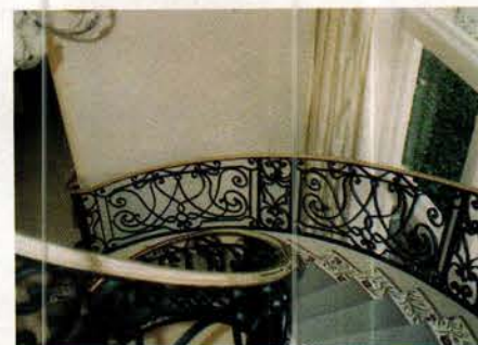
This forged-iron railing and polished bronze cap rail was designed, fabricated, finished and installed by Wiemann Ironworks.
