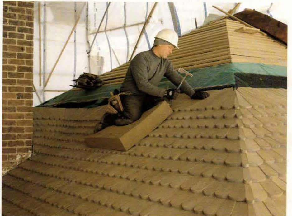
Old-growth cypress shingles were laid over new spaced battens to restore Montpelier's roof surface. The green membrane is Roof Shield, and the black mesh just above the shingles is Cedar Breather. A swept valley is visible behind the chimney at left, and a fanned hip appears on the right. The carpenter's foam rubber cushion protects shingles during installation.
