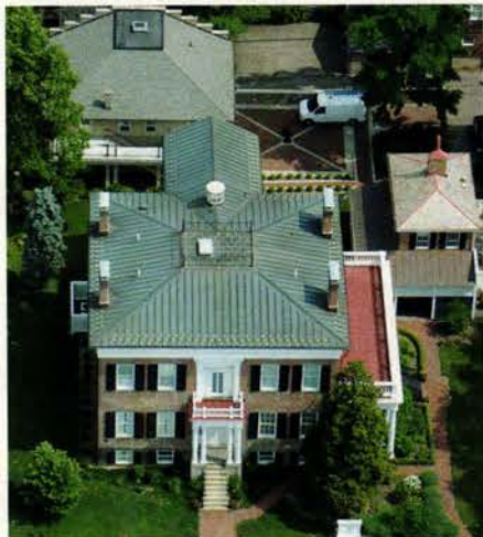
The Durable Slate Company restored this pre-Civil War-era mansion, now the Decorative Arts Center of Ohio, including the standing-seam and hand-soldered flat-seam copper roof on the main building and the slate roof on the carriage house.
