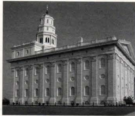
Kepeco+ installed the architectural stone-cladding system of Alabama limestone for the Nauvoo Temple in Nauvoo, IL.
