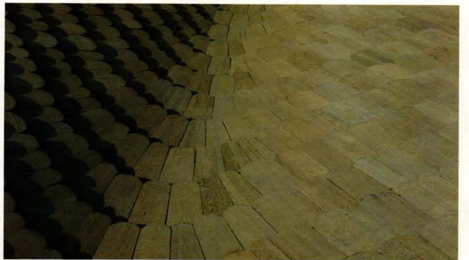
Old-growth cypress shingles were used to restore Montpelier's roof surface. The valleys were "swept," a period treatment that creates a seamless transition between adjoining roof planes. A hidden leaf of stainless-steel flashing is woven into each course at the valley. Photo: Maggie Wilson
