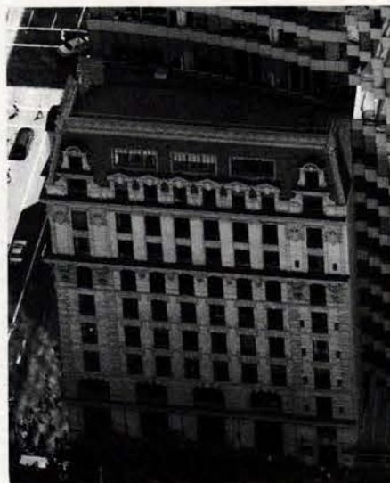
Nicholson & Galloway restored the slate roof, copper cornice and brick and limestone façades of this building.
