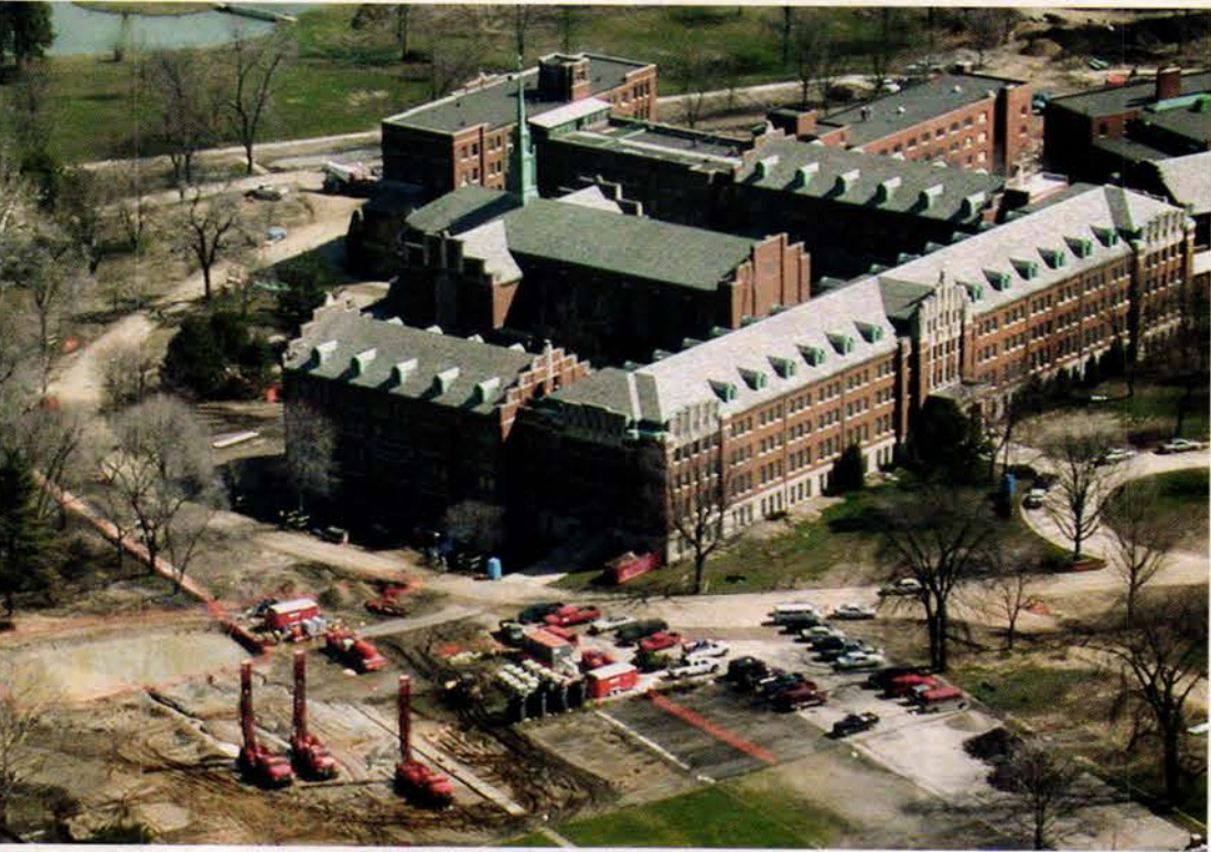
Above: The grounds at the Motherhouse of the Sisters, Servants of the Immaculate Heart of Mary in Monroe, MI, were torn up for several months during the installation of the large closed-loop geothermal system. It incorporates 232 boreholes, each 450-ft. deep, connected by 47 miles of pipe. Photo: Denyse Burkhart
