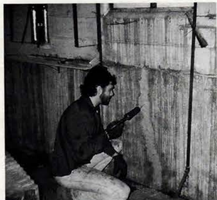
Cracked concrete structural elements can be restored with the Abojet crack-injection system from Abatron.
