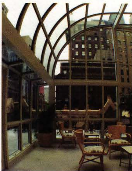
Glass House custom designed this conservatory, featuring custom bent glass and aluminum framing, for an upscale lounge in New York City.
