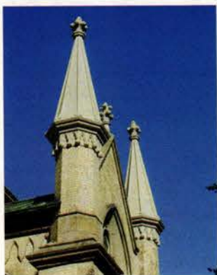
Traditional Cut Stone replaced the pinnacles on St. James Cathedral in Toronto.
