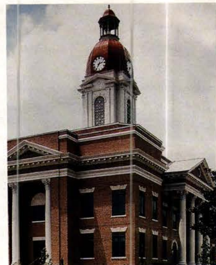
This 56-ft. 4-in. aluminum cupola, with a 6-ft.-dia. clock and aluminum cornice, was created for the Worth County Courthouse in Sylvester, GA, by Campbellsville Industries.
