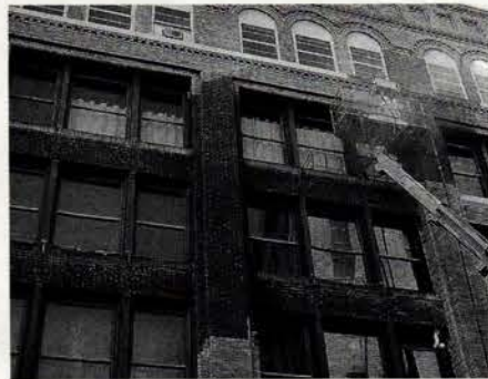
Armex blast media, a baking-soda-based abrasive from ArmaKleen, was used to clean this historic brick building.
