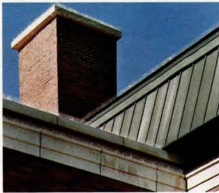
Stainless-steel bird barriers from Nixalite protect buildings from nesting birds.
