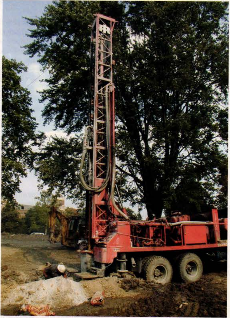
Above: The grounds at the Motherhouse of the Sisters, Servants of the Immaculate Heart of Mary in Monroe, MI, were torn up for several months during the installation of the large closed-loop geothermal system. It incorporates 232 boreholes, each 450-ft. deep, connected by 47 miles of pipe. Photo: Denyse Burkhart
