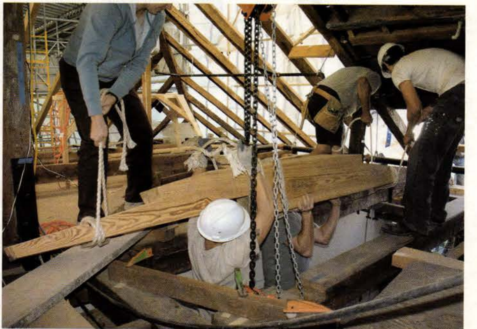
One of the beams that ties Montpelier's portico to the house had rotted clean through, so a 12-ft. section in the middle had to be replaced. Bolted scarf joints united replacement material with the original fabric. Reclaimed heart-pine timbers were salvaged from a textile mill in South Carolina. Photo: Maggie Wilson
