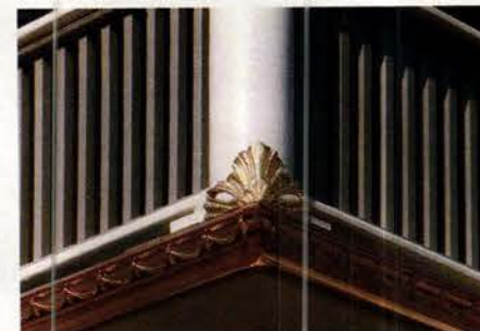
This ornate gutter, fabricated by Classic Gutter Systems, incorporates a hidden nuts-and-bolts adjustable hanger system.
