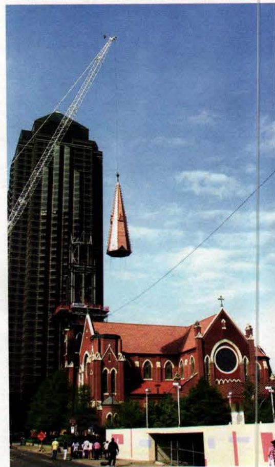
After the steel frame was built and the cladding was added to the top portion of the spire, copper steeples were lifted to the top of each tower. Photo: courtesy of Architexas
