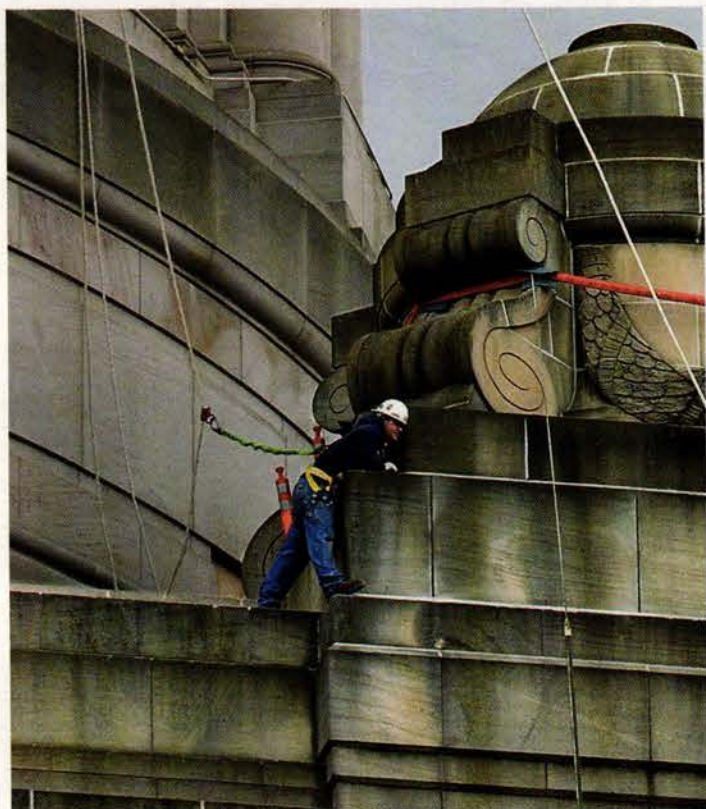
Above and right: All of the exterior surfaces were cleaned, repaired and recaulked, including the four mini-domes and the capitals. Photos: Dick Milligan
