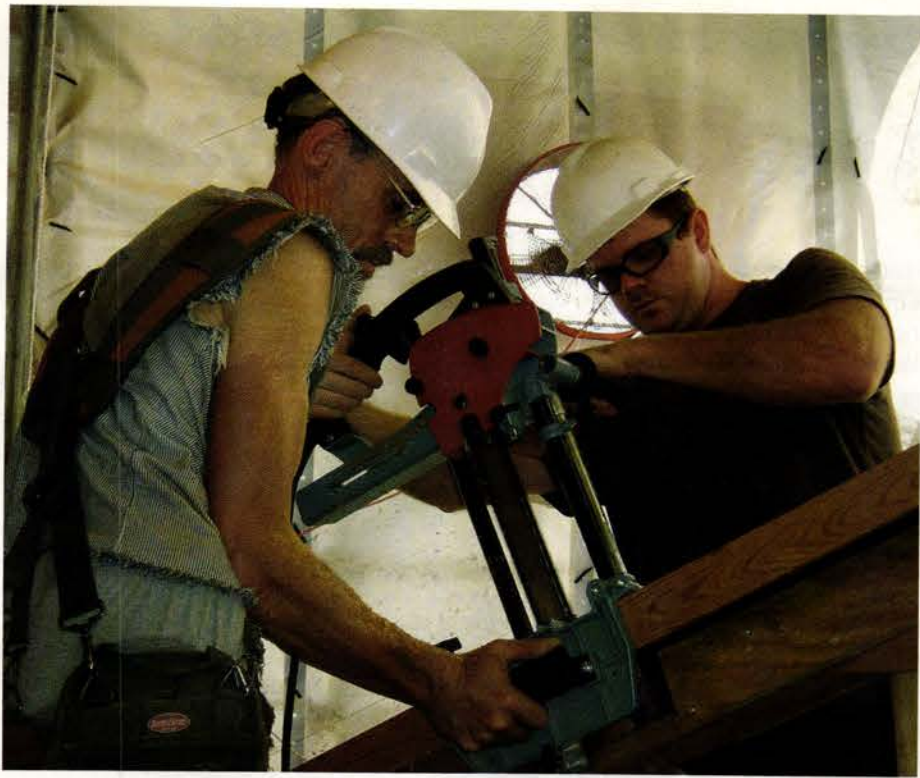
A spliced hip rafter was grooved with a chain mortiser to receive internal steel knife plates. Photo: Amy Wysocki
