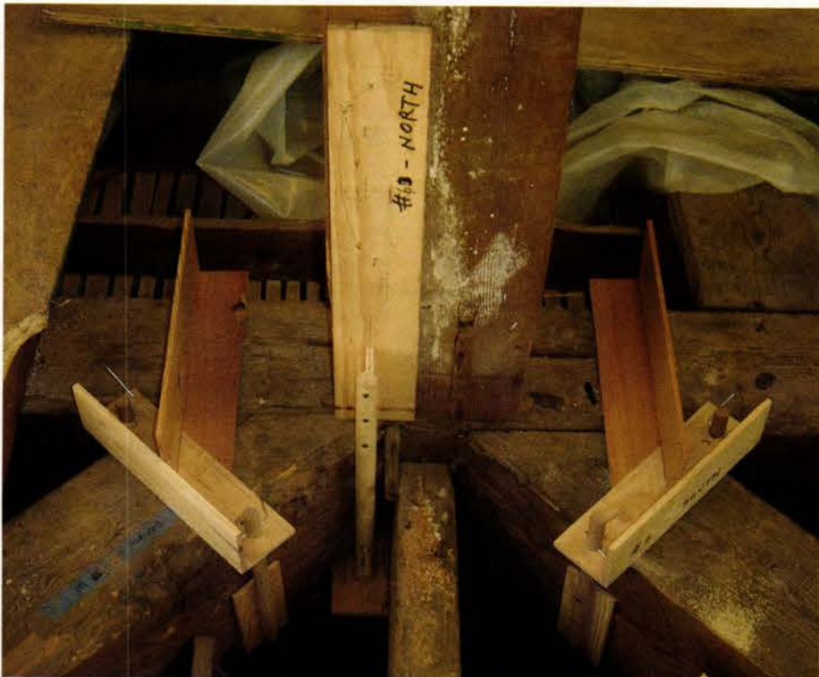
Two dragon beams, a joist and a kingpost all converge at the midpoint of the principal roof truss. The resulting mortises weakened the lower chord of the truss to the point of failure. After jacking up the truss, wooden patterns were made for specially designed steel hangers. Photo: Amy Wysocki
