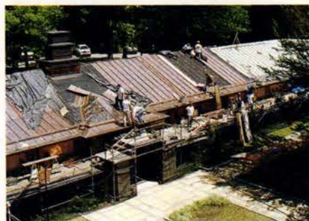
NIKO Contracting installed the batten-seam and flat-lock copper roof of the Kingswood School in Bloomfield Hills, MI.
