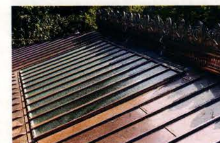
Charles River Restoration designed, fabricated and installed this replacement skylight for the approximately 100-year old skylight on the Stonington, CT, Library.
