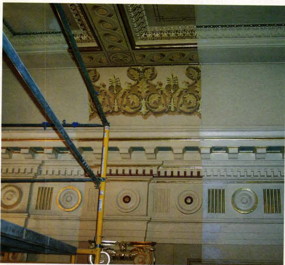
In the Senate and House chambers, as elsewhere, wonderfully detailed paintwork had been covered up over the years. The design team was able to uncover sections that plainly showed the building's original paint colors and designs, which are now being carefully reproduced. Photo: Kim A. O'Connell
