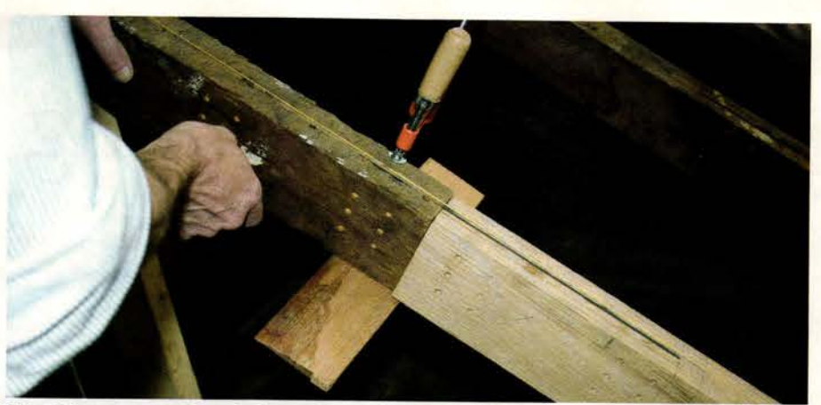
This 18th-century rafter (left) was severed in 1901 to accommodate roof alterations. A new extension (right) was attached by means of an internal steel knife plate that bridges the joint. The plate drops in from the top and is secured by four sets of self-drilling steel pins. Photo: Maggie Wilson
