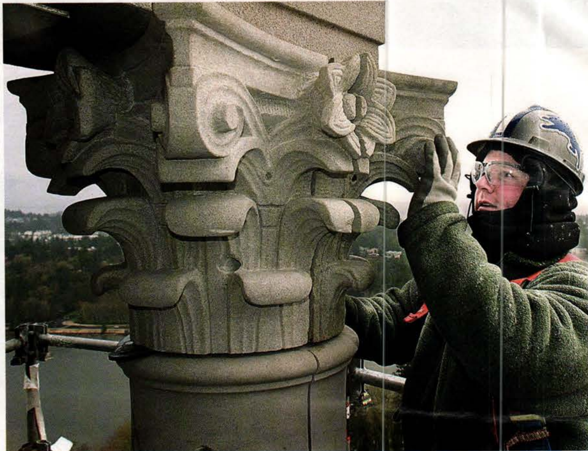
Above and right: All of the exterior surfaces were cleaned, repaired and recaulked, including the four mini-domes and the capitals. Photos: Dick Milligan
