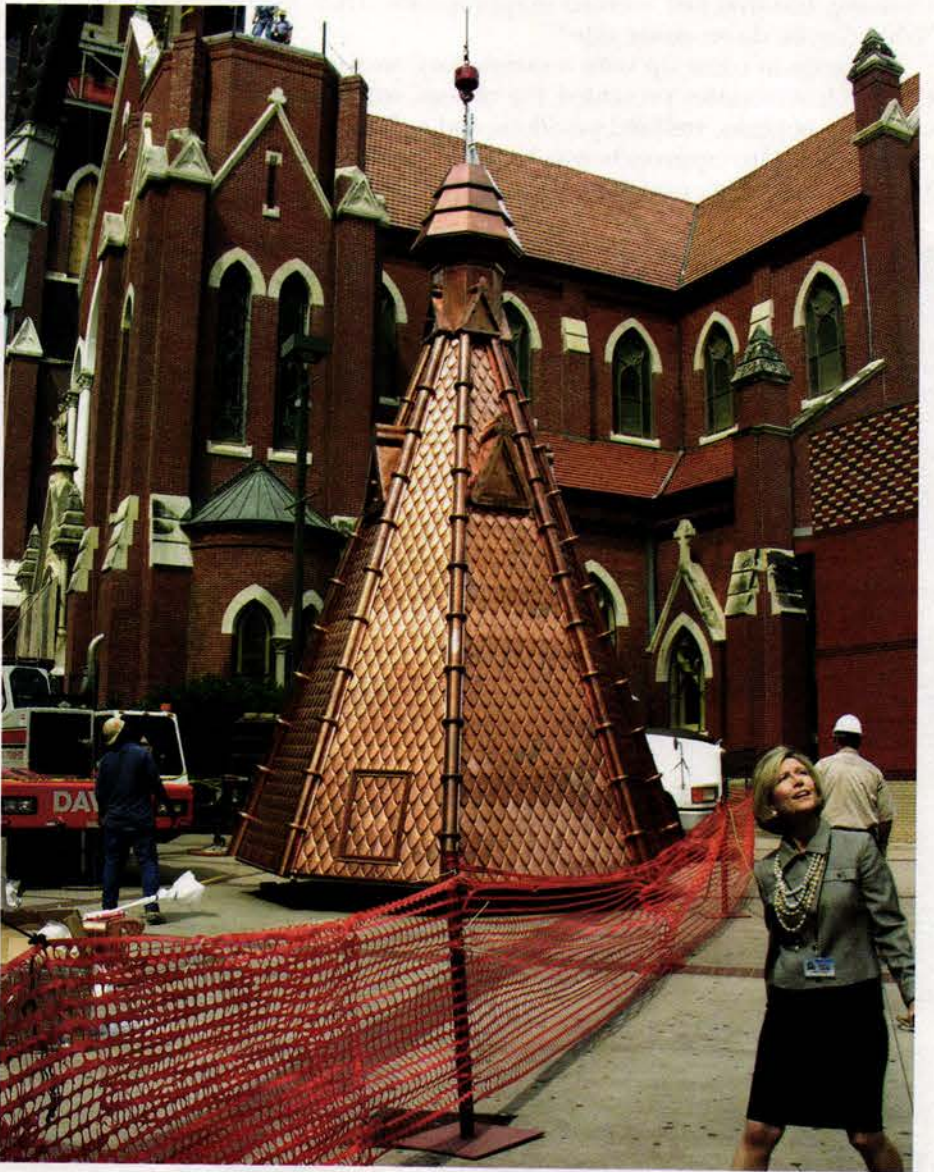
One of the last steps in the restoration was lifting the smaller spire to the top of the shorter tower. Photo: courtesy of Architexas
