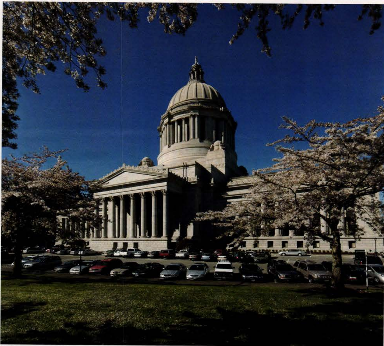
The $120-million restoration of the Washington State Legislative Building in Olympia, WA, added contemporary systems while maintaining the historic fabric of the 75-year-old structure. The masonry dome, which reaches a height of 287 ft., was secured so that the building is now ready to withstand another earthquake and to serve the public for at least another 50 years. Photo: Doug Walker Photography
