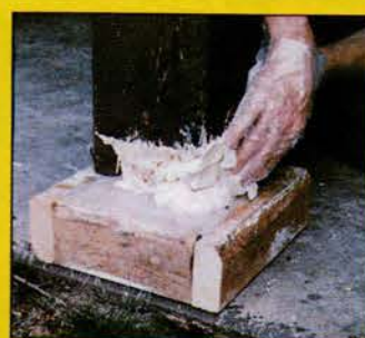
Rotted & infested base of a loadbearing column is completely sawed off & replaced with WoodEpoxy .
