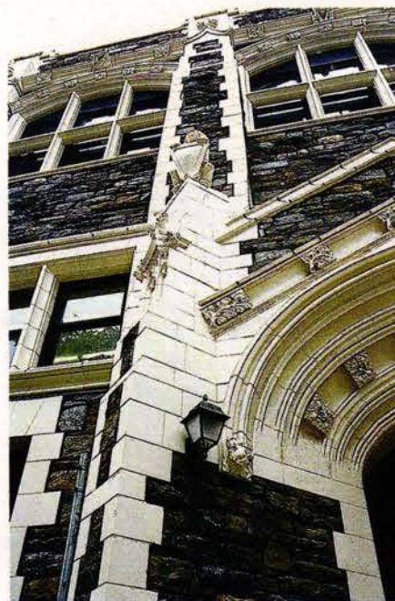
Gladding, McBean supplied the replacement terra-cotta elements on this building's façade.
