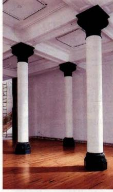
The old-growth heart pine flooring was remilled by Goodwin Heart Pine and installed in the oldest building in Key West, FL, to match the existing flooring.
