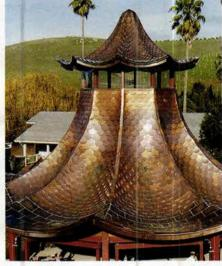
Vulcan Supply custom fabricated the shingles for this copper pagoda in its Vermont shop before completing the installation on-site.
