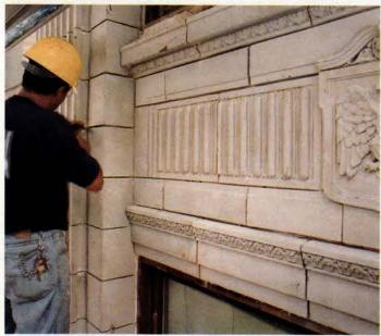
Polonia Architectural Restoration repointed where all mortar had powdered out between Keister's molded blocks, including cartouches of eagles clutching shields (right). Photo: Bernstein Associates
