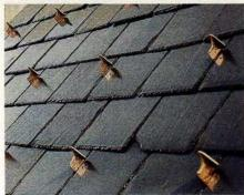
M.J. Mullane's BronzeGuard snowguards are designed for use on slate, shingle, shake, tile and metal roofs.
