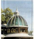
This glass and lead-coated copper dome was designed and constructed by Tanglewood Conservatories for a naturally stained mahogany con-
