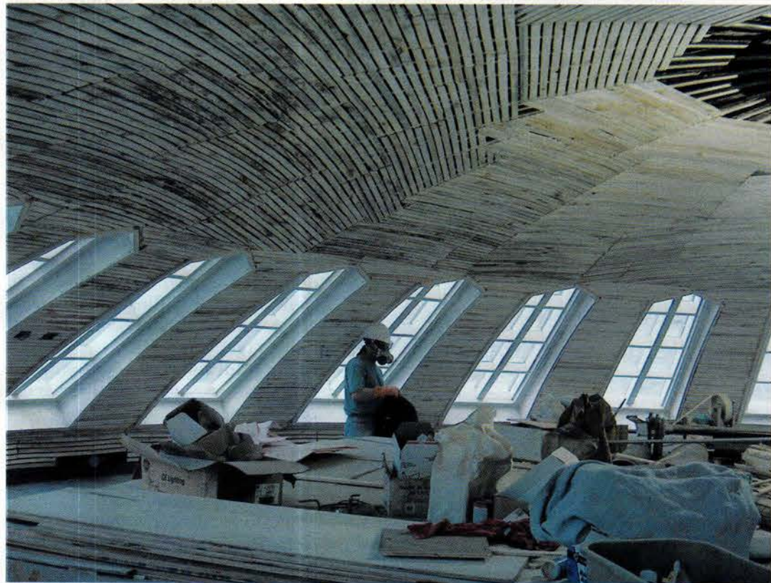
Above: The architects specified historic materials for the 77-ft.-dia. main dome – wood lath and lime plaster – to follow Latrobe's intent and because they realized that these materials had the flexibility needed to accommodate the movement of the outer wooden dome. Photo: courtesy of the Baltimore Basilica
