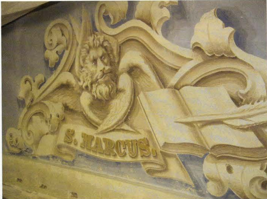
EverGreene painters restored the four murals that were discovered hidden behind a later plaster surface in the main drum of the building. They date from 1865 and were restored in place. Photo: courtesy of EverGreene Studios
