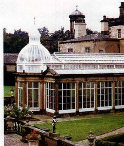
Each of the curved, double-glazed, laminated glass units for the domed conservatory of England's Broughton Hall were individually made by Oak Leaf Conservatories.
