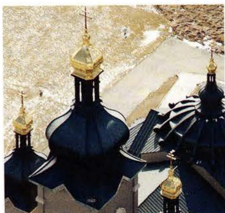
Heather & Little custom fabricated four copper-clad domes for the Church of the Transfiguration in Markham, ON; the upper domes are adorned with 22k gold leaf.
