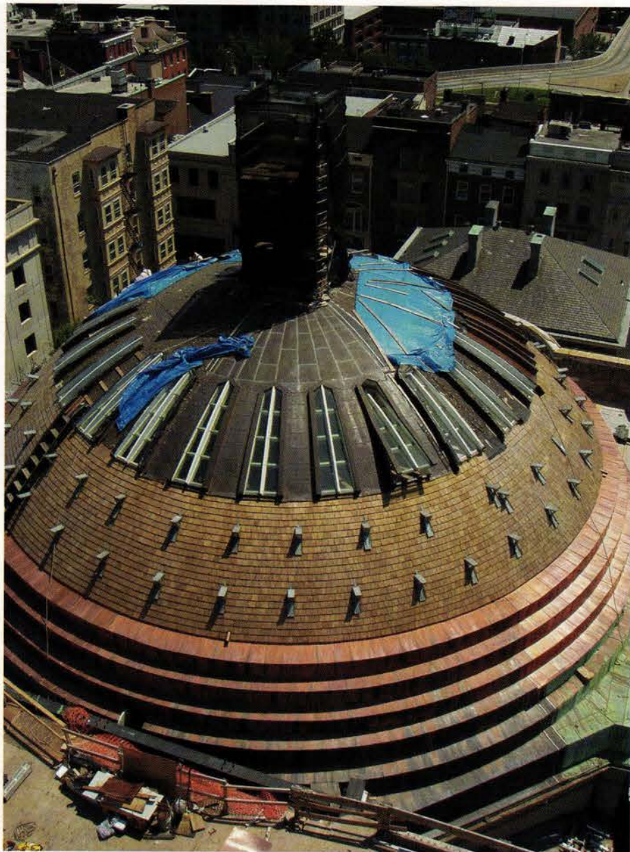
The roof of the main dome is wood shingle up to the perimeter of the wood frame, then new copper sheathing was added. The 24 skylights that had been covered during World War II and then later removed are back in place. Photo: courtesy of the Baltimore Basilica
