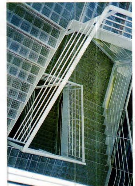
Circle Redmont's 71R solid glass paver & precast concrete panel system was used to create this stairway.
