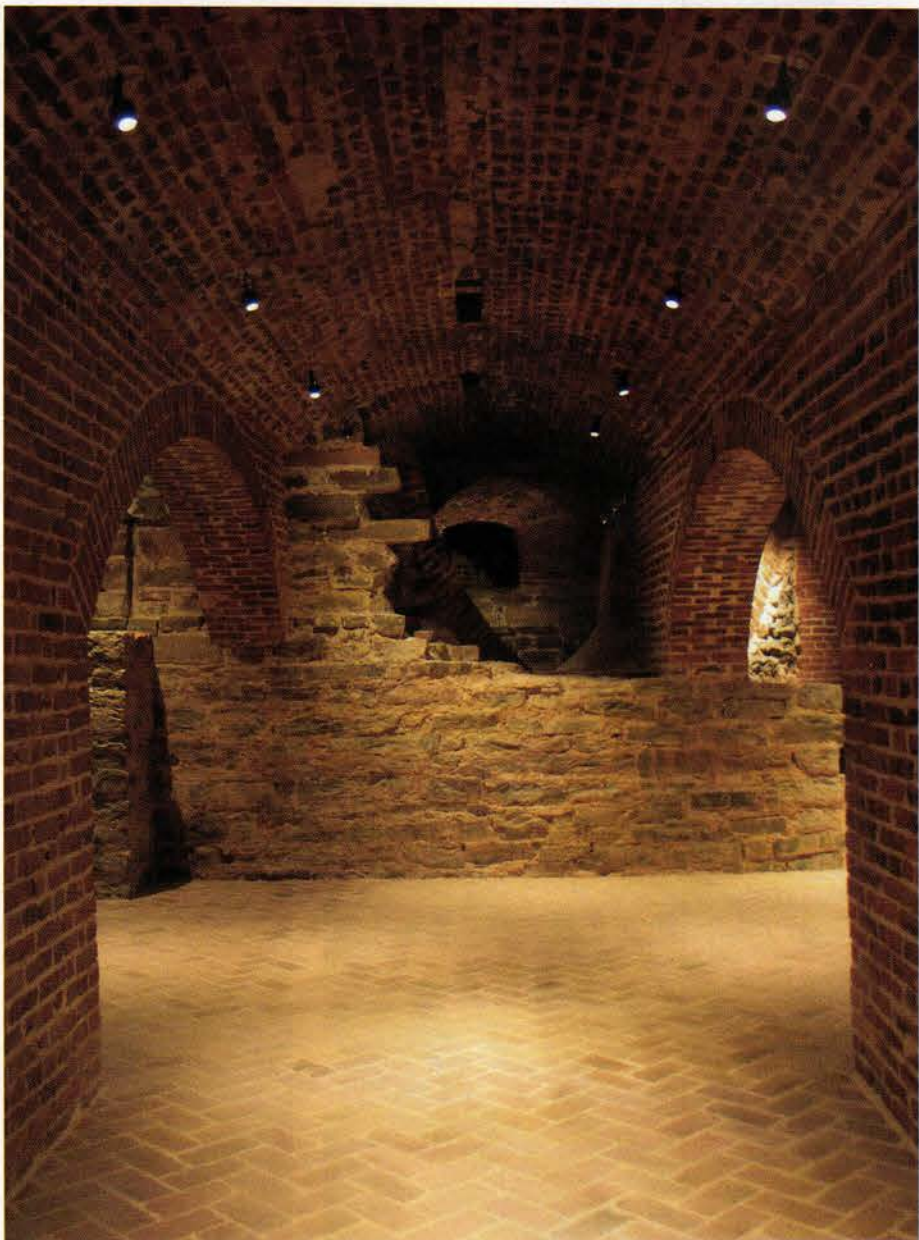
Made of a series of arches and vaults, the undercroft of the Baltimore Basilica now houses a small chapel and museum, as well as the crypt. Some of the original brick had to be removed to create an entry to the crypt. Photo: courtesy of John G. Waite Associates
