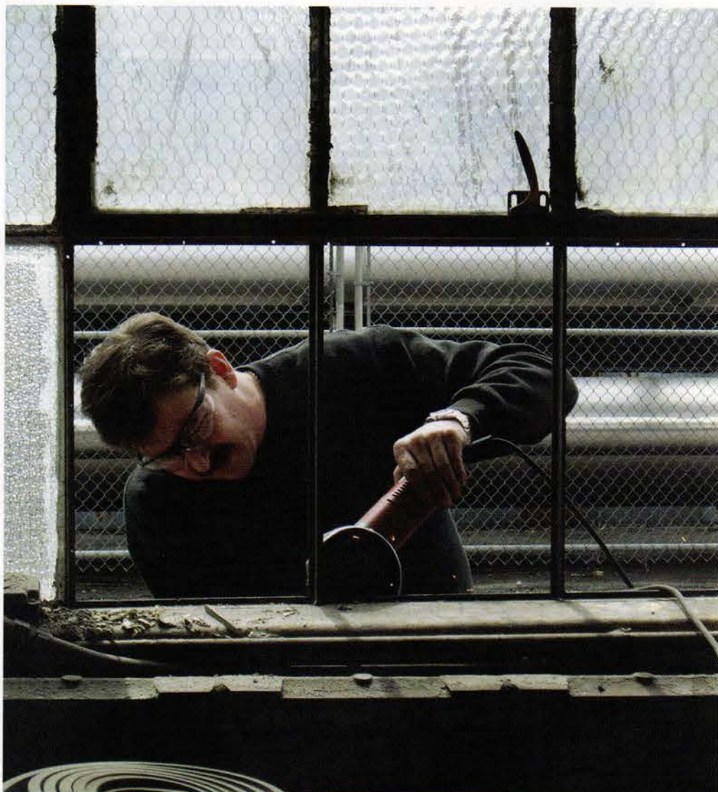
John Seekircher's team, which included his brother Robert (pictured), carried out the restoration in less than eight weeks, replacing more than 1,300 panes of glass and repairing and replacing missing steel and hardware.
