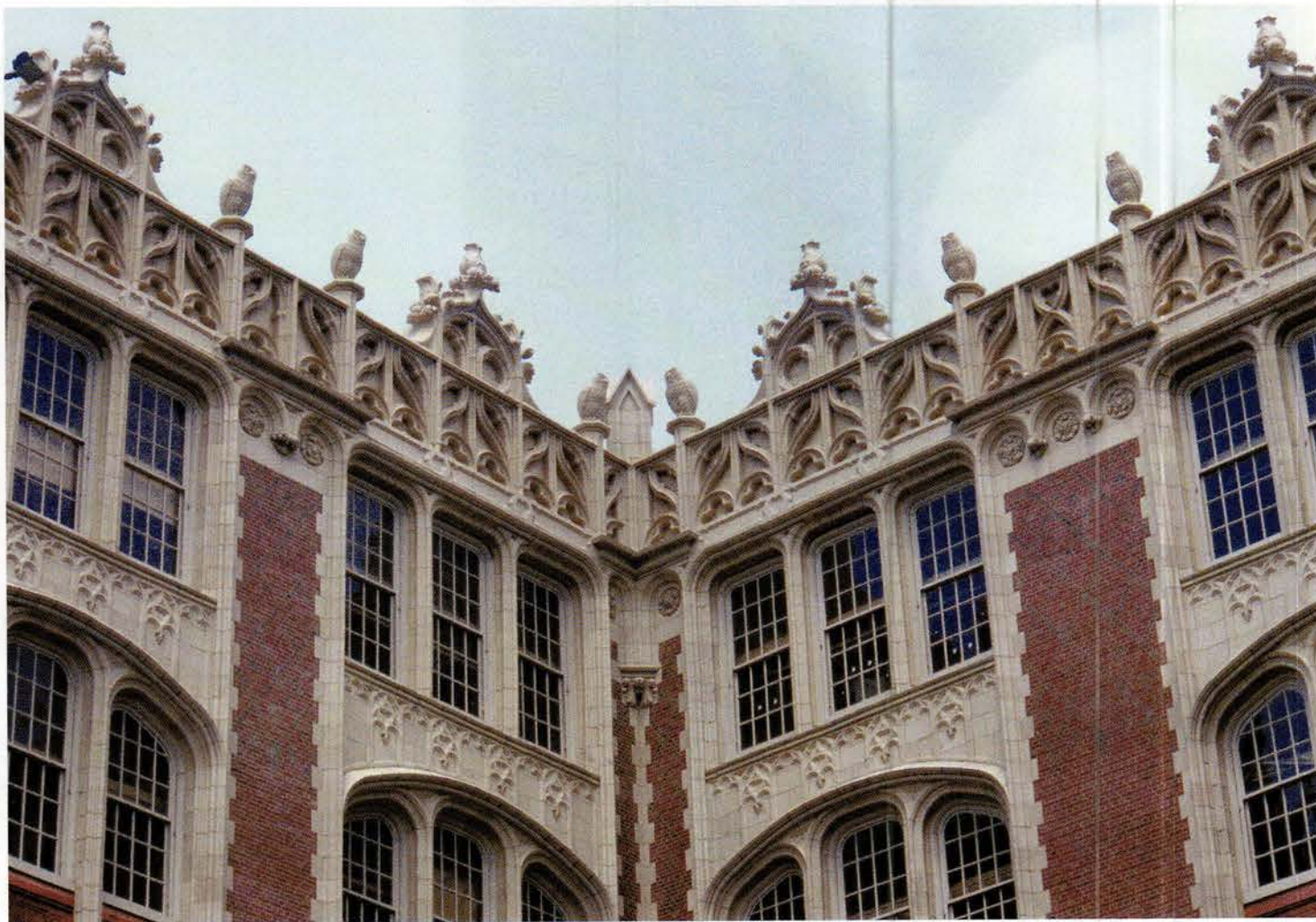
Highlighting the Gothic Revival architectural style of P.S. 157 in Brooklyn, NY, are its terra-cotta copings, mullions and ornament, complete with watchful owls. Extensive failure of the terra cotta had marred the building's exterior until Gladding, McBean was brought in to replicate the missing details. Photo: Mary Swisher
