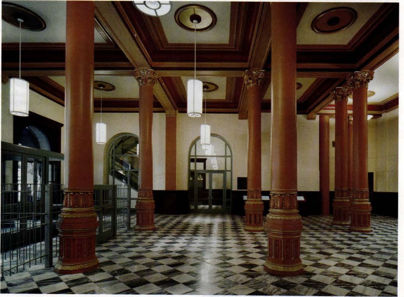
The new marble flooring and restored decorative painting in the entry hall of the U.S. Bankruptcy Court mirrors that throughout the majority of the building. The flooring, supplied by Georgia Marble of Tate, GA, is Solar Gray, Black Champlain and Imperial White marble. It offsets the Victorian-style polychromatic color scheme.
