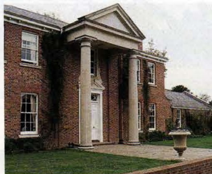
Haddonstone's cast-stone M1 columns were used with Doric capitals to create the Classical entryway for this building.
