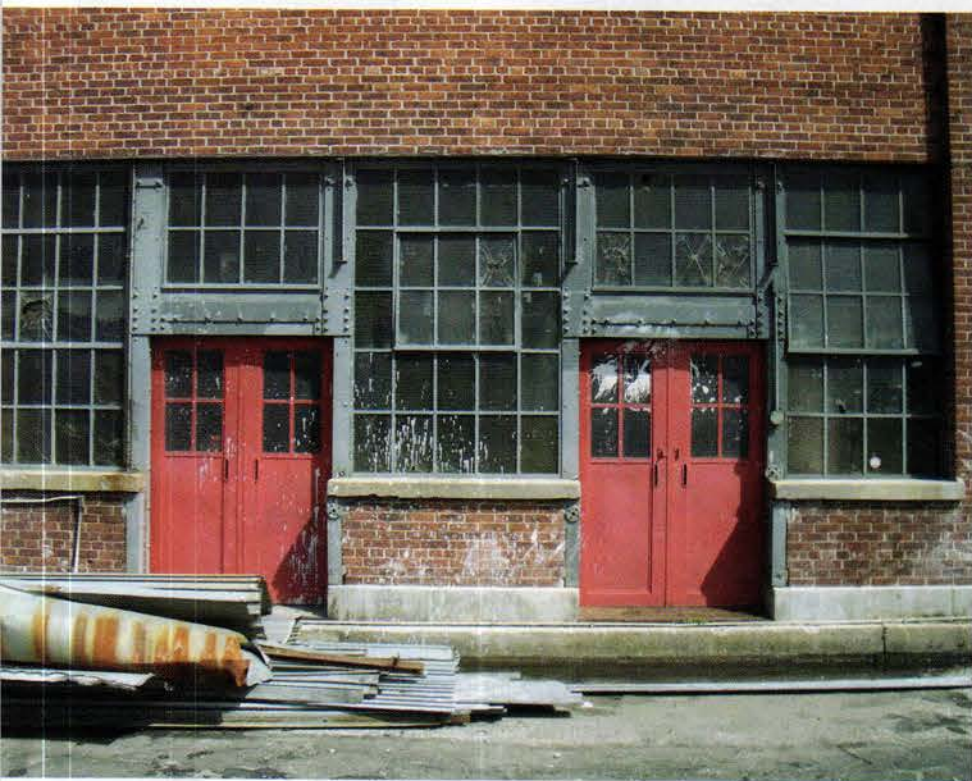
Many of the original window frames were misaligned or missing hardware or glass, resulting in substantial thermal loss and making the building look unattractive.
