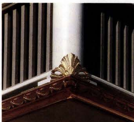
This ornate gutter, fabricated by Classic Gutter Systems, incorporates a hidden nuts-and-bolts adjustable hanger system.
