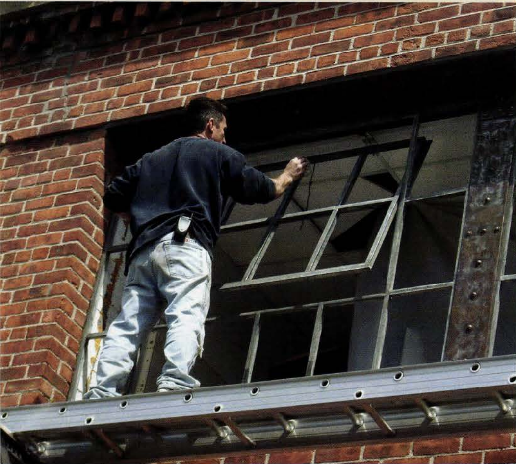
Some of the windows were operational and required only replacement 1/4-in. laminated glass, stripping and painting; others were permanently open.
