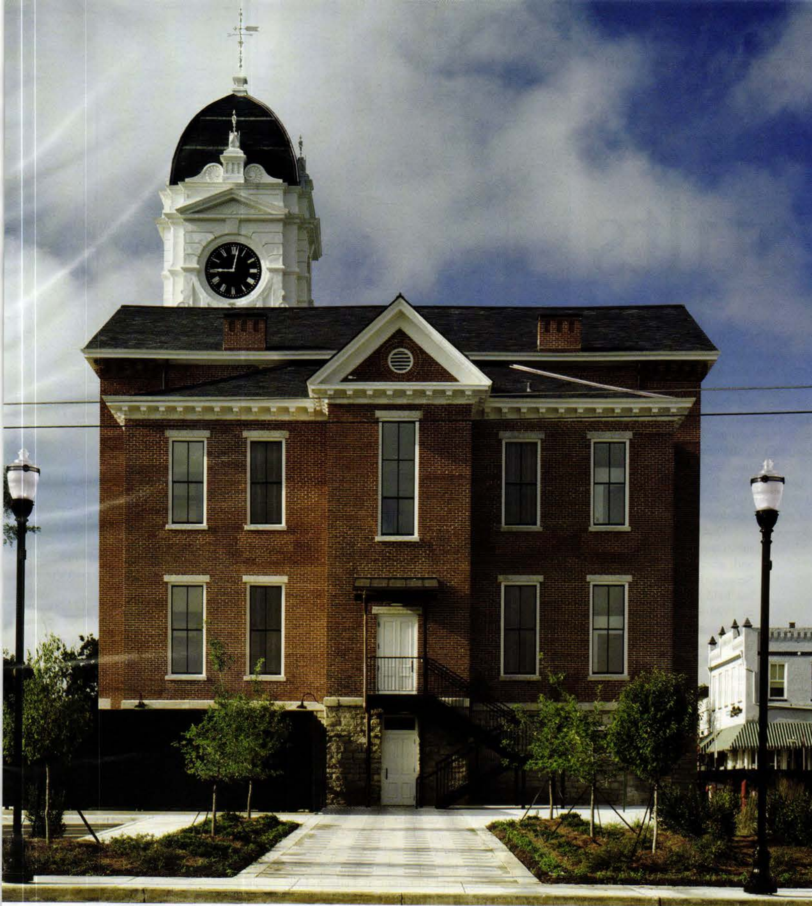
On the exterior, the process of recapturing the courthouse's historic character included restoring the slate roof and windows to their original appearance.
