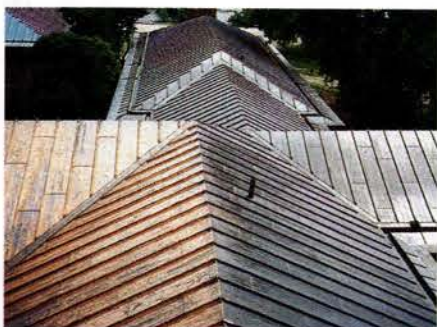
NIKO installed this batten-seam and flat-lock copper roof.
