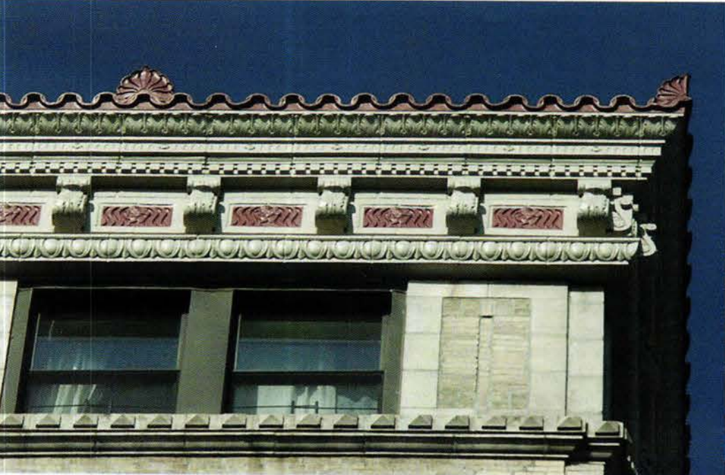
The terra-cotta cornice at 327 Central Park West in New York City is actually a replication in FRP, produced by Architectural Fiberglass Corp. Both colors were molded into the fiberglass, which is lightweight enough to permit the firm to produce numerous “terra cotta” components in single, modular units measuring 6 ft. long and weighing less than 150 lbs. Photo: courtesy of Architectural Fiberglass Corp.
