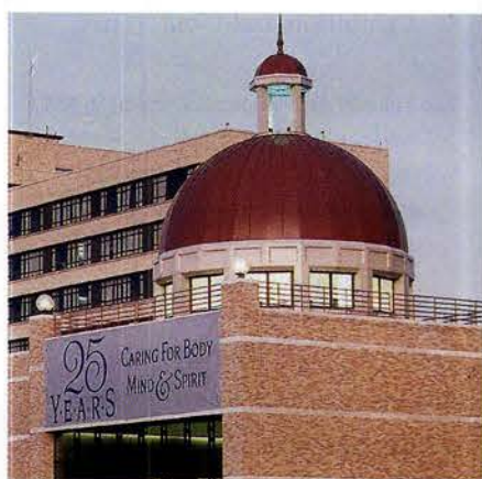
The main dome and matching cupola for the Presbyterian Hospital in Dallas, TX, were clad in aluminum with standing-seam panels by CopperCraft.
