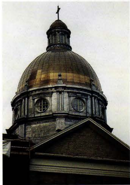
Heather & Little restored the lead-coated-copper dome and cupola for Our Lady of Lourdes Roman Catholic Church in Toronto, Canada.
