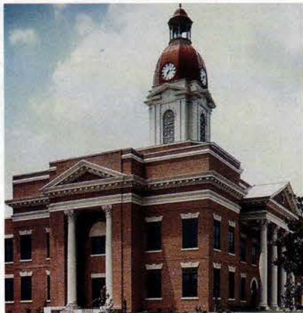
This aluminum cupola, with a 6-ft.-dia. clock and aluminum cornice, was created for the Worth County Courthouse in Sylvester, GA, by Campbellsville Industries.
