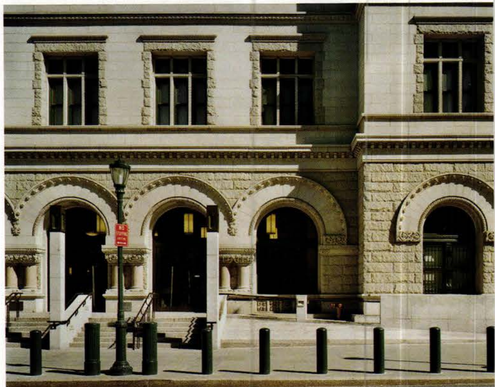
Kliment & Halsband added granite stairs and a ramp that access a new plaza along the west side of the building. New pylons, along with site lighting and railings, call attention to the entrances, some of which were enlarged to permit an increase in pedestrian traffic.
