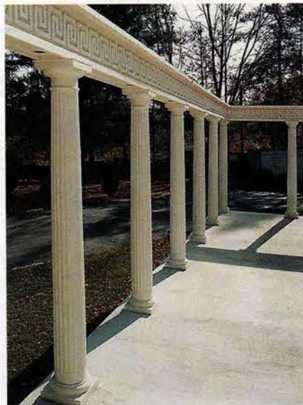
Manor Style's load-bearing, fluted fiberglass-composite column and custom-fabricated PVC Greek Key-patterned beam adorn this patio.
