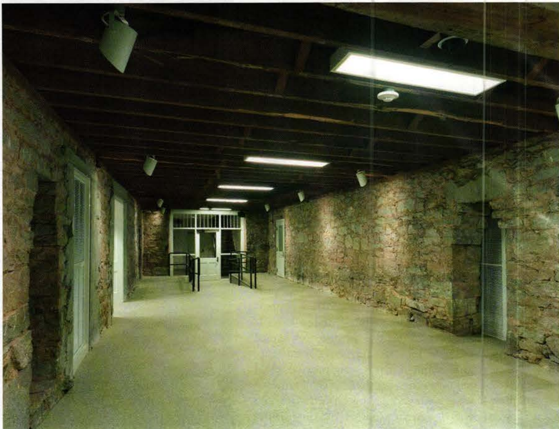
In the non-historical demolition phase, original rubble walls were discovered behind paneling that had been added in the mid-20th century.
