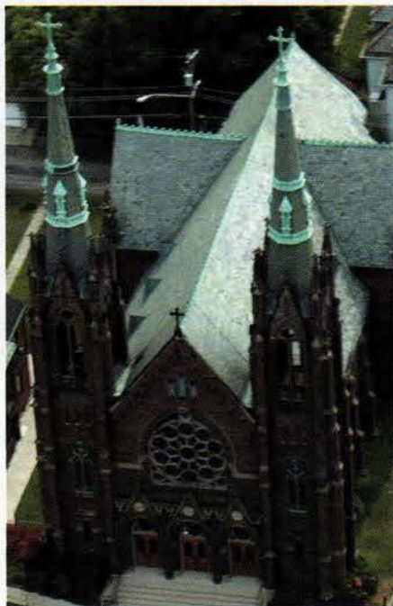
The Durable Slate Co. repaired the slate roof and replaced copper valleys, ridge roll, the copperwork at the base of the steeples and the custom-fabricated copper gutter system for this century-old church and rectory in Ohio.
