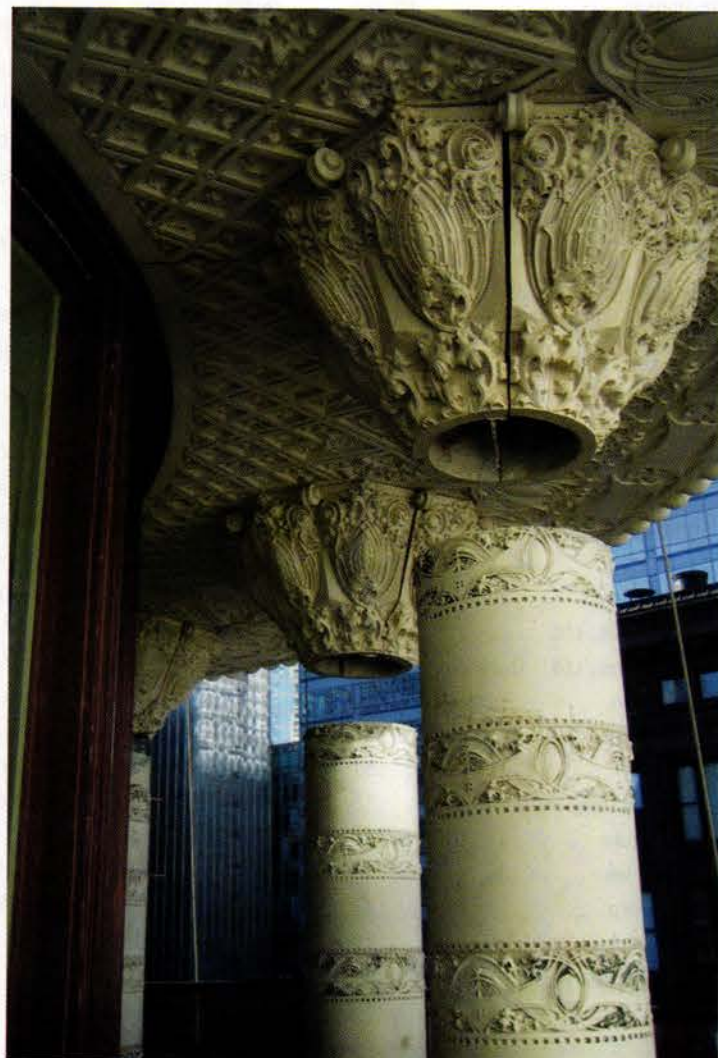
To recreate the cornice and colonnade – including capitals, column banding, soffits and fascia – 13 unique ornament masters were combined.
