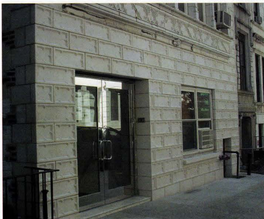
The cast-stone experts at Towne House Restorations decided to tackle this job in GFRC. The lower section of 126 West 73rd Street in New York City, a 13-story 1915 apartment building, designed by architects Buchman & Fox, was originally faced in white terra cotta. It eventually suffered damage caused by the deterioration of its original anchoring system – a familiar fate for architectural terra cotta of an earlier era. Photo: courtesy of Towne House Restorations
