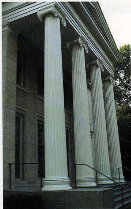
Fagan Design replicated this 30-in.-dia. x 20-ft.-tall fluted column (foreground) to match the existing columns.
