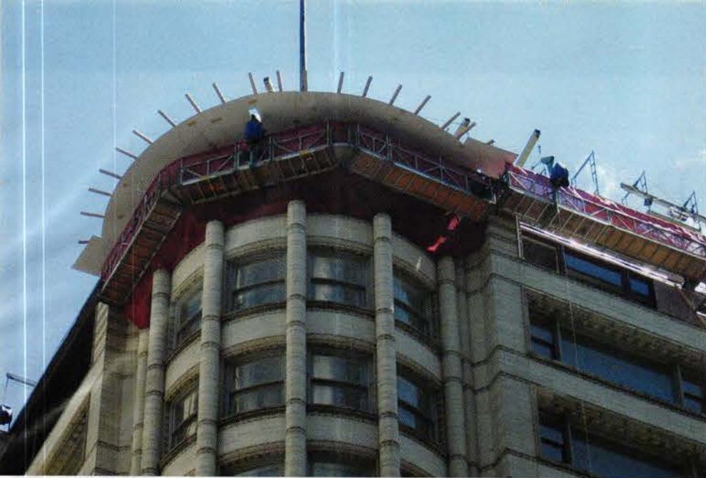
The architects modified full-scale plywood templates six times before successfully matching the rotunda's existing construction to ensure that the new cornice panels would fit properly.
