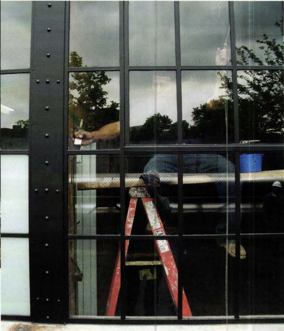
Some of the windows were operational and required only replacement 1/4-in. laminated glass, stripping and painting; others were permanently open.
