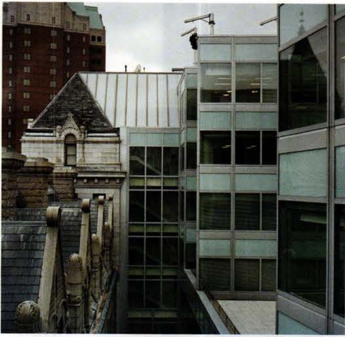
Above: A four-story, U-shaped, painted-aluminum and glass curtain wall encloses the U.S. Attorney's Office, one of the four tenants in the building. Kliment & Halsband designed it to meet the Secretary of the Interior's Standards, clearly contrasting new and old. The height of the addition does not exceed the existing roof line so it can not be seen from the street.
