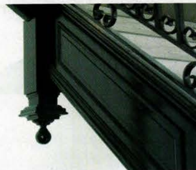
O.K. Foundry fabricated this custom cast-iron stairway fascia and newel post cap for the restoration of the Virginia State Capitol.
