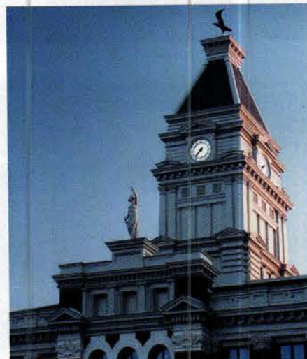
Campbellsville Industries fabricated the clock tower, clock, decorative cornice, modillions, paneled railing and corner pediments for the restoration project at Montgomery County Courthouse in Clarksville, TN.
