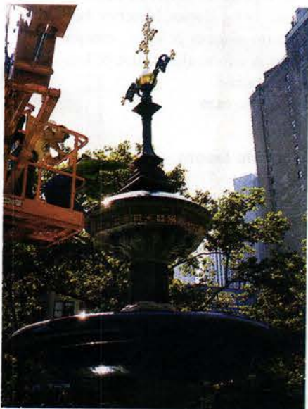
The ornamental bronze spire of the Jacob Wrey Mould Fountain in New York City's Central Park was replicated by Allen Architectural Metals.
