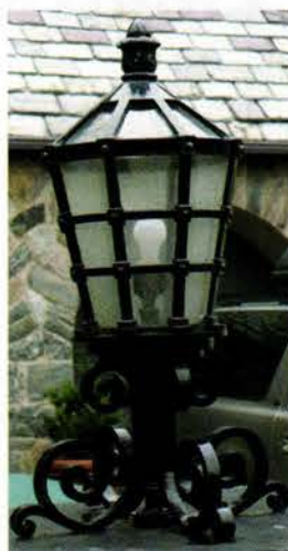
This pier-mounted reproduction lantern was fabricated by Fine Architectural Metalsmiths; it features a glassed-in cap and an acorn finial.
