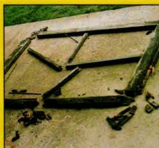
Antique window sash is salvaged, consolidated with LiquidWood & rebuilt with WoodEpox .
