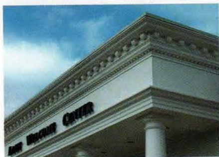
This cornice was built using pre-finished architectural urethane multi-profile moldings supplied by Melton Classics.
