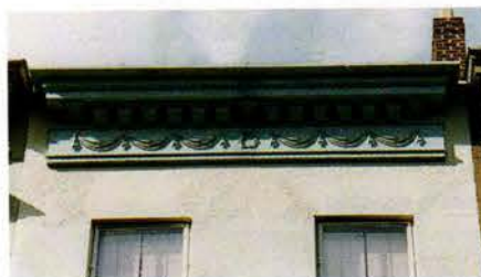
Seal Reinforced Fiberglass provided an FRP replica of the original metal cornice for this New York City building.
