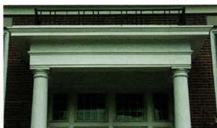
Molded fiberglass elements from Architectural Fiberglass were used to replicate historical moldings for this building.
