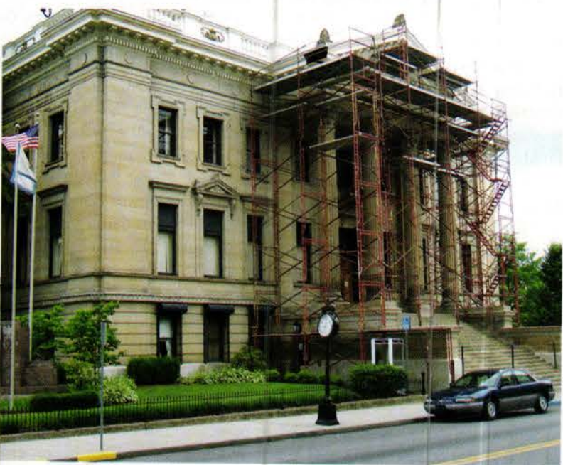
Above: Heavy-loading scaffolding was erected around the front entrance of the Marion County Courthouse while its cast-iron elements were repaired, cleaned and repainted.
