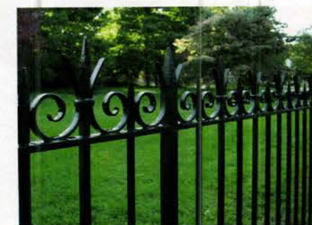
This custom fence was designed and fabricated by Wiemann Ironworks using solid-bar steel; to ensure longevity, it was galvanized before the urethane paint was applied.
