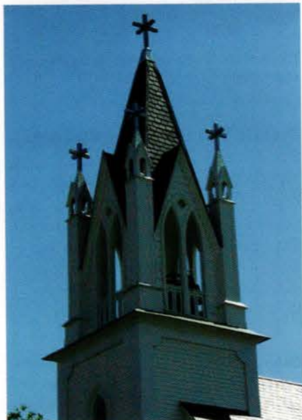
A new Canadian purple-slate roof with copper flashings, custom copper gutters and downspouts was installed on the Zion Lutheran Church in New Orleans by The Durable Slate Co. after Hurricane Katrina damaged the existing asbestos roof.
