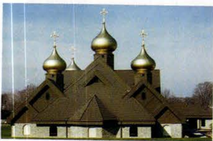
Five onion-style golden domes were custom manufactured and installed by Architectural Fiberglass on the Holy Trinity Church in Parma, OH; one measures 18x32 ft. and the other four are 15x26 ft.
