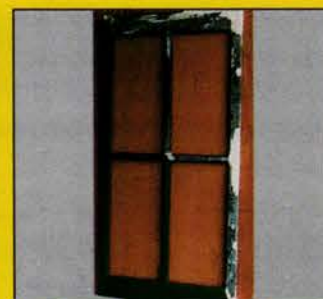
Antique window sash is salvaged, consolidated with LiquidWood & rebuilt with WoodEpox .
