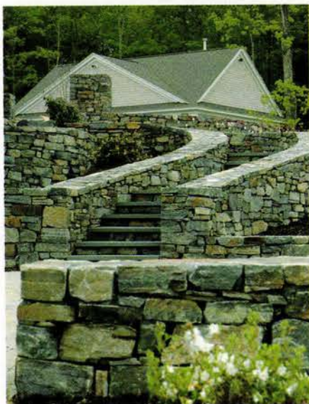
American Granite, a medium- to coarse-grain hand-split stone from Champlain Stone, was utilized in the creation of these steps and walls.
