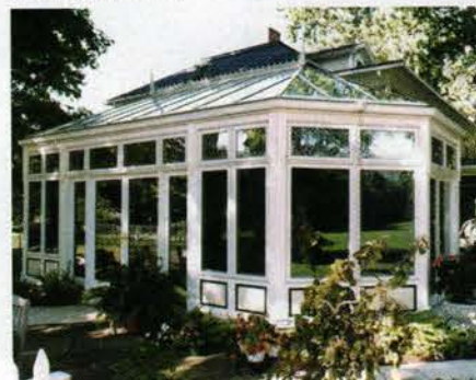
This conservatory by Glass House features custom details such as molding, gutters, downspouts, cresting and finials, leaded glass, French doors, interior ornamental eave bracketry and tension rods.
