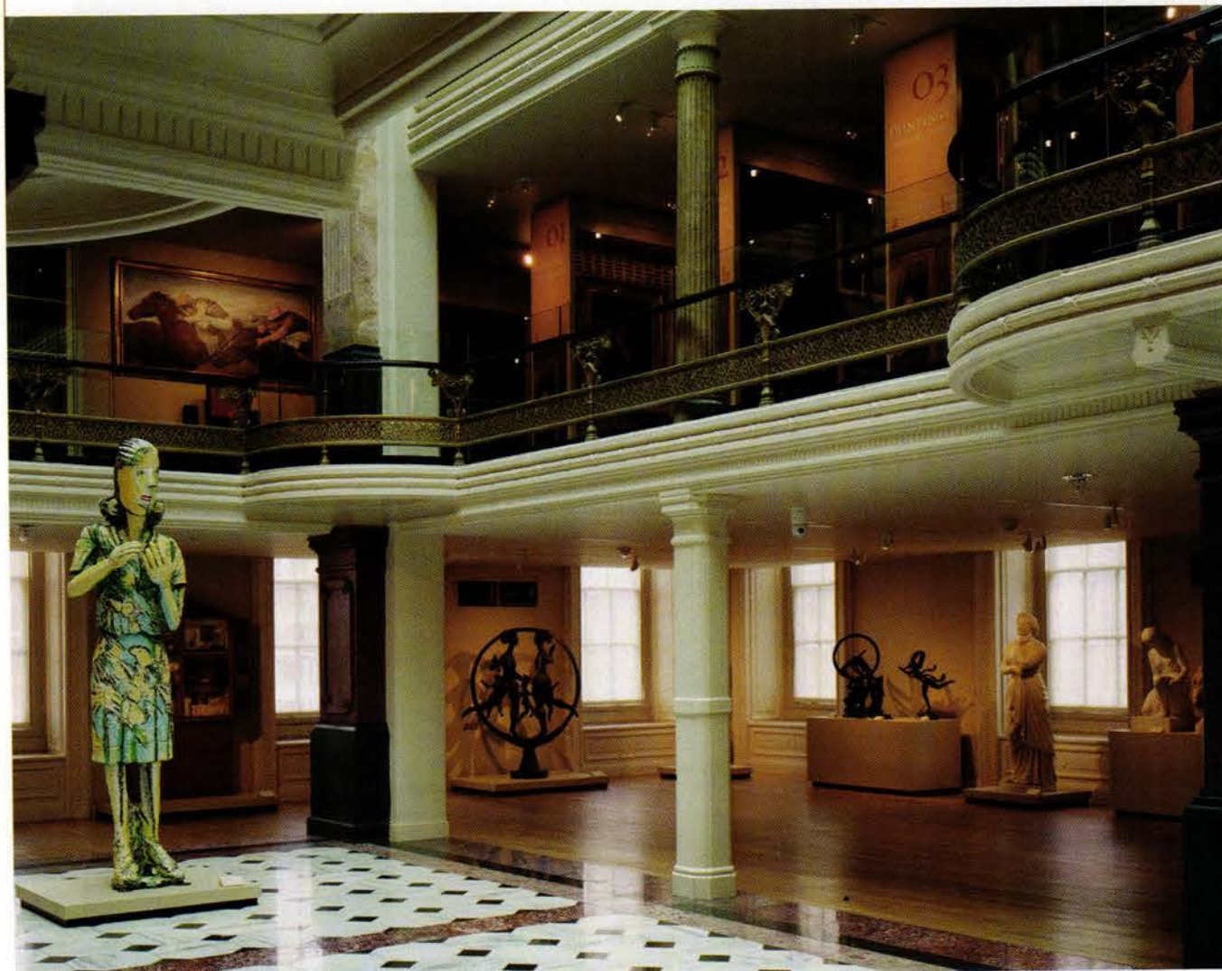
Cast-iron piers on a marble gallery floor support a mezzanine with cast-iron fluted columns.
