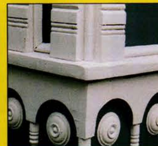
Antique window sash is salvaged, consolidated with LiquidWood & rebuilt with WoodEpox .
