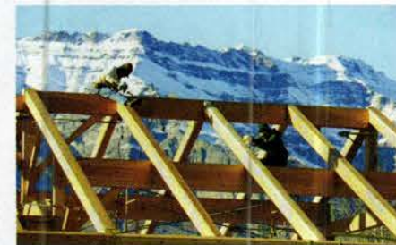
Reliance Specialty Building Products supplied the Douglas fir, hemlock, white fir, spruce and pine for this timber-frame structure.
