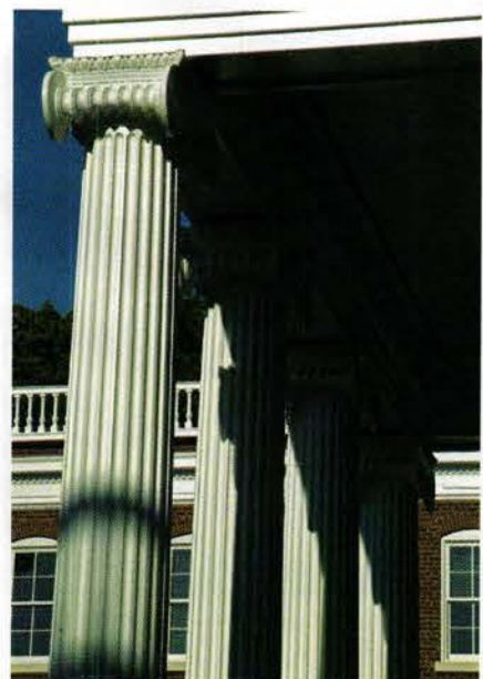
Melton Classics built these Greek Erechtheum Ionic columns in all-heart redwood for Longwood University in Farmville, VA.
