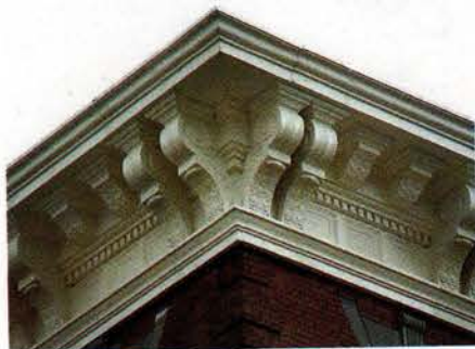
Architectural Fiberglass fabricated this 61-in.-tall cornice with a 30-in. projection for a restoration project in the Bronx, NY.
