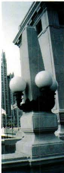
The city of Chicago commissioned Allen Architectural Metals to re-create these bronze obelisk light fixtures and cast-iron lampposts from original castings.
