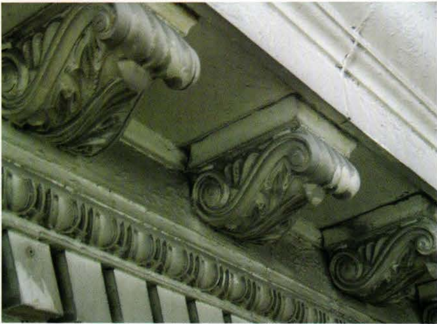
The white epoxy paint had failed in places, leading to cracks and potentially dangerous corrosion.
