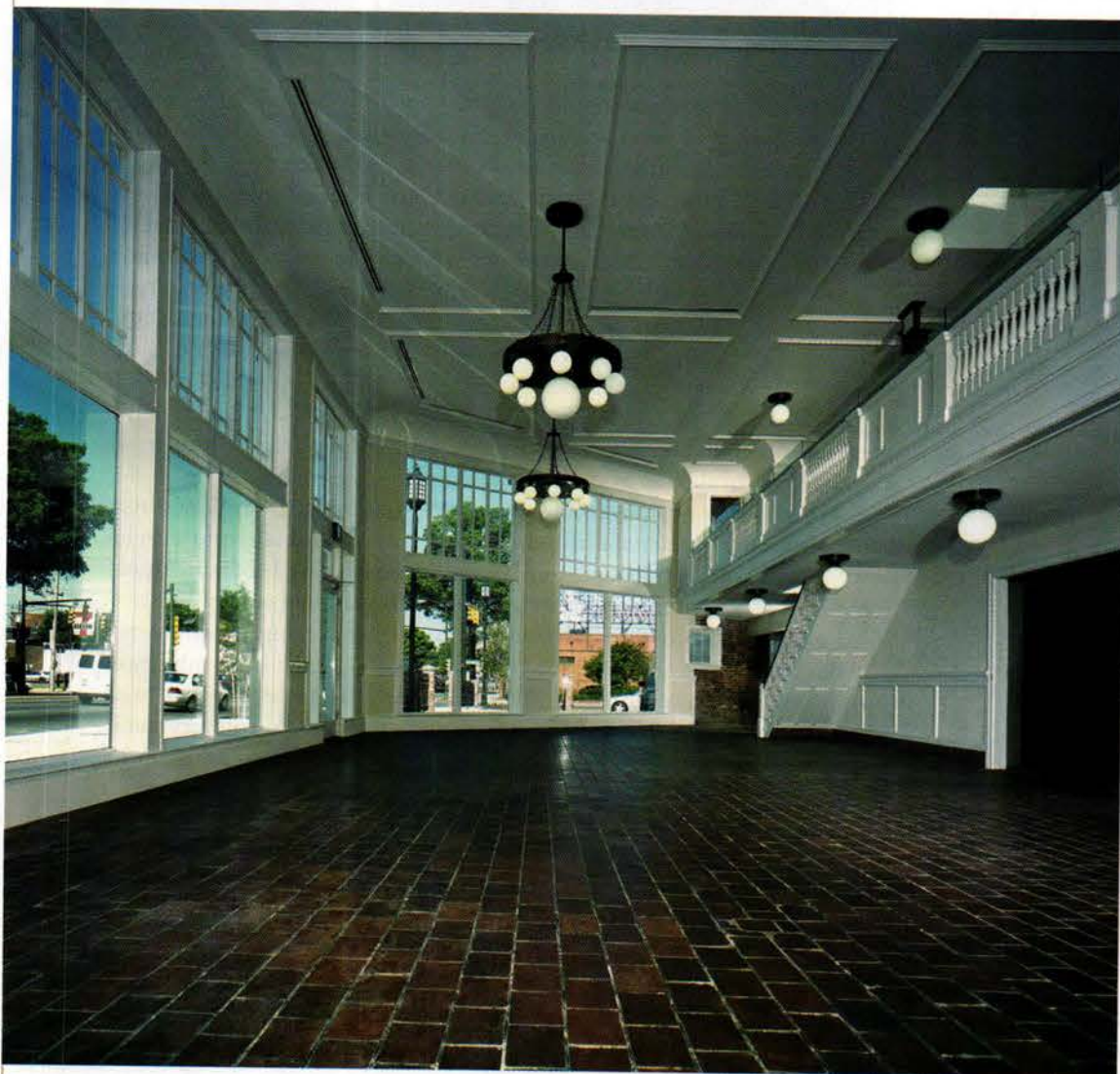
The old automobile showroom (above) had suffered water damage caused by leaks in the roof, necessitating the replication and reinstallation of plasterwork. New steel beams were added to the renovated space (left) and the ductwork was moved to the attic. The terra-cotta floor only required wet-mopping to return it to its original sheen. Before photo: courtesy of Commonwealth Architects; after photo: Lee Brauer Photography ©2006
