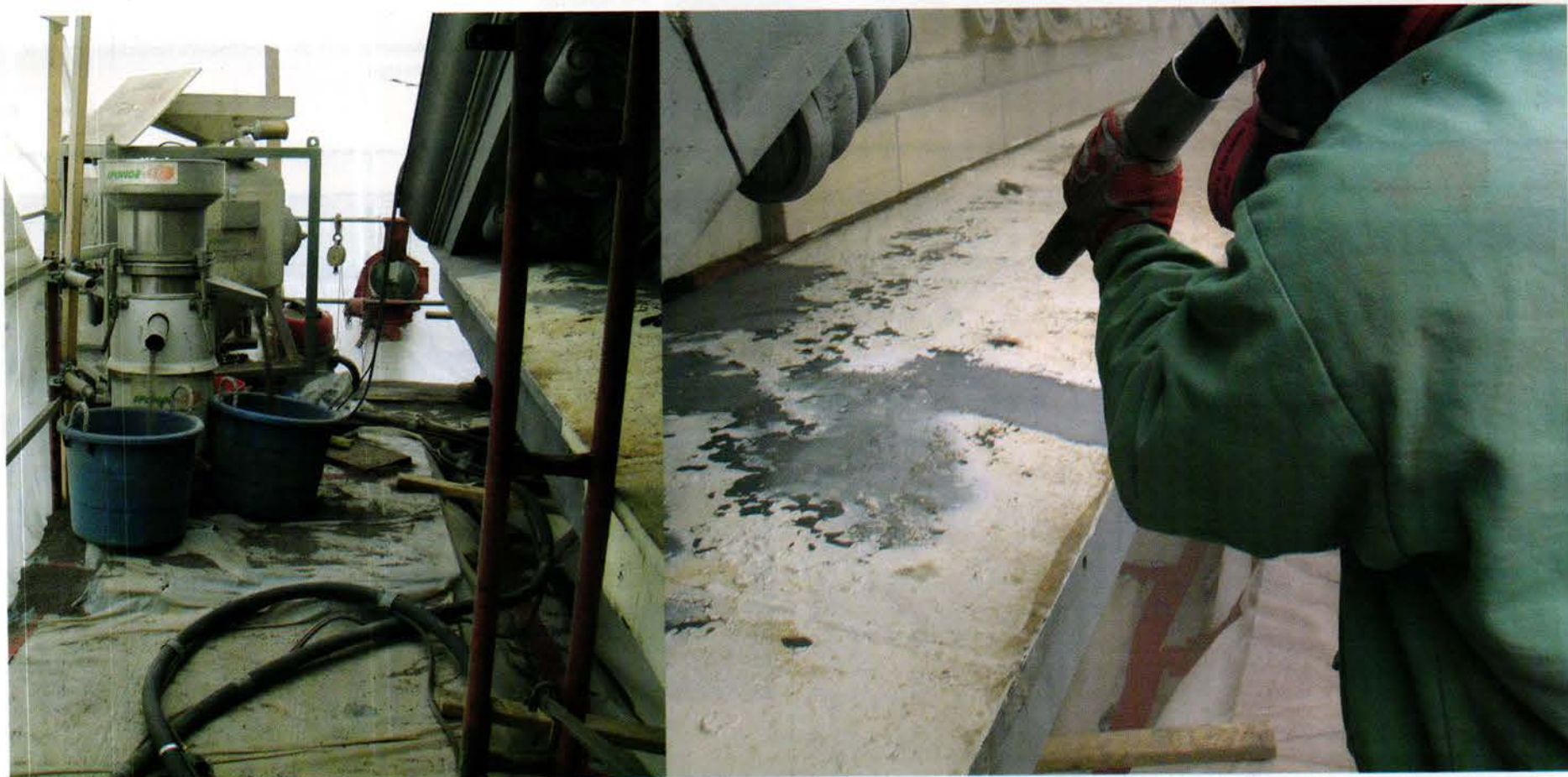
The Sponge-Jet blasting system was located on the same level as the work being done, allowing blasting and recycling to be carried out within feet of the blaster.
