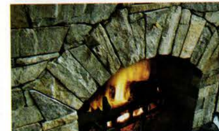
Champlain Stone's American Granite, used in this rustic fireplace, is medium- to coarse-grained and weathered to present an aged appearance.
