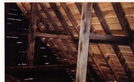
This timber-frame roof of this 60-ft. barn was replaced by Colonial Restorations using gin poles instead of a crane.
