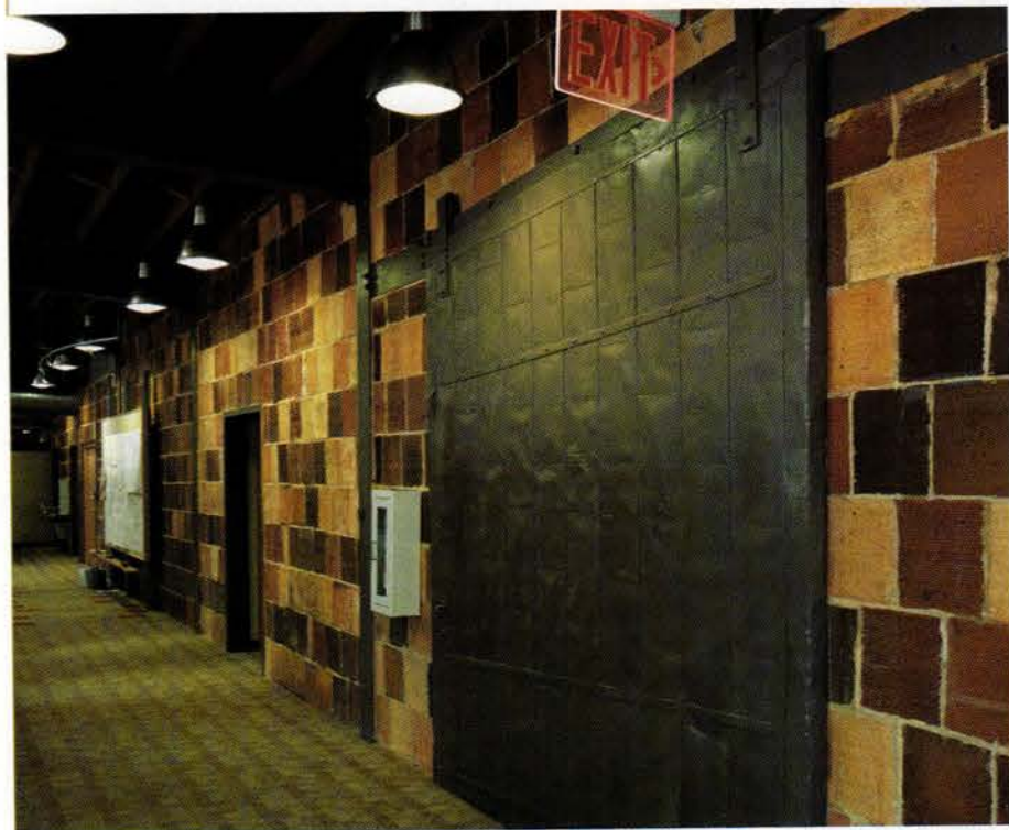
Dividing the north and south offices is a terra-cotta wall that was stripped of whitewashing and restored to its original color scheme. The metal door is another historic relic but is now fixed in place. Photo: Lee Brauer Photography ©2006
