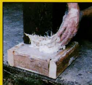
Rotted & infested base of a loadbearing column is completely sawed off & replaced with WoodEpox .
