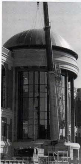
Campbellsville Industries installed this 55 1/2-ft.-dia. dome on the Warren County Justice Center in Bowling Green, KY.
