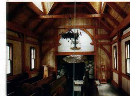
Timberpeg built the Douglas fir frame, vaulted ceiling, triangular skylight windows and bell tower of this chapel near Los Angeles, CA.
