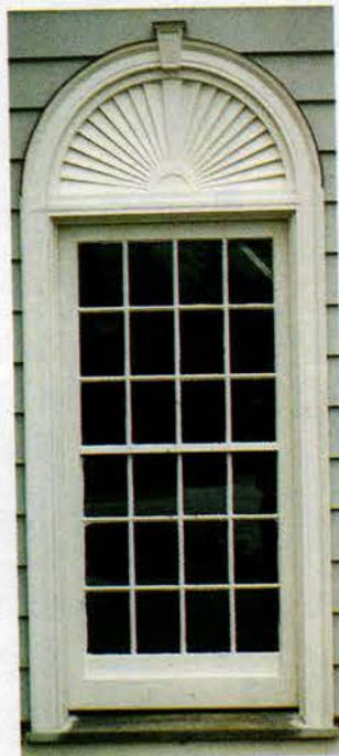
This reproduction 12/12 window with fan was fabricated by Architectural Components.
