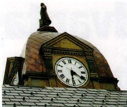
The dome on the clock tower of the Hancock County Courthouse in Findlay, OH, was sheathed in new copper by NIKO; the firm also replaced the slate roof as part of the restoration.
