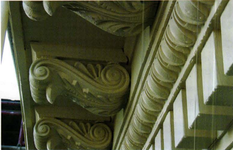
The cornices were re-anchored to the façade before being cleaned and repainted.
