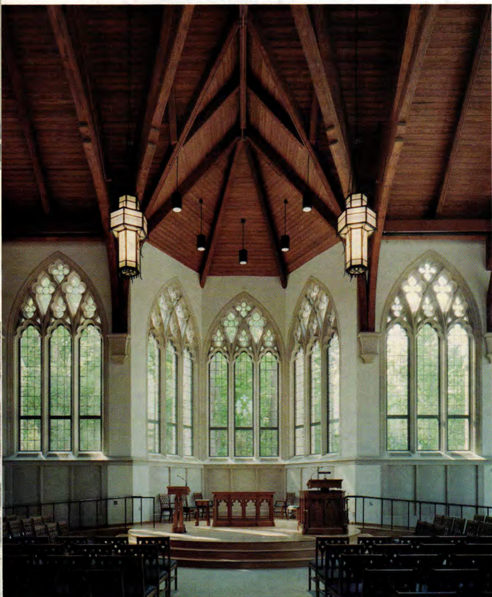
Goodson Chapel features 55-ft.-tall heavy-timber ceilings, an architectural-grade southern-pine ceiling deck and rustic-buff Indiana limestone trim and detailing. The window tracery is Hartman-Cox Architects’ own design; it was inspired by Duke Chapel’s window trim.
