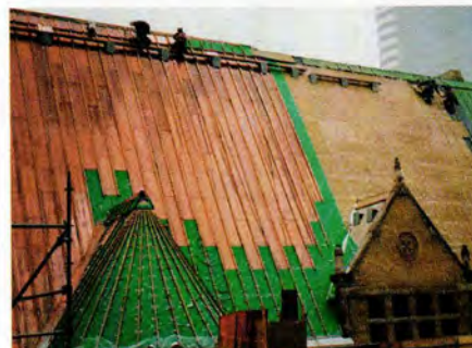
Heather & Little's restoration of the Toronto Old City Hall required 113,900-sq.ft. of copper roofing, cornices, gutters and sheet-lead work.
