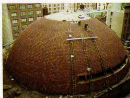
The dome of the New York City Center was originally completed in Ludowici Roof Tile in 1923; it was restored with roof tile from the same company in 2004.
