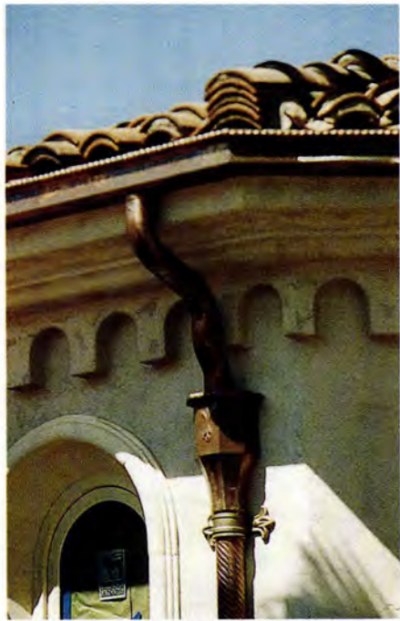
Hans Liebscher Custom Copperworks & Sheet Metal fabricated this ornamental gutter, smooth downspout gooseneck leader head and twisted downspout.
