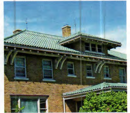
Tile Roofs provided the matching green salvaged Spanish tile and fittings for the restoration of this clay tile roof.
