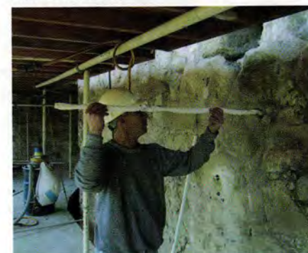
The Cintec Reinforcing Anchor System is a micro cement anchoring and reinforcing system used for the repair and renovation of existing masonry buildings.
