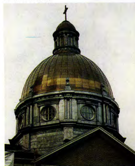
Heather & Little restored the lead-coated-copper dome and cupola for Our Lady of Lourdes Roman Catholic Church in Toronto, Canada.
