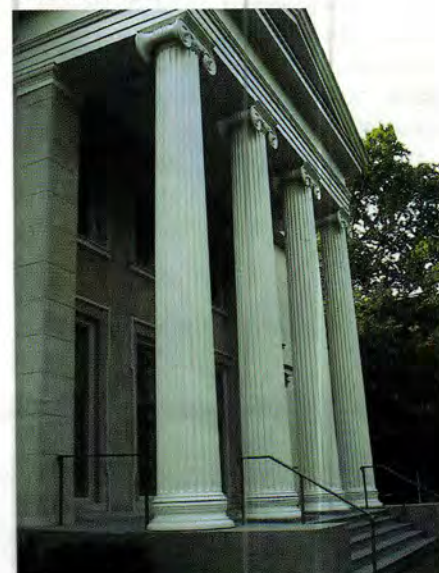
Fagan Design replicated this 30-in.-dia. x 20-ft.-tall fluted column (foreground) to match existing columns.
