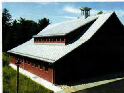
Yale University's Lewis Walpole Library in Farmington, CT, has a roof made of Follansbee's TCS II terne-coated stainless steel with a gray patina.
