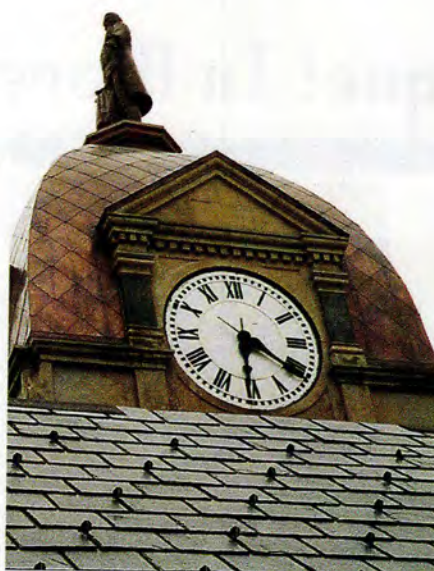
The clock tower of the Hancock County Courthouse in Findlay, OH, was sheathed in new copper by NIKO; the firm also replaced the slate roof as part of the complete restoration.
