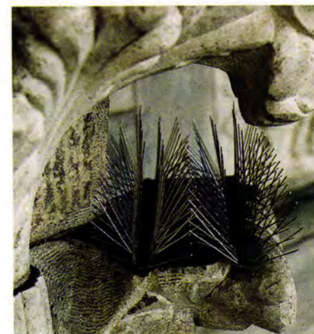
The South Australian Parliament Building used adhesive spikes from Nixalite beneath wide cornice and pediment overhangs.
