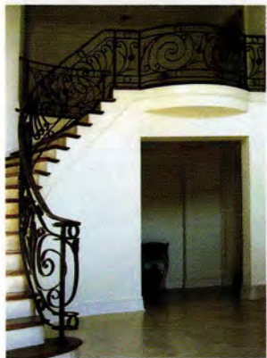
New Star Brass & Bronze Works custom fabricated this decorative iron railing with a hand-forged bronze top rail.
