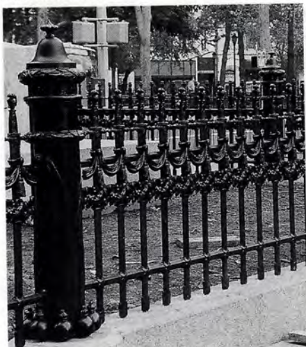
This wrought- and cast-iron entry gate was restored by Architectural Iron Co.
