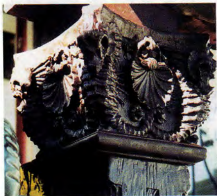
De Groot Historical Restoration restored this white-oak capital from an exterior staircase leading to the bell tower and William Vanderbilt's third bedroom at the Vanderbilt Museum in Centerport, NY.
