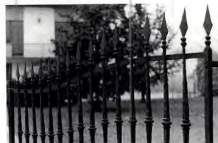
This fence is constructed of tapered pickets that were forged by King Architectural Metals.
