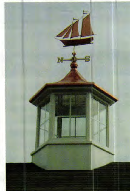
Designed to be maintenance free, cupolas from New Concept Louvers are wrapped with PVC-coated aluminum.
