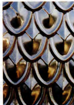
These roof shingles were fabricated by Hans Liebscher in 20-oz. copper.
