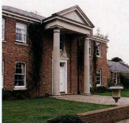
Haddonstone's cast-stone M1 columns were used with Doric capitals to create the Classical entryway for this building.
