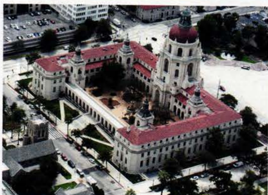
Right: Pasadena's multi-domed City Hall has undergone a $117.5 million restoration, including subterranean seismic reinforcements and a steel-reinforced concrete arcade (left) replacing a quake-vulnerable terra-cotta original.
