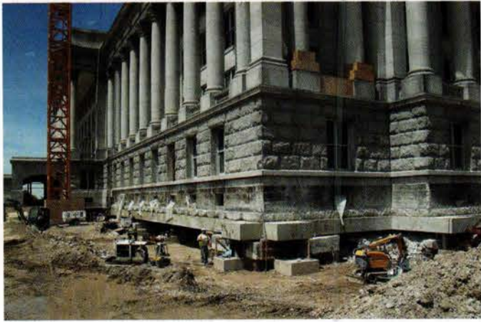
The foundation of the capitol building was removed so that 265 base isolators weighing 5,000 lbs. each could be installed. During that time, temporary jacks supported the building. Photo: Robert Loversidge, Jr., Schooley Caldwell Associates
