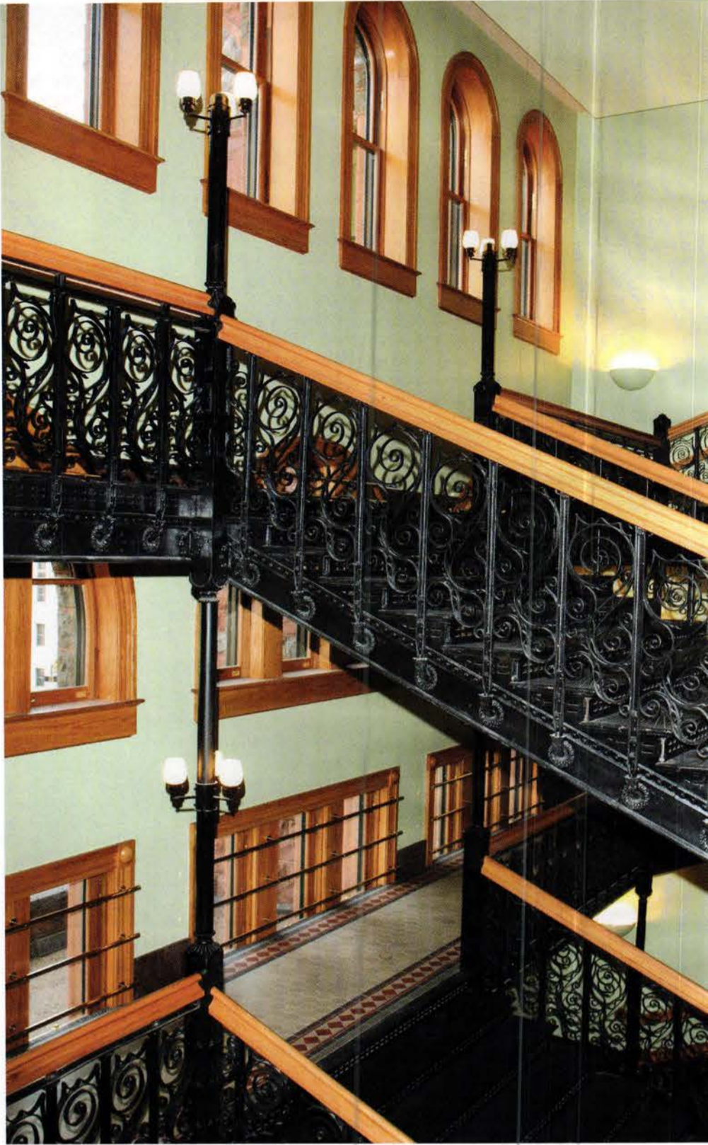
Based on staircase ghosts found throughout the courthouse atrium, Robinson Iron of Alexander City, AL, created a curlicued multi-switchback replica.
