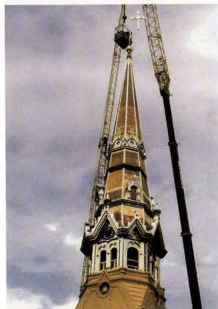
Heather & Little fabricated the new 115-ft.-tall, 60,000-lb. spire, which incorporates more than 2,000 sq.-ft. of hand-pressed copper shingles, for the historic St. Raphael Cathedral in Madison, WI.
