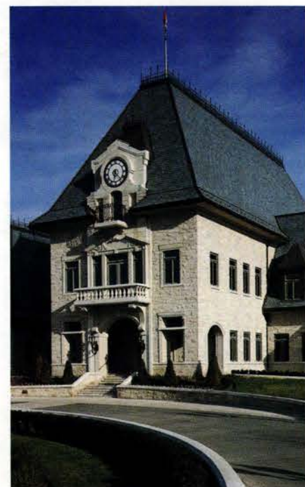
Casemaster aluminum-clad casement windows with green-tinted glass from Marvin Windows & Doors were used for the Magna International headquarters building in Aurora, Ontario, Canada.
