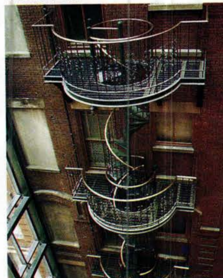
Stairways designed and manufactured this 55-ft.-tall spiral staircase with a bronze handrail.
