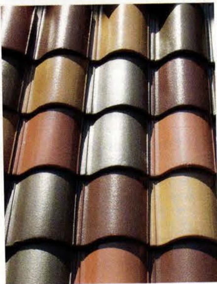
When replacing the terra-cotta roof of the Breakers Mansion in Newport, RI, Boston Valley Terra Cotta used 35,000 field tile and approximately 4,000 special-shaped fittings.
