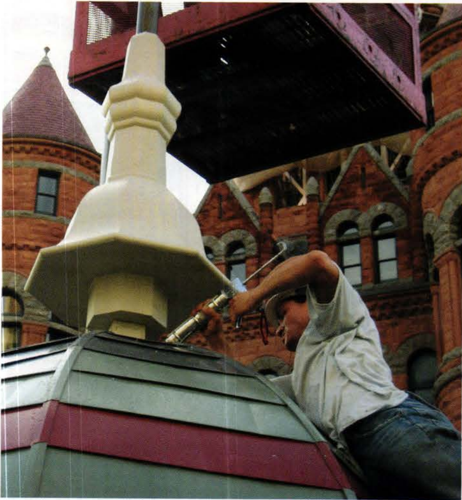
The aluminum and steel cupola, by Campbellsville Industries of Campbellsville, KY, is roofed in overlapping stripes that emulate the original slate.
