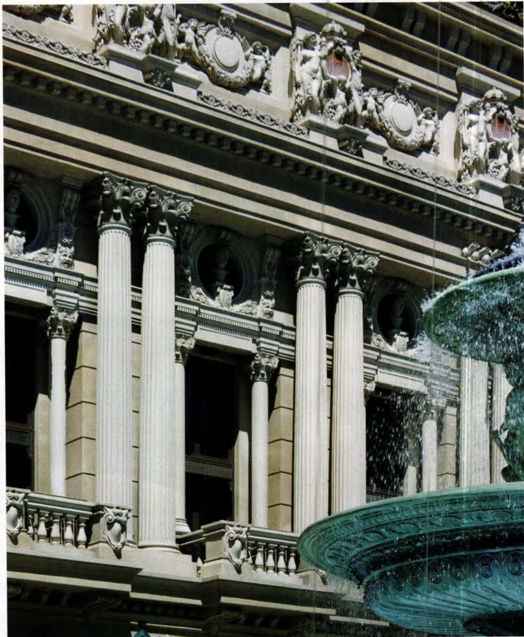
To simulate limestone for the facade of Caesar's Palace in Las Vegas, NV, Melton Classics, Inc., created these elaborately textured GFRC columns, along with the FRP cornice and cast-stone balustrade. Photo: courtesy of Melton Classics
