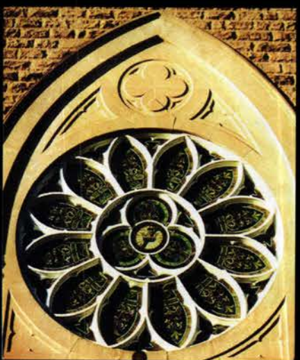
Above: First United Methodist Church, Iowa City, Iowa. Rose window with Bovard Studio's aluminum Precision Flow® framing system bent to match the original historic Rose window frame.
