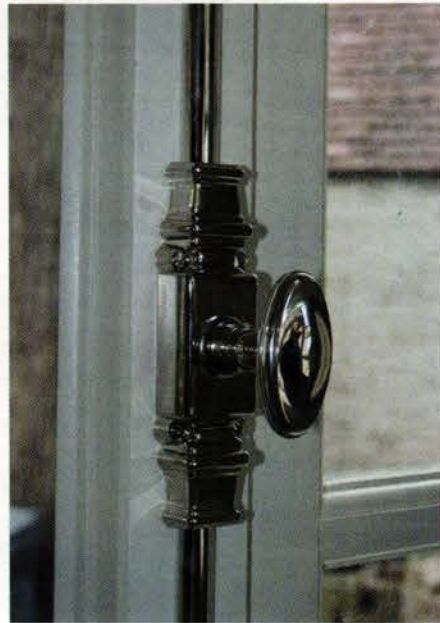
Al Bar-Wilmette installed this un-lacquered silver cremone set for a client on Lake Michigan.
