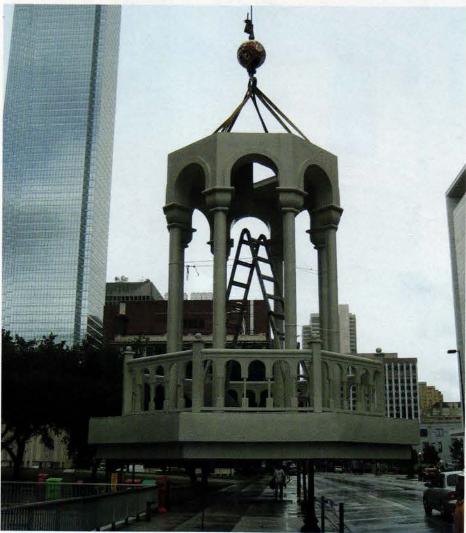
Below: A crane hoisted Campbellsville’s balustraded, domed cupola to the tower peak.
