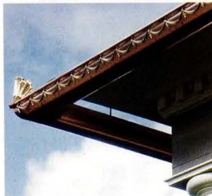
Classic Gutter Systems fashioned this elaborate half-round copper gutter with gold-patinated solid-brass trim and a rain deflector.
