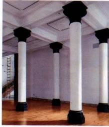
The old-growth heart pine flooring was re-milled by Goodwin Heart Pine and installed in this building in Key West, FL, to match the existing flooring.
