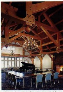
A hammer-beam timber frame dominates the Mozart Room, the main conference room of the Trappe Family Lodge in Stowe, VT, erected by Vermont Timber Works.
