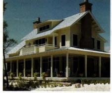
FiberCement siding from CertainTeed is made of recycled fly ash, Portland cement, wood fiber and
