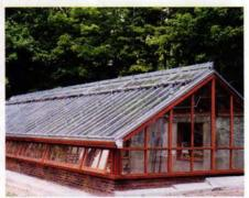
Glass House, LLC reconstructed this greenhouse that has been converted into an architectural studio; it features mahogany framing, ganged roof and side vents for ventilation, refitted with the actual chain pulley operators with copper exterior roof cappings.
