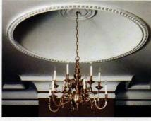
Goodwin Associates supplied the fiberglass dome and polyurethane moldings for this ceiling.
