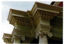
Seal Reinforced Fiberglass used fiberglass to replicate the complex architectural elements on this building.
