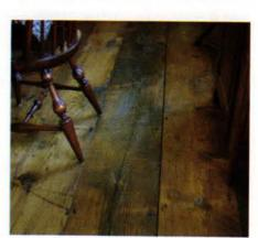
Reclaimed, hand-planed antique chestnut flooring supplied by Old Wood Workshop is available in widths from 9 to 14 in.
