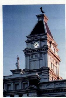
Campbellsville Industries fabricated the clock tower, clock, decorative cornice, modillions, paneled railing and corner pediments for the restoration project at Montgomery County Courthouse in Clarksville, TN.
