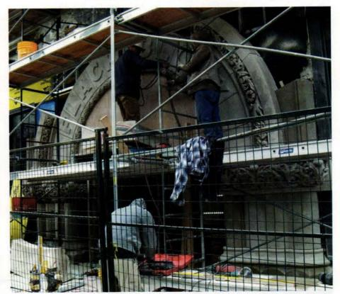
Above: The building's seismic upgrade required that the new ornamental stonework be clad around a steel frame, which entailed some complex anchoring details. As a result, the re-created entry for the Flack Block was installed not by ASM's own team but by the masonry-restoration contracting firm of Atlantis Rausch Granite & Marble Installations, Ltd.
