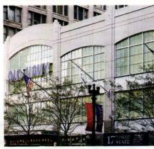
The glass fiber reinforced concrete (GFRC) used to re-clad this building on State Street in Chicago, IL, was acquired from Ball Consulting.
