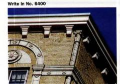
Architectural Fiberglass Corp. replicated the cornices on this New York City apartment building in fiberglass-reinforced polymer.
