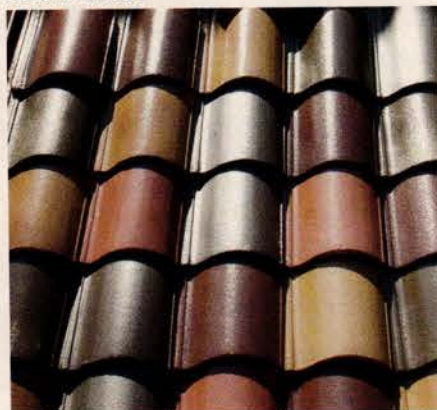
When replacing the terra-cotta roof of the Breakers Mansion in Newport, RI, Boston Valley Terra Cotta used 35,000 field tile and approximately 4,000 special-shaped fittings.
