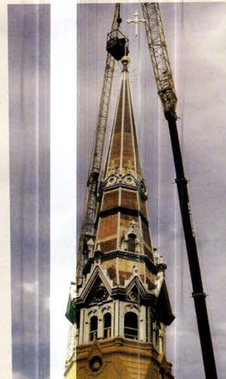
Heather & Little fabricated the new 115-ft.-tall, 60,000-lb. spire, which incorporates more than 2,000 sq.ft. of hand-pressed copper shingles, for the historic St. Raphael Cathedral in Madison, WI.
