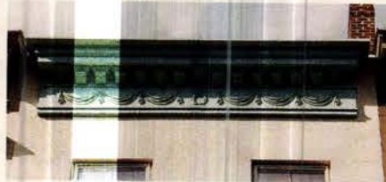
Seal Reinforced Fiberglass provided an FRP replication of the original metal cornice for this New York City building.
