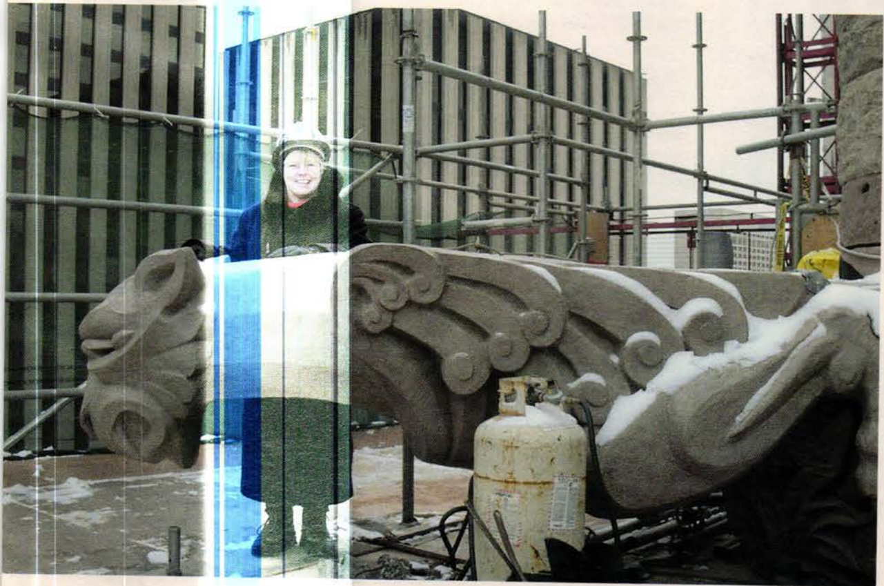
The design of the clock tower's original gargoyles was unusual in that the statues were horizontal and cantilevered out from the clock tower about 9 ft. at its corners. Carved in sandstone, their own weight inevitably resulted in dangerous crumbling, and so they all had been removed. The replacements were cast in bronze at the end of 2002: an innovation that significantly reduced their weight. An artificial-patina solution, mixed with sifted-sand mortar, was applied to give the metal the color and texture of stone.
