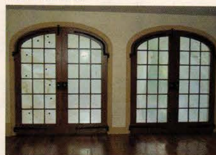
These elliptical arched-top French doors with double pane insulated glass were fabricated by Illingworth Millwork.
