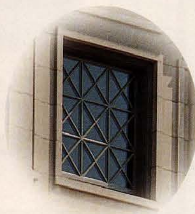
The 3-by-3 diamond lite cut is uncommon; Marvin's Simulated Divided Lite with spacer bar solution is equally unique.
