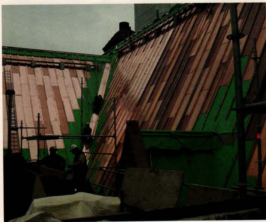
Laying a new copper roof for Old City Hall involved the removal of the old roofing, the addition of a new surface of 1½-in. plywood over the existing wood deck, a layer of peel-and-stick membrane plus insulation spaced with wooden sleepers, and ¾-in. V-tongue-&-groove plywood covered with Roofshield: a flexible acrylic underlay system popular in Europe but still fairly new in North American applications.
