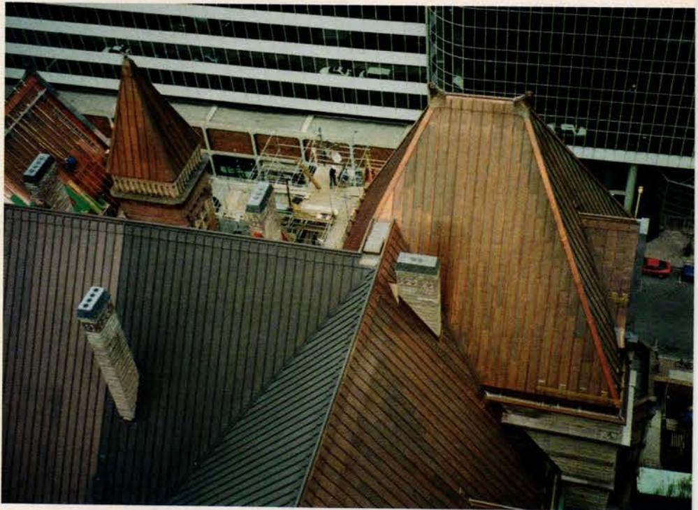
Above: Workers from Heather & Little Limited of Markham, ON, relied on bosun chairs, attached to rope falls, to lay almost four acres of copper sheet in a batten-seam pattern for the new roof of Toronto's Old City Hall. The roof's vast size and its complex details – including snow guards, dormers and finials – complicated the painstaking effort. In all, some 66 tons of 20-oz. sheet copper and 20 tons of sheet lead were used to cover the 173,600 sq.ft. roof.
