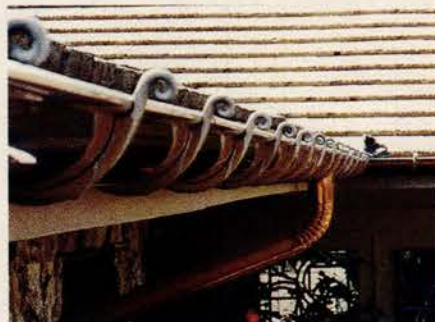
This decorative 6-in. half-round gutter from Classic Gutter Systems is made of 20-oz. copper and heavy-duty aluminum.
