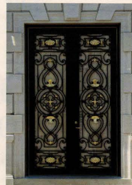
These forged-steel entry doors from Schwartz's Forge & Metalworks have 23k gold-leaf details.
