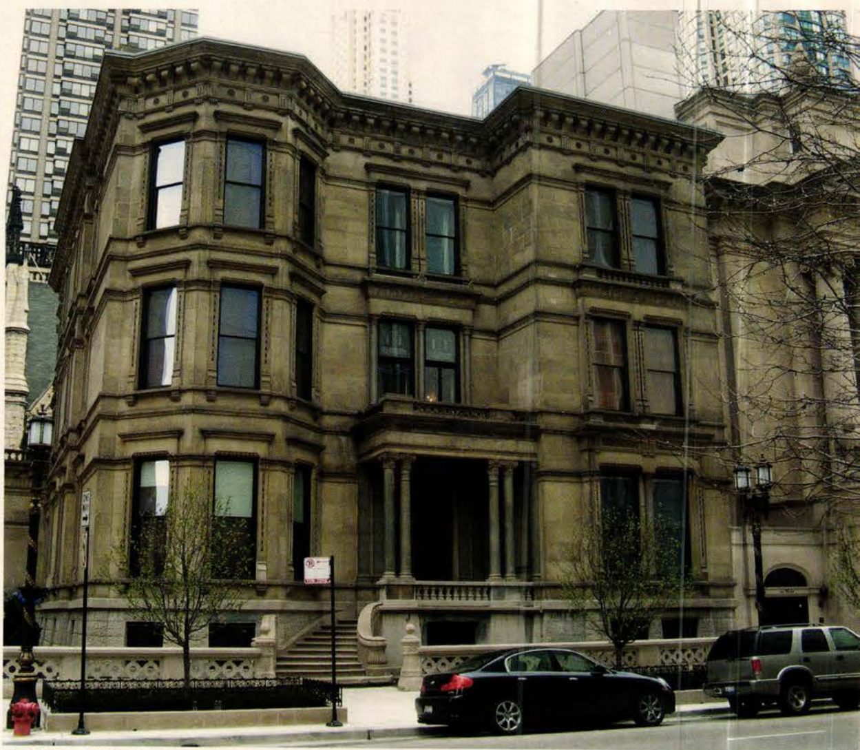
The Nickerson Mansion-turned-Richard H. Driehaus Museum is the first American building to be wholly cleaned by lasers; soot had covered the sandstone and limestone for so many decades that most Chicagoans assumed that the original stone was black. Photo: courtesy of the Richard H. Driehaus Museum
