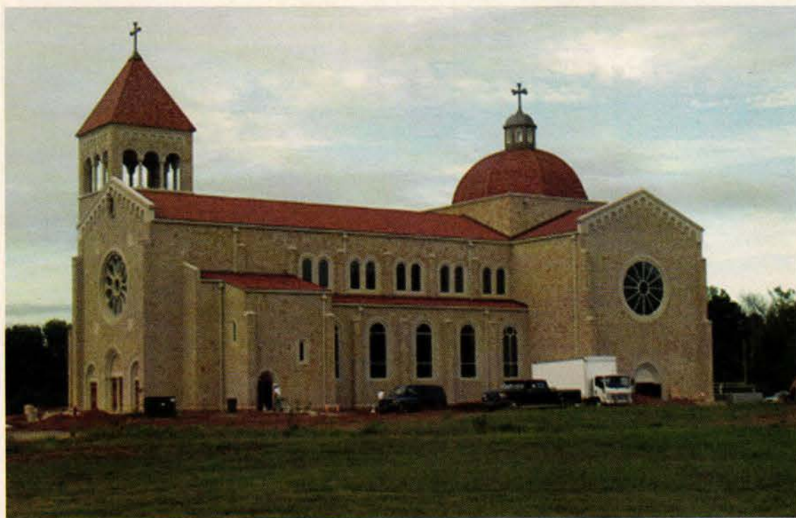
The openings of the church were intentionally designed to be small in proportion to the mass of the building – a characteristic of the Romanesque style.
