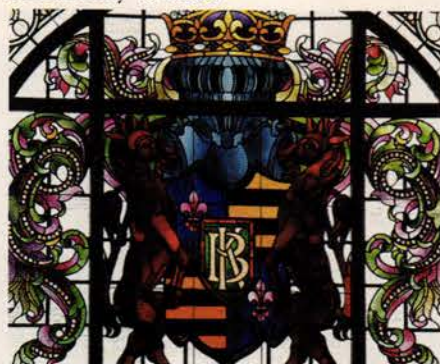
This detail of a window in the Chicago Theatre illustrates the film strips, reels and monogram of the theater entrepreneurs Balaban & Katz; when restoring it, Restoric was able to preserve more than 90 percent of the original glass and lead came.
