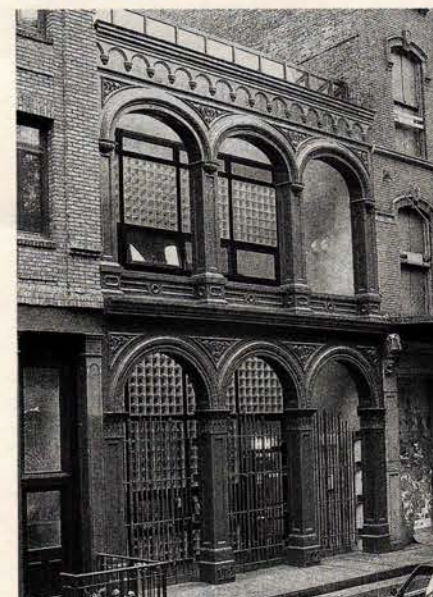
Historical Arts & Casting restored and re-installed the cast-iron windows of this building in New York City.
