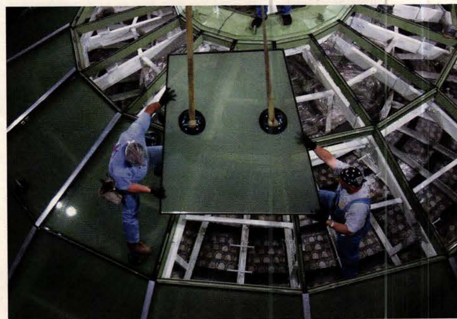
Insulated glass units weighing several hundred pounds were set with a crane. Photo: Elizabeth Blaisius
