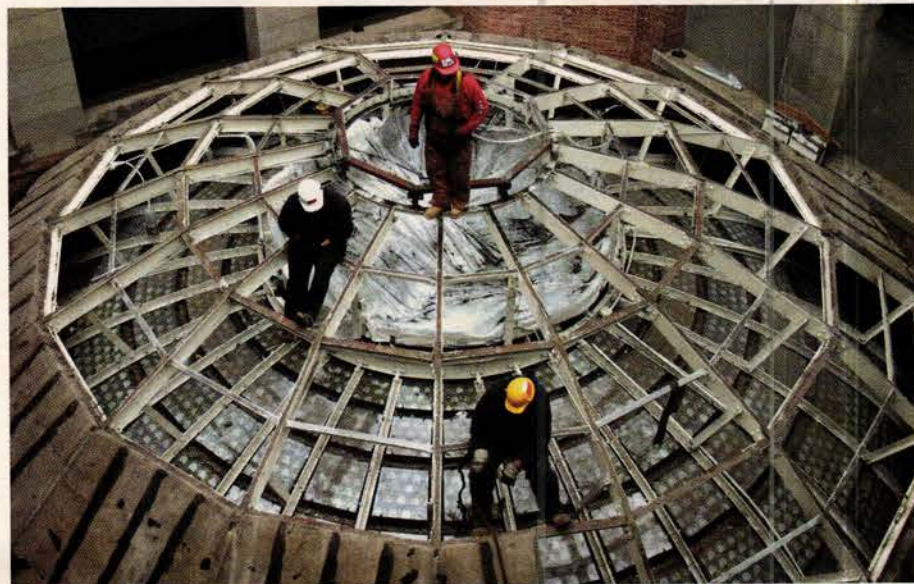
The precast concrete installed in 1935 is removed from the original 1897 steel frame; what appears to be art glass below the workers is actually a graphic reproduction on Lexan. Photo: Neal A. Vogel, Restoric, LLC
