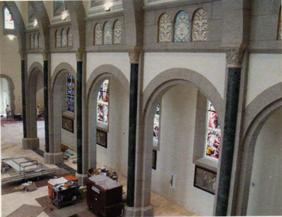
Instead of wrapping the entire pier with marble, half columns of marble were added to the side facing the nave.
