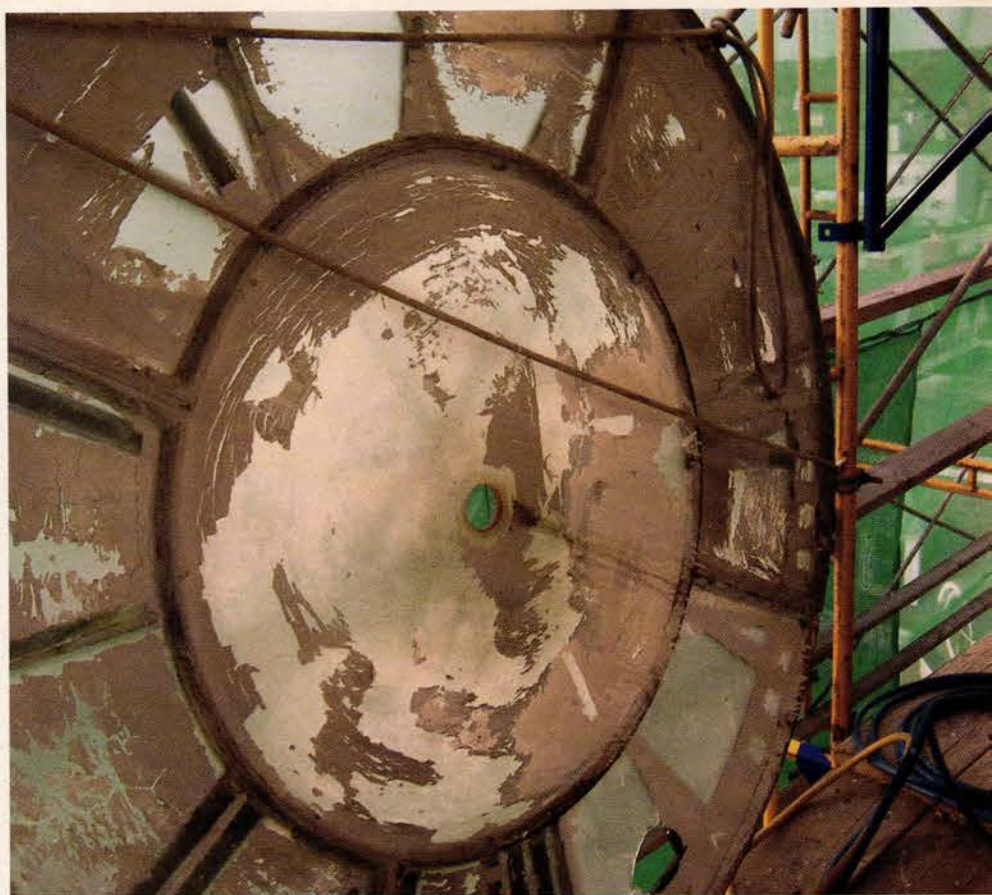
Above: The 1893 clock faces were clogged with paint. Photo: David Baer, Milestone Engineering & Construction
