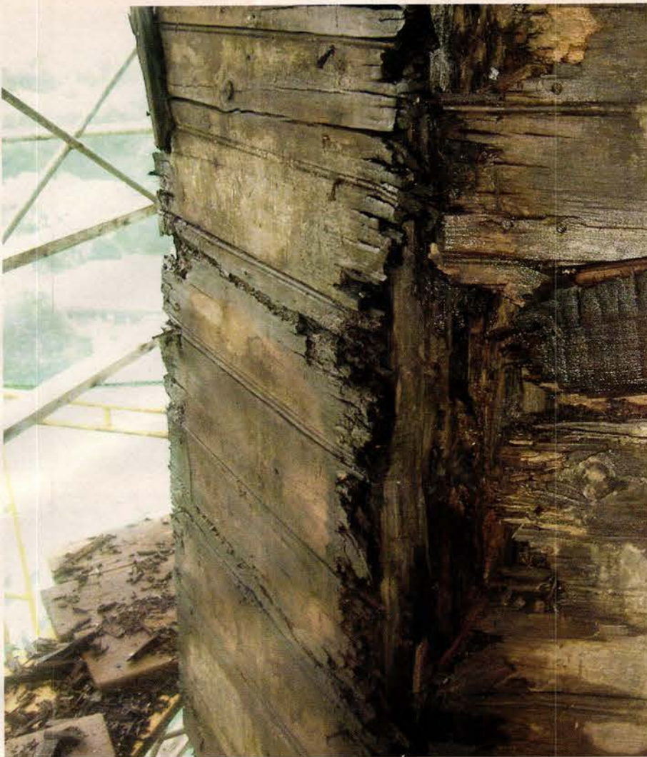
Water damage had caused deep rot in the steeple timbers and sheathing. Photo: David Baer, Milestone Engineering & Construction
