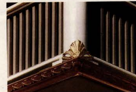
This ornate gutter, fabricated by Classic Gutter Systems, incorporates a hidden adjustable hanger system.
