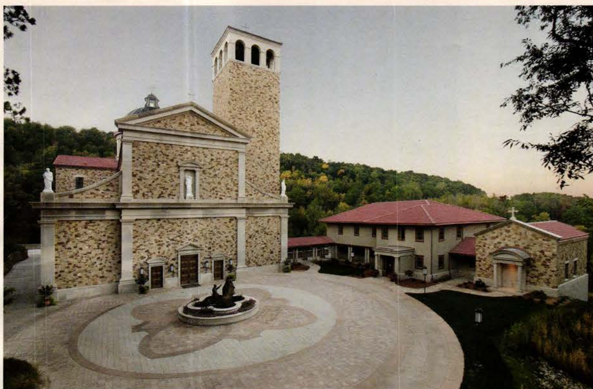
The church building is part of a complex of buildings in the hills outside of La Crosse, WI. The exterior was designed to look like a simple Tuscan building. Stone from Minnesota and Wisconsin was blended to create the colorful appearance, while gray limestone was used for the cut details. Bob Metcalf Commercial Photography, La Crosse, WI
