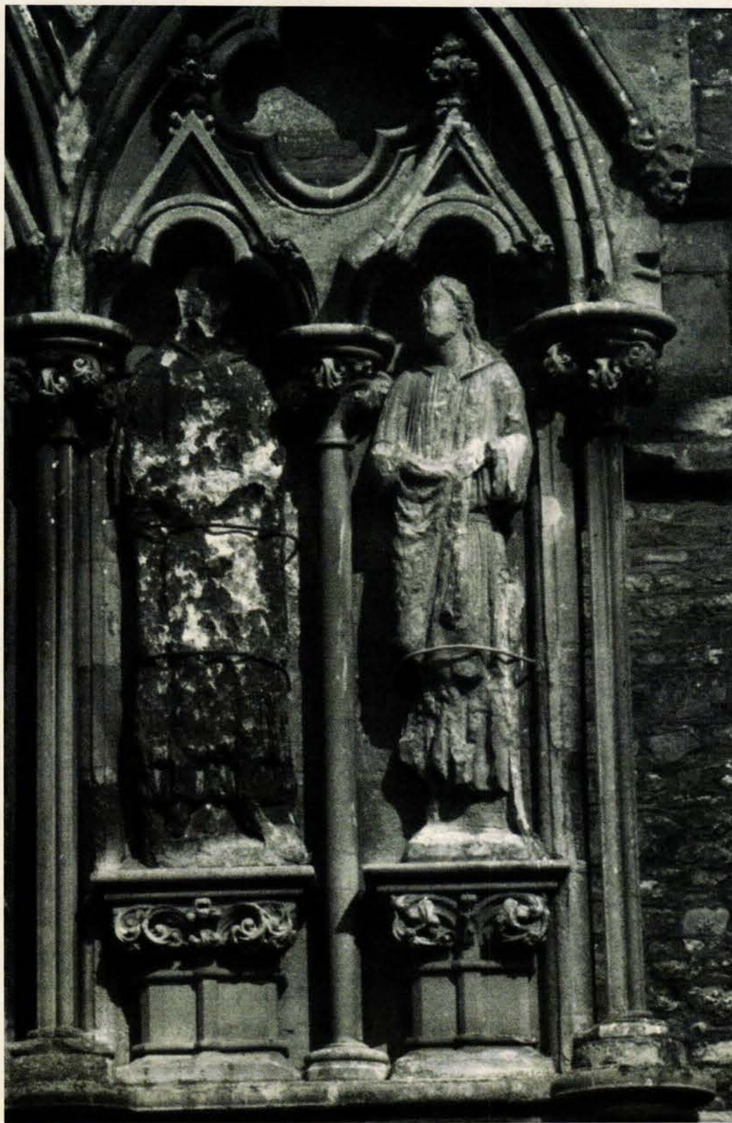
At Wells Cathedral in Somerset, England, the stone figure on the right was consolidated with lime solution to good effect.
