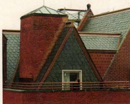
Nicholson & Galloway restored the roof of this historic building, providing the carpentry, coppersmithing, slating, waterproofing and masonry restoration.
