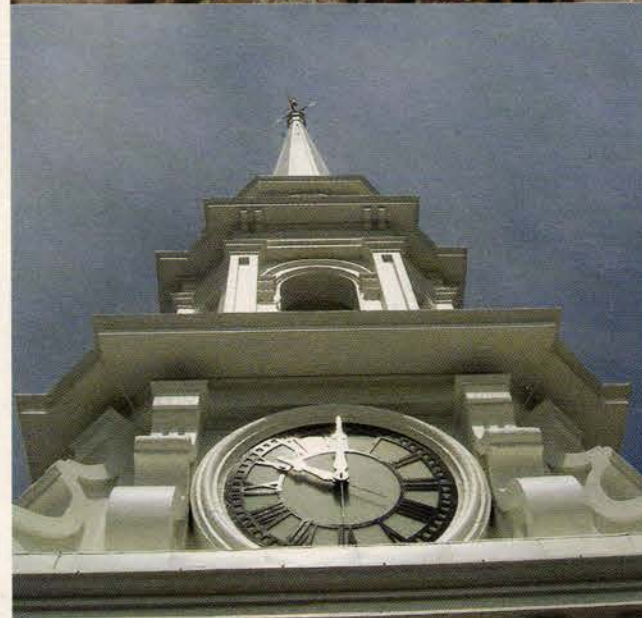
Above: The 1893 clock faces were clogged with paint. Photo: David Baer, Milestone Engineering & Construction
