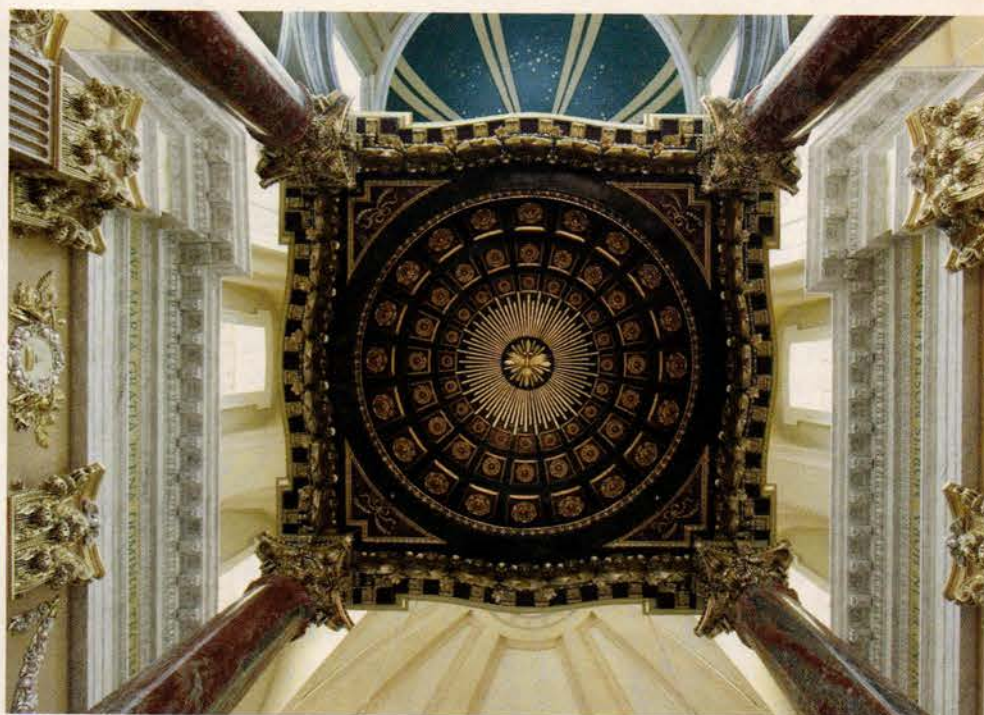
Inspired by Santa Maria Maggiore in Rome, the marble baldacchino features a coffered dome, delicately curved cornice and an intricate angel valence. This view shows the baldacchino's plaster ceiling with its faux marble and gilded finish. Photo: Bob Metcalf Commercial Photography, La Crosse, WI
