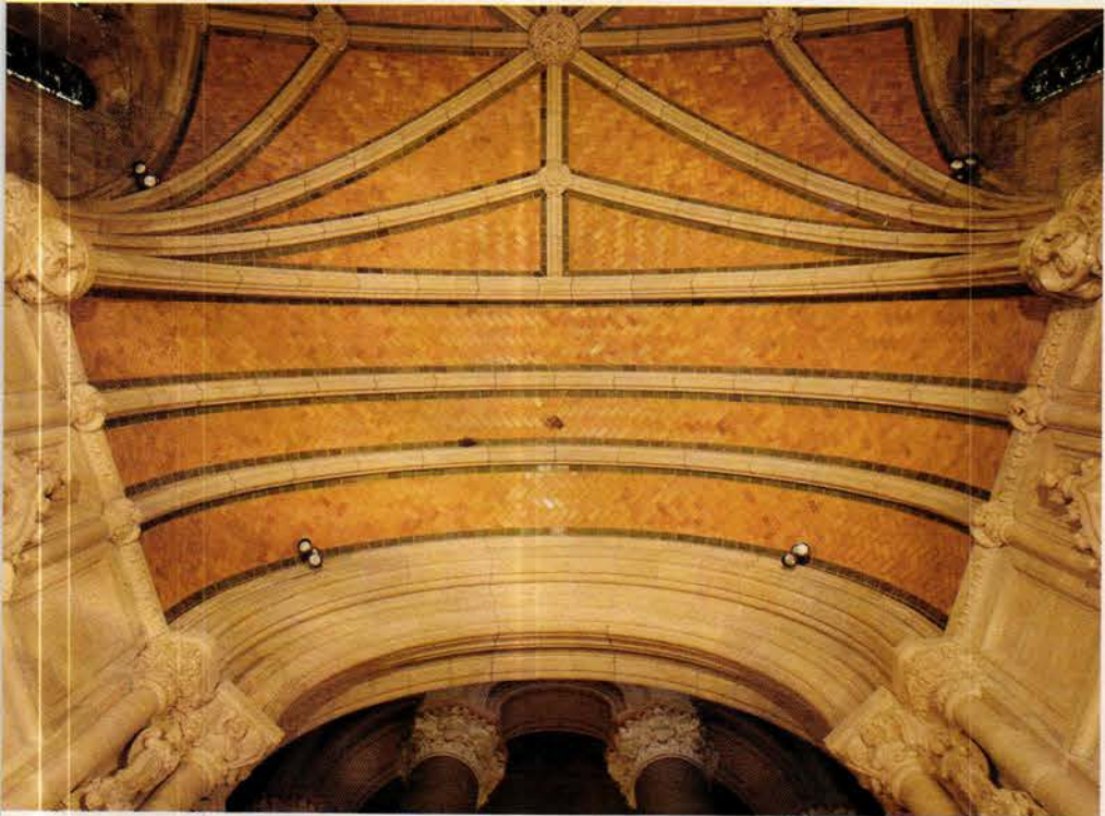
Most of the cathedral vaults are lined in lightweight interlocking tiles manufactured by the Guastavino Fireproof Construction Company. Photo: T. Whitney Cox
