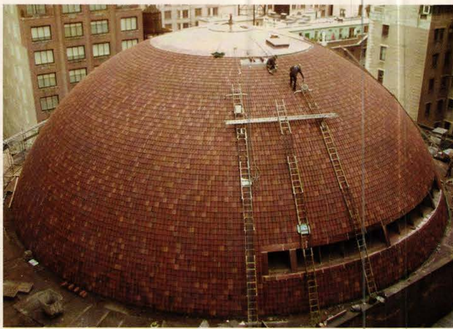
The dome of the New York City Center was originally finished in Ludowici Roof Tile in 1923; it was restored with roof tile from the same company in 2004. Key in no. 2760
