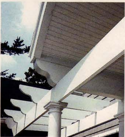
This custom pergola from Goodwin Associates uses girders and cross rafters of reinforced board that is maintenance-free and rot-resistant. Key in no. 806
