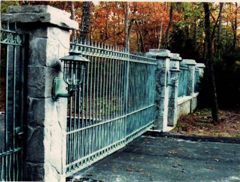
Fine Architectural Metalsmiths fabricated this country estate gate and matching fencing, with miter-forged terminals on broken-edge pickets, traditional lower picket line and circle frieze in a verde gris patina. Key in no. 2640
