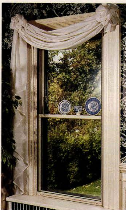
Innerglass Window Systems created this custom interior storm window, which is designed to eliminate drafts and reduce sound infiltration. Key in no. 909
