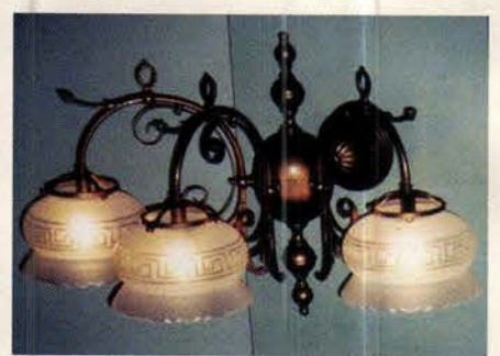
The original 19th-century gas wall sconces at the Georgia State Capitol in Atlanta were retrofit with glass fiber-optics functional architectural lighting by Conservation Lighting .
