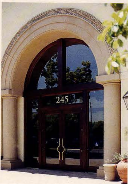
This precast arched entry surround to the Lytton Building in Palo Alto, CA, was fabricated by Architectural Facades Unlimited . Key in no. 1470
