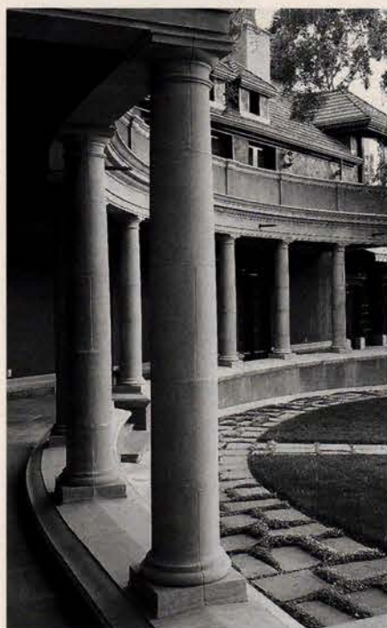
These precast GFR columns and capitals in this curved colonnade were manufactured by Architectural Facades Unlimited . Key in no. 1470
