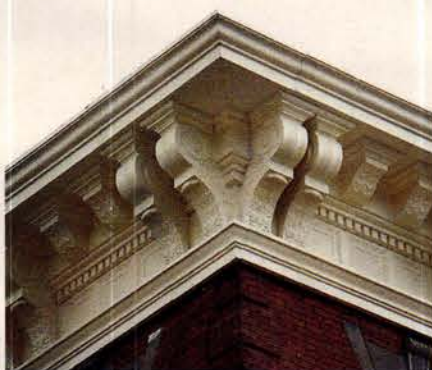
Architectural Fiberglass Corp. fabricated this 61-in.-tall cornice with a 30-in. projection for a restoration project in the Bronx, NY. Key in No. 6400
