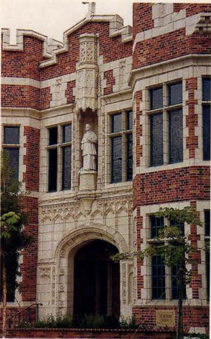
A&M Victorian Decorations cast new concrete ornamentation for the renovation of the Loretto-Conaty High School in Los Angeles, CA. Call for more information.
