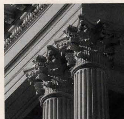
DeAngelis Iron Work, Inc. supplied and installed 12 cast-iron capitals for the exterior restoration of the Massachusetts State House. Key in no. 1023
