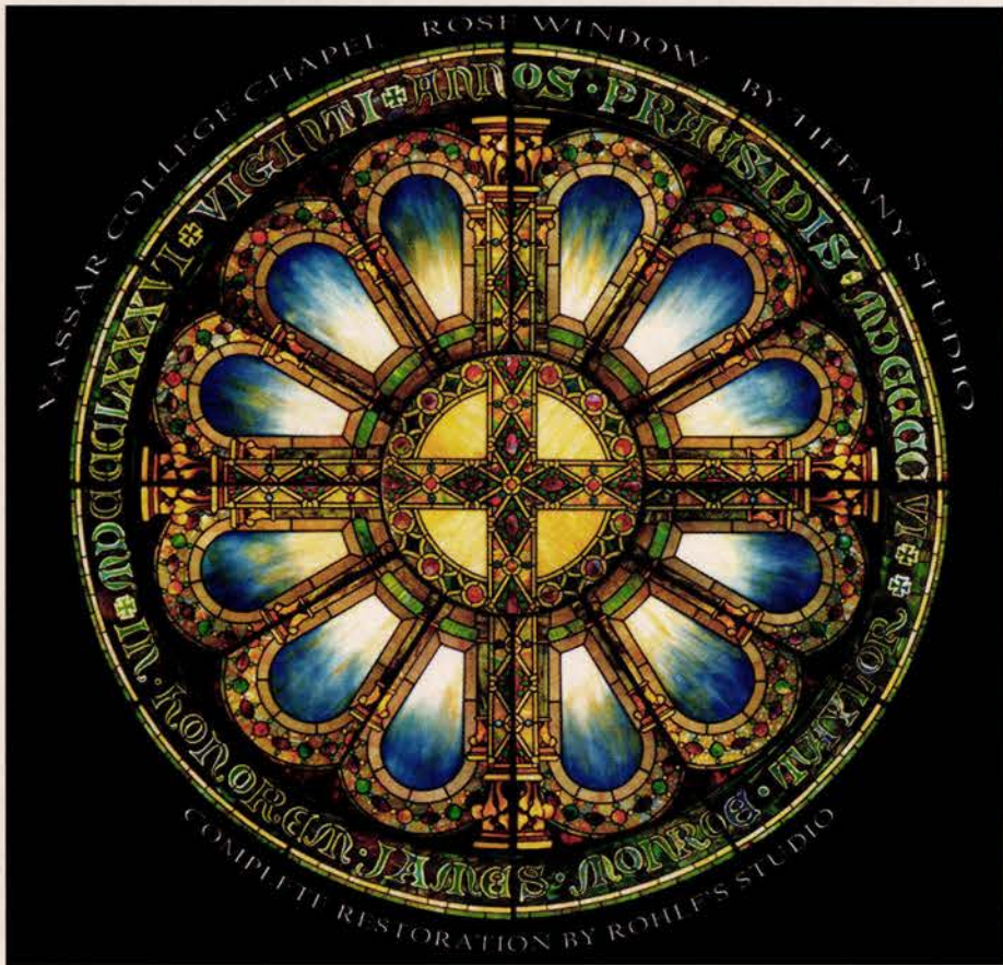
The Tiffany Rose Window at the Vassar College Chapel in Poughkeepsie, NY, was removed, re-leaded and re-installed by Rohlf's Stained & Leaded Glass Studio ; the firm also retrofitted the double-glazed steel frame system. Key in no. 1480
