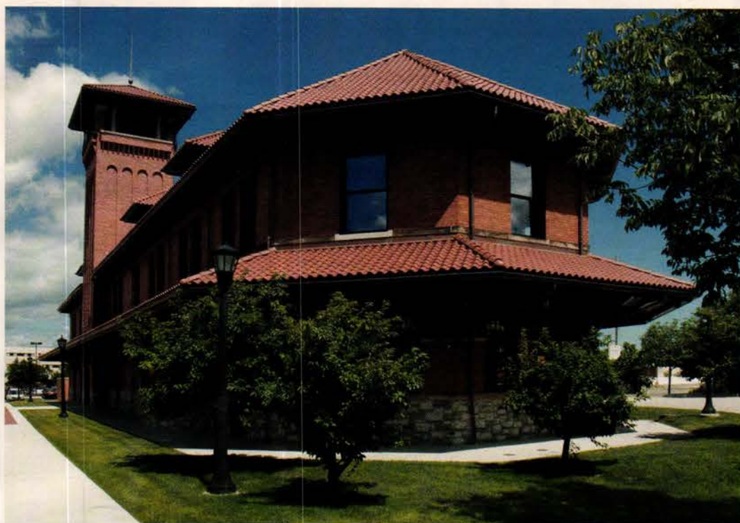
QUINN EVANS | ARCHITECTS rehabilitated the Pere Marquette Depot in Bay City, MI, after it had been abused and vacant for more than 50 years. Instead of going to the landfill, the extant brick walls, heavy timber attic framing, second floor original offices and almost all of the original windows and doors were saved, repaired and reused.
