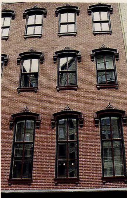
These double-hung windows were custom designed by Parrett Windows and installed with weight-and-pulley sash and balance systems. Key in no. 3003
