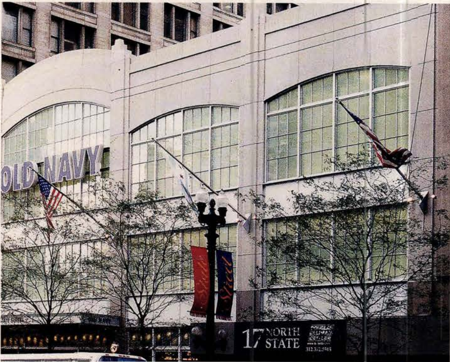
The glass-fiber-reinforced concrete (GFRG) used to re-clad this building on State Street in Chicago, IL, was supplied by Ball Consulting . Key in no. 7260
