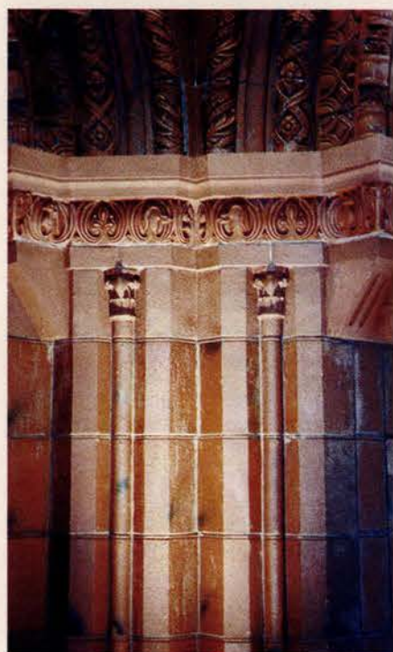
Boston Valley Terra Cotta custom fabricated the terra-cotta moldings and trim in this church. Key in no. 160
