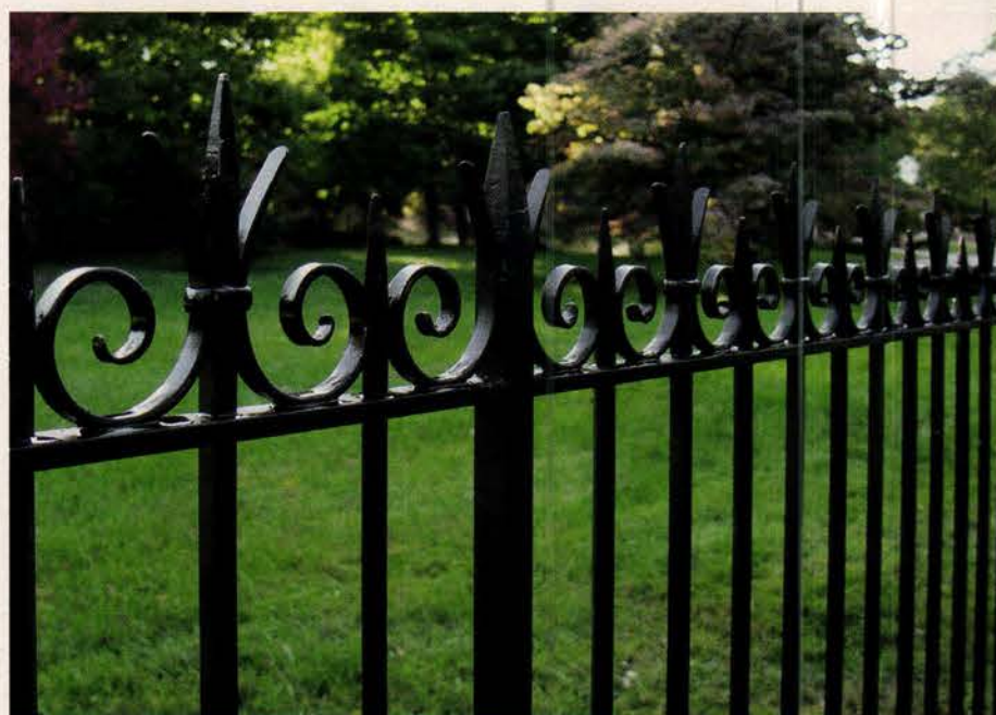
This custom fence was designed and fabricated by Wiemann Ironworks using solid-bar steel; to ensure longevity, it was galvanized before urethane coating was applied. Key in no. 1223
