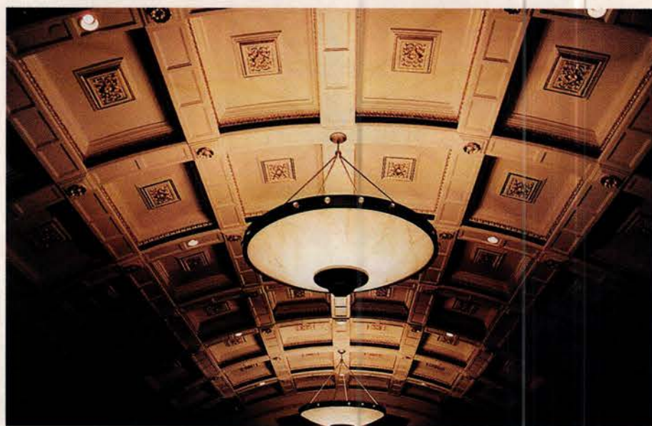
Flex Moulding used polyester resin to create this ornate barrel-vaulted ceiling. Key in no. 4900
