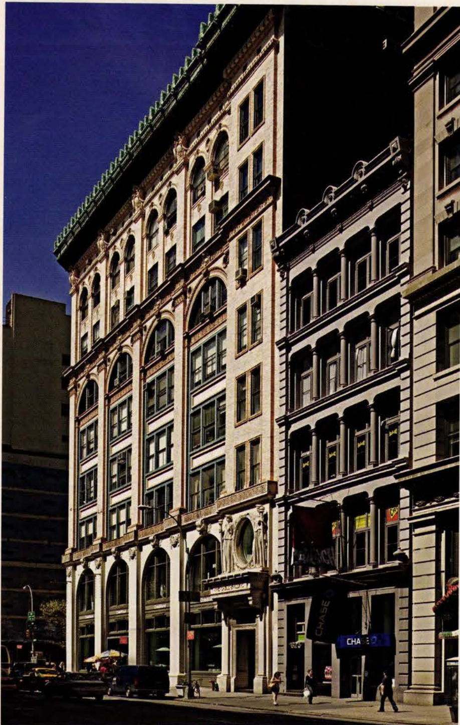
On the 1894 Cable Building in Manhattan, stringcourses delineate the base, piano nobile and attic. Terra-cotta ornament and a massive copper cornice project from the yellow-brick façade.
