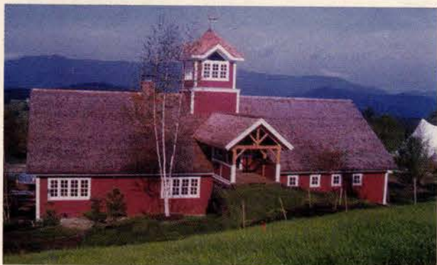
This 1½-story 20x36 ft. post-and-beam barn was built with a kit from Country Carpenters ; it features a 10x36-ft. lean-to. Key in no. 1439
