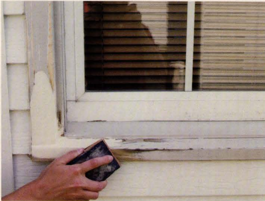
Abatron's LiquidWood restoration system regenerates and waterproofs dried-out or spongy wood. Key in no. 1300
