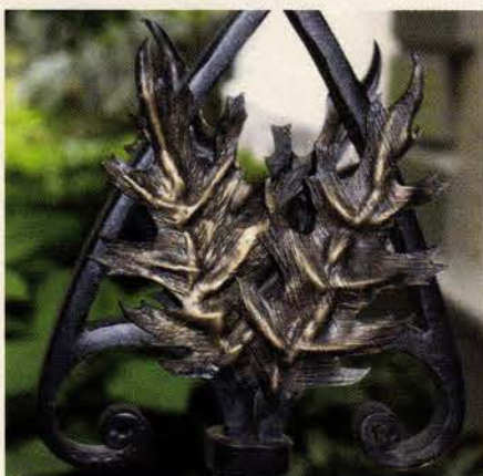
Fine Architectural Metalsmiths used mixed metals to create a cluster of repoussé oak leaves in this grillework. Key in no. 2640
