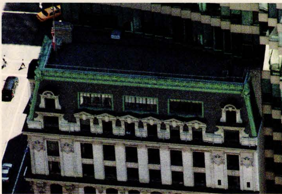
Nicholson & Galloway restored the slate roof, copper cornice and brick and limestone façade of this building. Key in no. 3067
