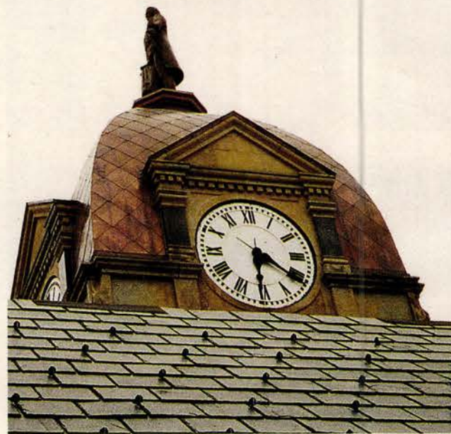
NIKO Contracting Co. replaced the slate roof and sheathed the clock-tower dome in copper on the Hancock County Courthouse in Findlay, OH. Key in no. 8300
