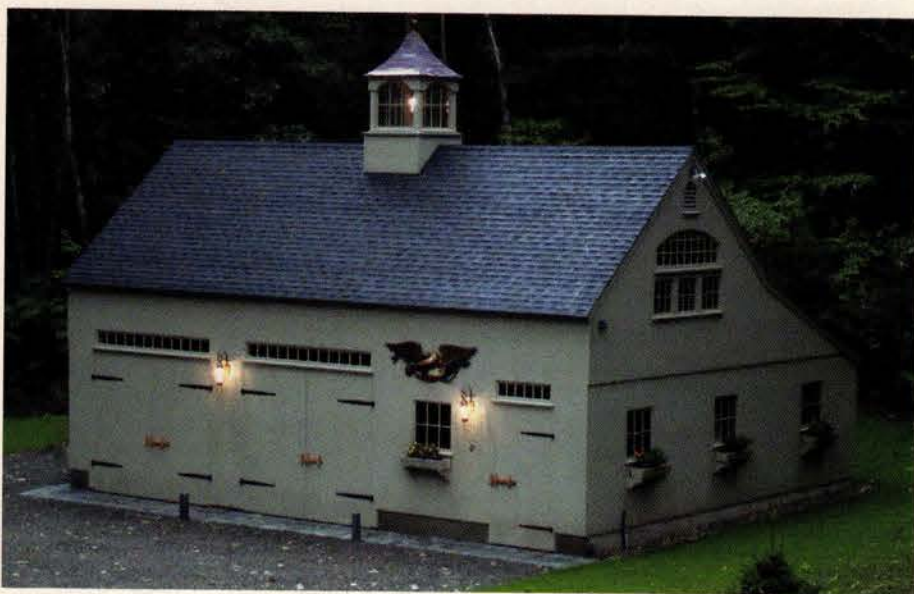
This 1½-story 20x36 ft. post-and-beam barn was built with a kit from Country Carpenters ; it features a 10x36-ft. lean-to. Key in no. 1439
