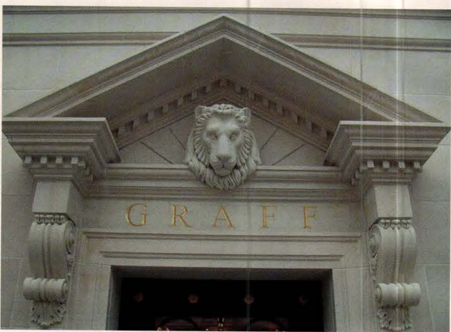
The exterior ornament on this Palm Beach, CA, building was fabricated in French limestone by Traditional Cut Stone . Key in no. 2902
