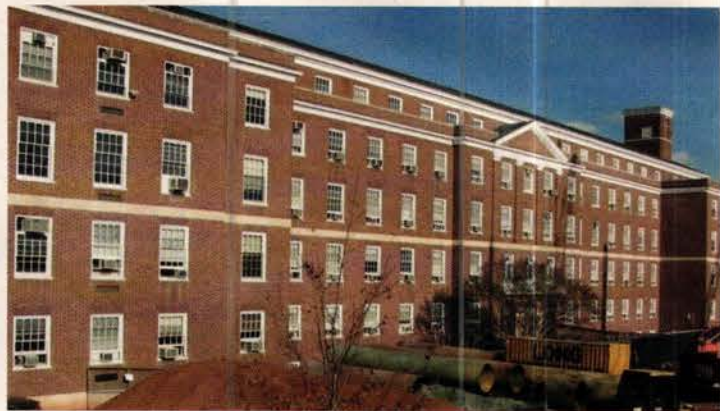
Below: Goody Clancy is renovating this 50-year-old, five-story, 159,129-sq.ft. building, New Cabell Hall, at the University of Virginia. Although the character of the building is considered uninspiring, the university recognized that it is more cost-effective to renovate than to replace it. The renovation will address systems improvements such as replacing heating and adding central air conditioning, and will update interior finishes and classrooms and create a new lobby.
