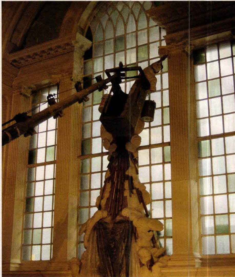
John Tiedemann used a boom system when restoring the interior of St. Paul's Chapel in New York City. Key in no. 1765
