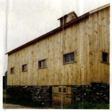
South County Post & Beam built this 56x32-ft. timber-frame barn on the existing stone foundation of a building that had been demolished.
