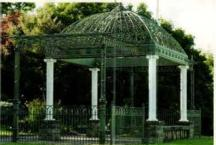
Wiemann Ironworks fabricated this gazebo, fence and trellis in cast and wrought iron.
