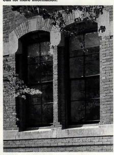
Architectural Components manufactured these custom windows with true-divided lites and insulated restoration glass for Weld Hall at Harvard University.
