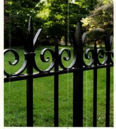
This custom fence was designed and fabricated by Wiemann Ironworks using solid-bar steel; to ensure longevity, it was galvanized before urethane coating was applied.
