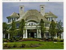
A Cedar Shake & Shingle Bureau member provided the cedar roofing for this building; the shakes are lightweight and have a high insulation value.
