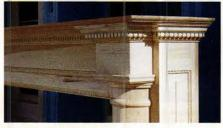
The Wood Factory used stile-and-rail construction to fabricate this pecan mantel.
