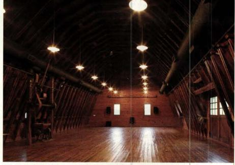
The wood interior of the assembly hall, in the loft of the Main Barn, has been rigorously cleaned and sealed with a preserver. Structural insulated panels, from Shenandoah Junction, WV-based PanelWright, were installed in the roof. The finishes were left in their original colors and the existing pulleys were also left intact.
