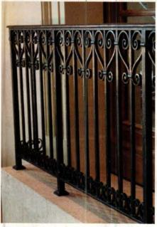
Wiemann Ironworks designed and fabricated this custom hand-forged iron railing.
