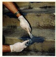
Abatron's Abocrete restoration epoxies can be used to patch various surfaces.
