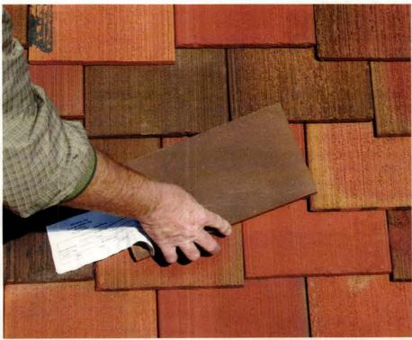
The custom-designed clay tiles on the original clubhouse building were manufactured by B. Mifflin Hood Tile Company, which went out of business in the 1950s. In order to replicate the roof, New Lexington, OH-based Ludowici Roof Tile was brought on board. Ludowici's first step was to color match the glazing.
