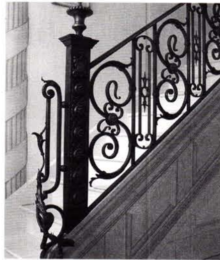
This custom-forged, cast-bronze and -iron stair railing was fabricated by Wiemann Ironworks.
