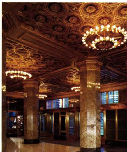
Conrad Schmitt Studios installed new gilded ornamental plaster to a previously bare ceiling at 35 East Wacker Dr., Chicago, IL.
