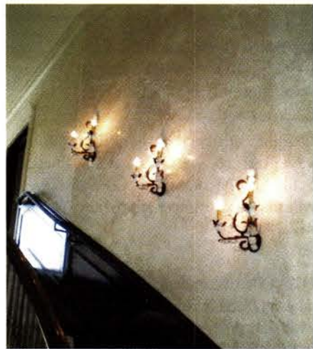
Conrad Schmitt Studios worked with Luczak Brothers, Inc. in the application of Venetian plaster to add the illusion of depth and texture to this wall.
