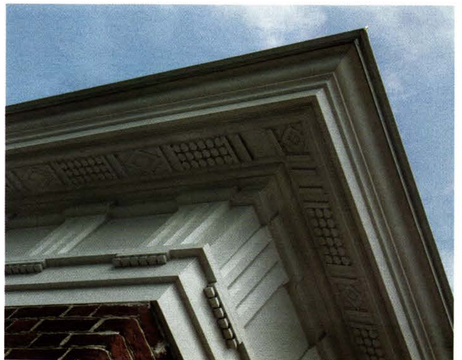
Built by Charles Karas in the SBD Kitchens mill shop, the Classical moldings are made of Azek cellular PVC. Each guttae had to be cut and applied individually and a c&c machine was used to carve the mutules.
