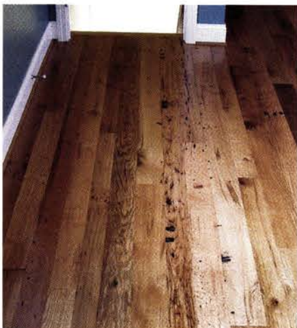
Chestnut Specialists manufactured this flooring, which is a combination of re-milled chestnut, red and white oak.
