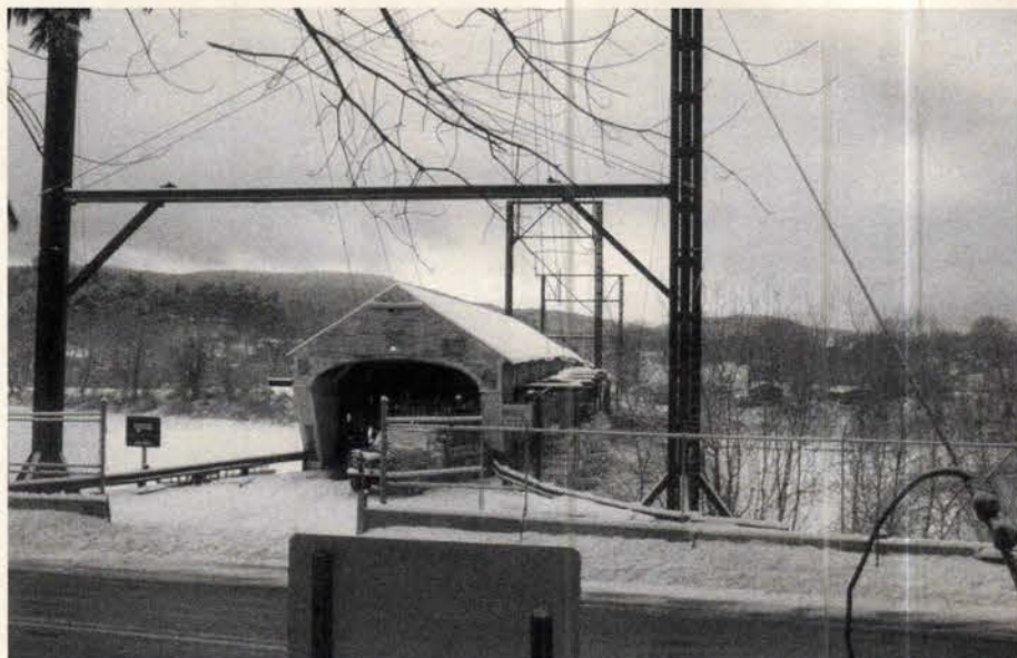
The Cornish-Windsor Covered Bridge was supported by a cable-stayed system that allowed work to progress during the winter.
