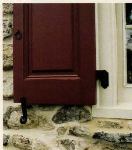
This exterior shutter from Vixen Hill is held back with a traditional shutter dog.
