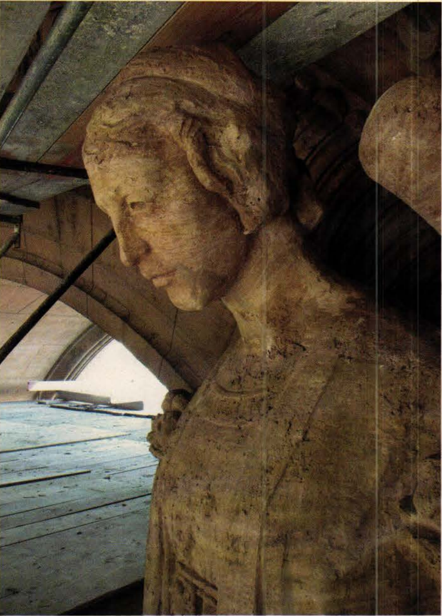
Concrete maidens have been pinned back onto the colonnade and patched in a variety of concrete hues. Photo: courtesy Carey & Co.
