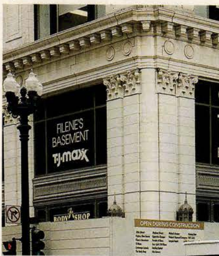
The terra-cotta elements on this commercial building in Chicago were replicated with GFRG elements with technology provided by Ball Consulting.
