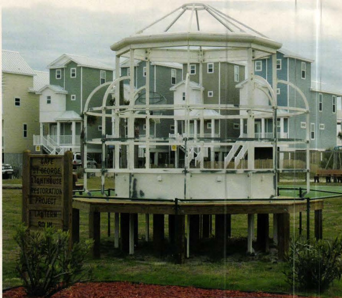
The rebuilt lantern room for the St. George Lighthouse, from Allen Architectural Metals, was assembled on a platform in a county park to stoke enthusiasm for the lighthouse reconstruction. Photo: courtesy of Kenneth Smith Architects
