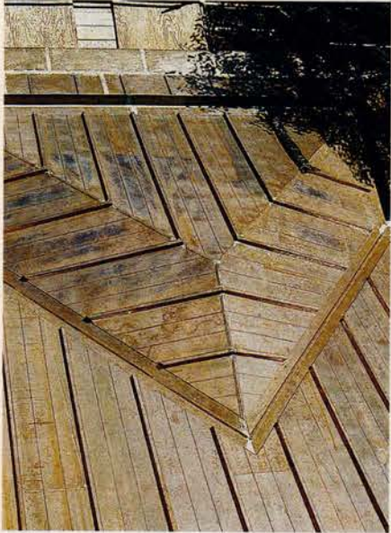
NIKO installed this batten seam and flat-lock copper roof for an historic building.
