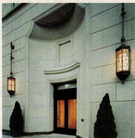
These solid cast-bronze exterior lanterns with leaded glass panels were designed and built by Lighting Nelson & Garrett for a Robert A.M. Stern building.
