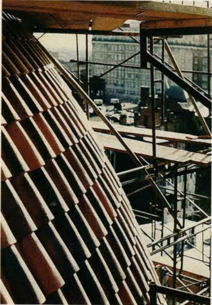
Boston Valley restored the terra-cotta roof tile of the Berea Temple in Baltimore, MD.
