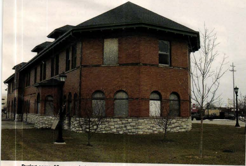
During some 40 years of abandonment, the forlorn depot's broad asphalt-shingled hip roof loomed over boarded-up windows. Photo: courtesy of Quinn Evans | Architects
