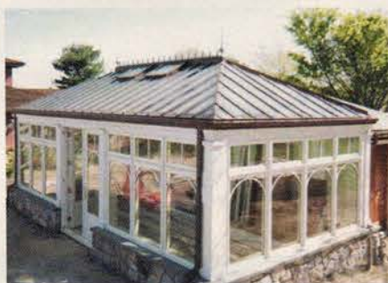
This conservatory pool house from Glass House, LLC features white painted mahogany framing, dentil molding and true divided lite transom windows over casement windows with applied arches.
