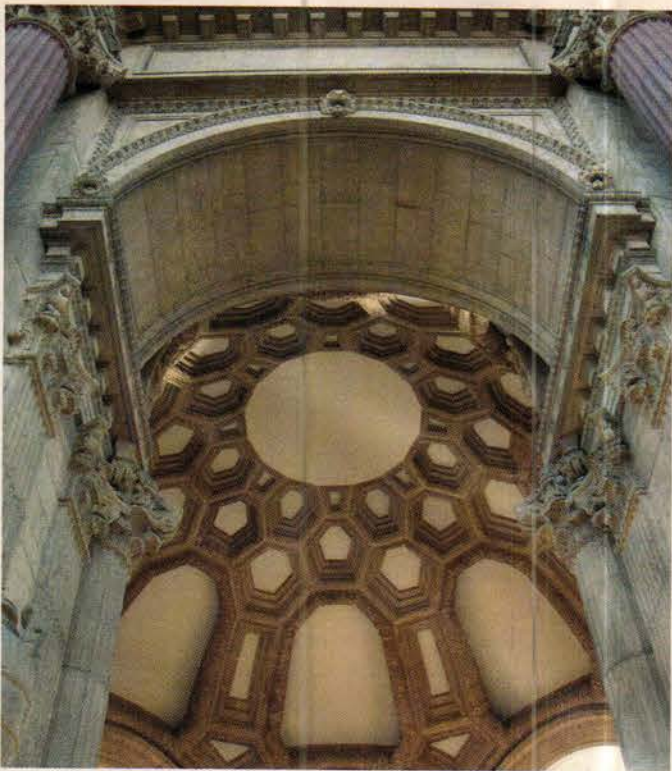
In the restored dome at the Palace of Fine Arts, angels bear up the concrete vaults. The coffers had spent nearly two decades engulfed in netting, after suffering earthquake damage. Photo: courtesy of Carey & Co.
