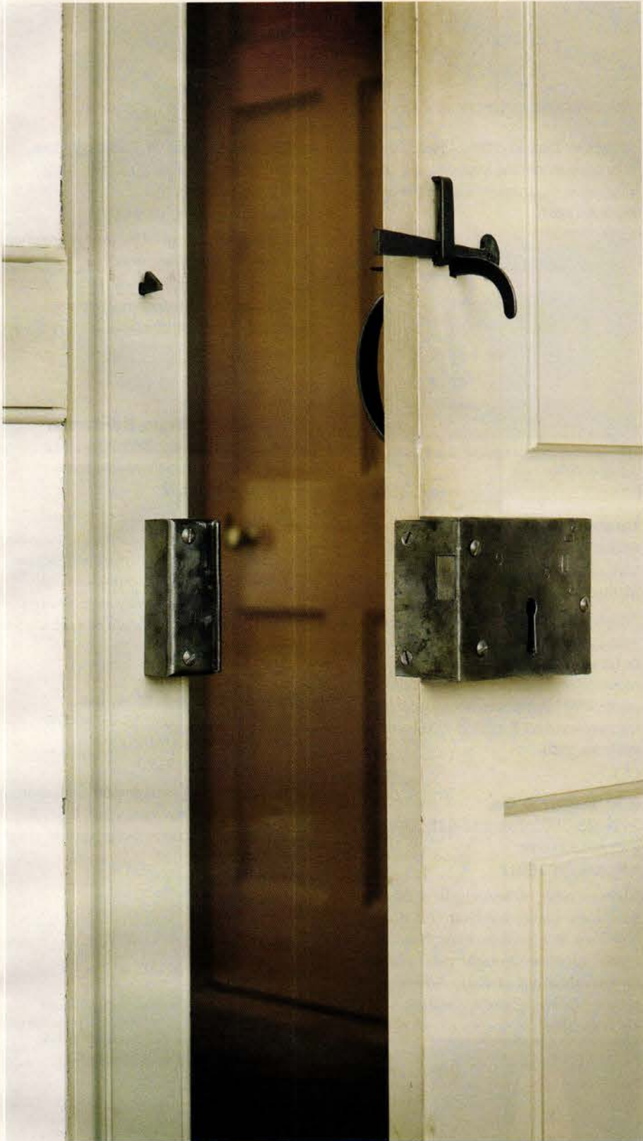
In the oldest section of the building, this interior door features a dead bolt with a hand-forged thumb latch. The metal was left unfinished for an aged appearance.
