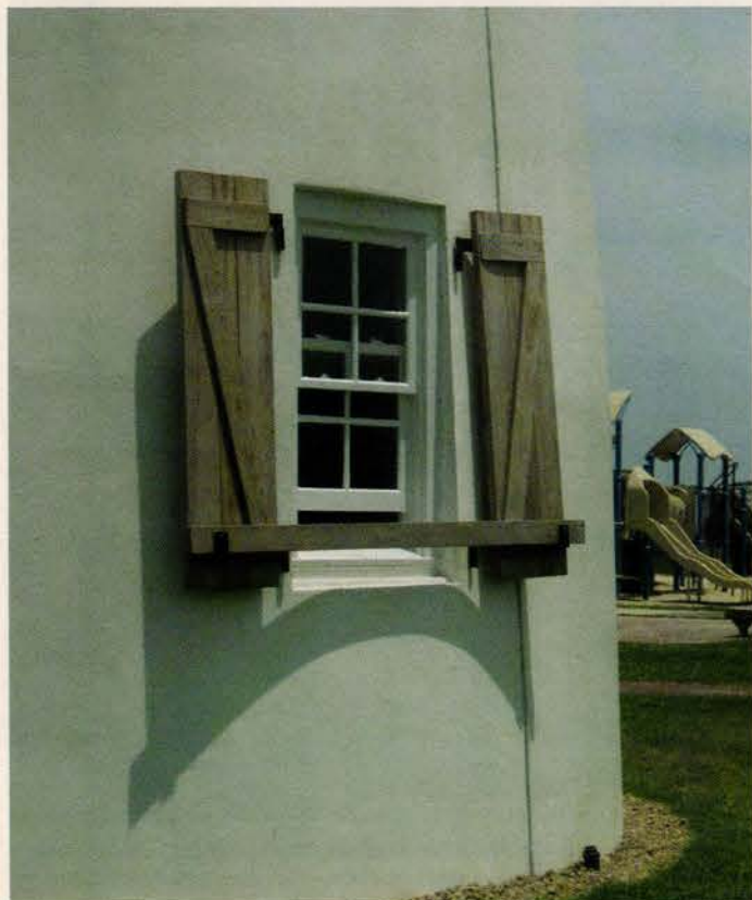
Left: Cypress shutters with Z-bar reinforcements flank windows cut into the thick brick shell of the St. George Lighthouse. Photo: courtesy of Kenneth Smith Architects
