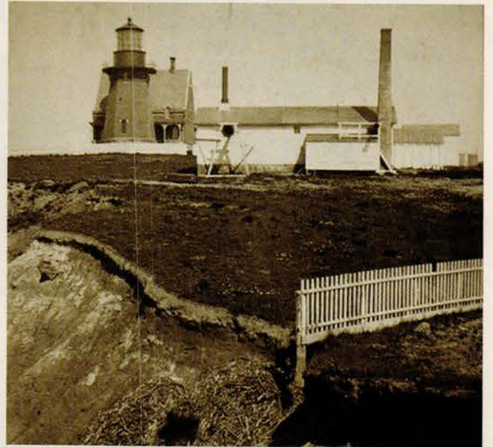
In 1993, the Southeast Lighthouse was hauled away from an eroding cliff, and then its nonprofit owners fundraised for a few years to solve structural and cosmetic problems. Porch gingerbread was missing, chimneys truncated, tower windows boarded up, and granite coping failing. Photo: courtesy of Dr. Gerald F. Abbott, Southeast Lighthouse Foundation
