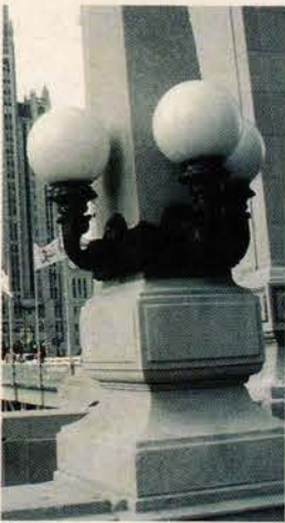
The city of Chicago commissioned Allen Architectural Metals to re-create these bronze obelisk light fixtures and cast-iron lampposts from original castings.
