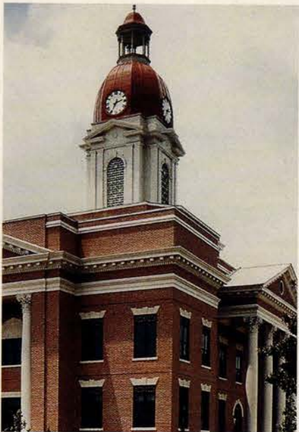
This aluminum cupola, with a 6-ft.-dia. clock and aluminum cornice, was created for the Worth County Courthouse in Sylvester, GA, by Campbellville Industries.
