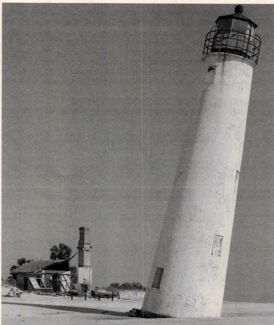
At its original site on a sandy island spit, the 1852 tower of the St. George Lighthouse was canted and rusted, and its lighting apparatus was missing. Photo: Tom Baird, Historic American Buildings Survey, 1998
