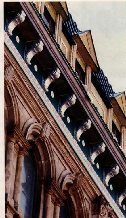
This stamped sheet-metal cornice was fabricated by W.F. Norman Corp.
