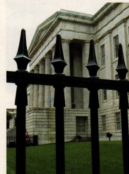
O.K. Foundry Co. reproduced an 11-ft. section and a new gate for this cast-iron fence for the Smithsonian National Portrait Gallery, Washington DC; the gate weighs approximately 500 lbs. and was cast as one contiguous iron casting as an exact replica of existing gates.
