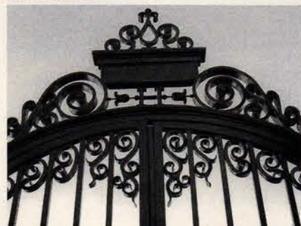
DeAngelis Iron Work fabricated this ornamental metal gate with hand-forged scrolls for a project at Harvard Yard in Cambridge, MA.
