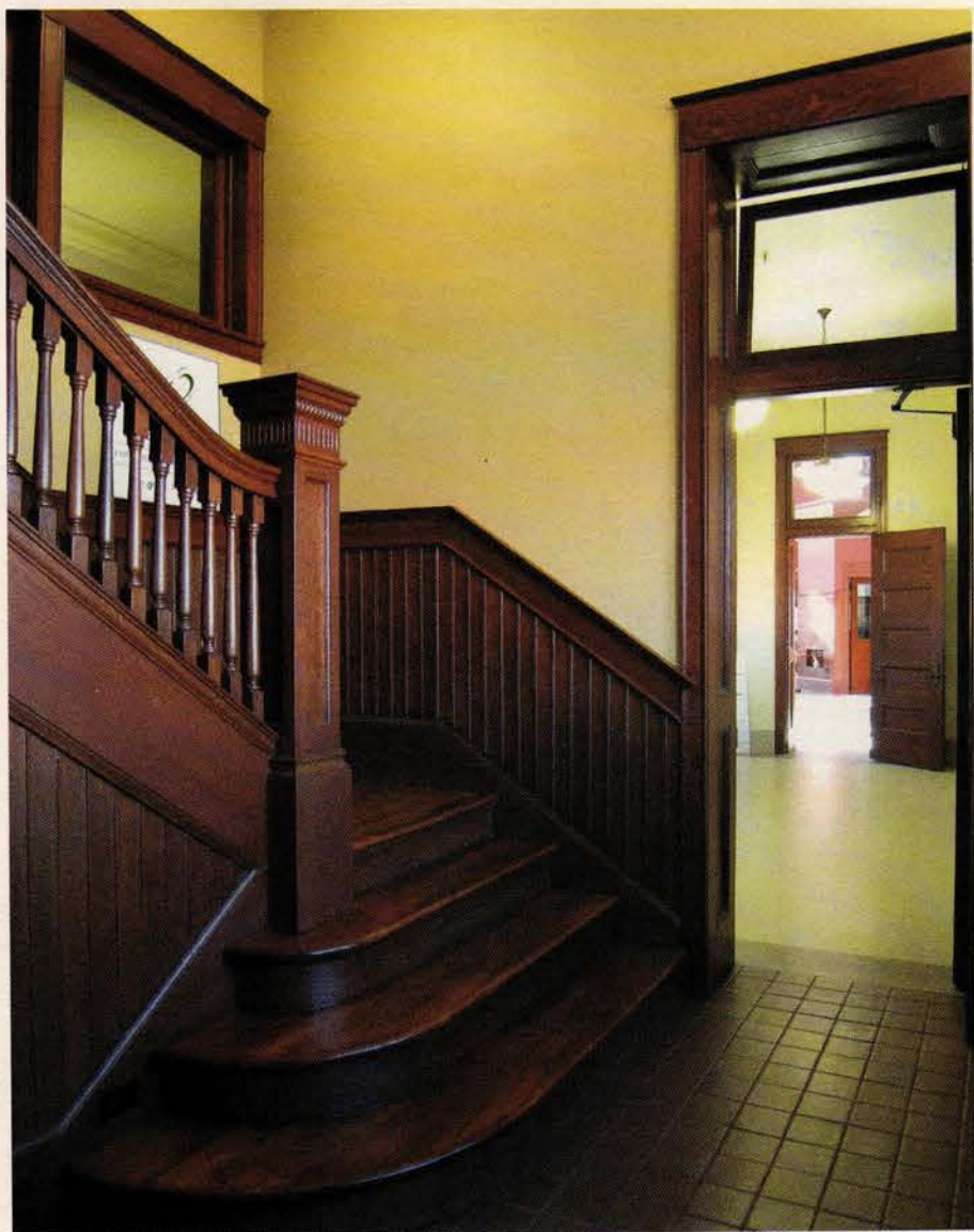
Above: The staircase's oak wainscoting and turned posts remained intact beneath peeling paint. Photo: courtesy of Quinn Evans | Architects
