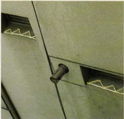
Made of all-natural, food-grade materials, Bird Barrier's Bird-Off Gel, shown here on recessed window ledges, repels birds but doesn't entrap them.
