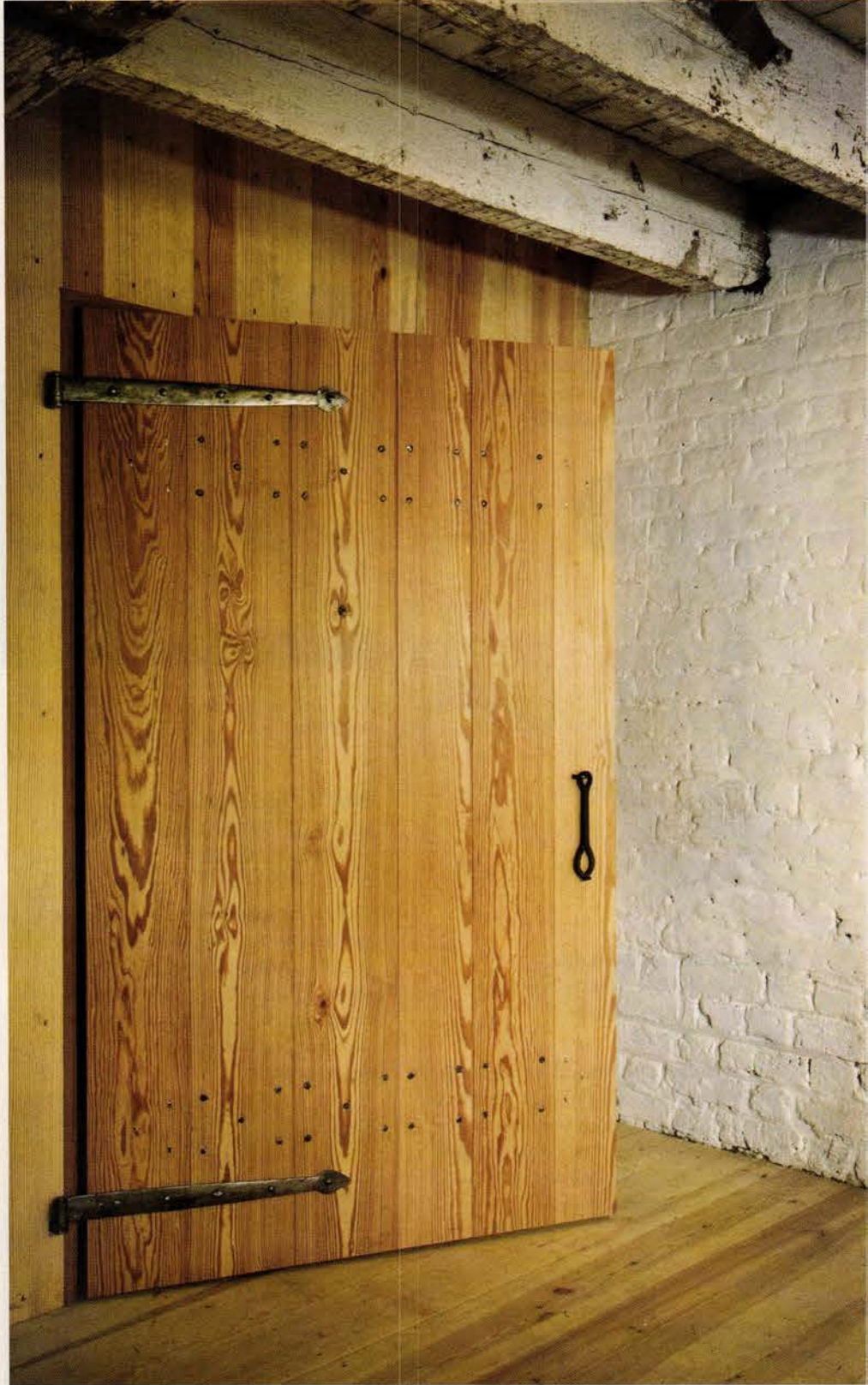
For this and two other adjacent cellar doors, Ball & Ball reproduced the existing strap hinges and produced the nails and rivets.
