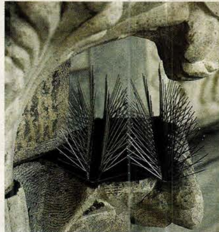
Nixalite bird-control spikes were used on the large, ornate columns under the cornice and pediment of the South Australia Parliament Building in Adelaide, Australia.
