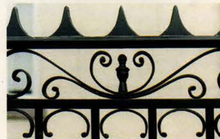
This detail shows the restoration work of Fine Architectural Metalsmiths on a gate featuring a saw-tooth "loafer's rail" and typical Vitruvian scrollwork.
