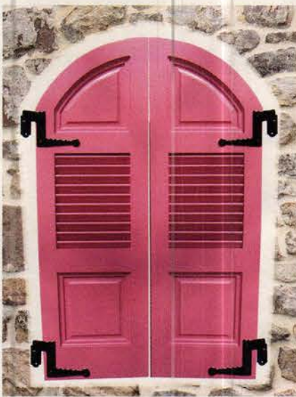
Vixen Hill's traditional arch-top, paneled and louvered shutter has cast stainless-steel hardware and hurricane panels.
