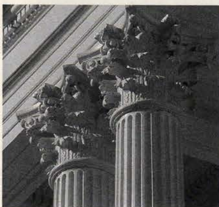
DeAngelis Iron Work, Inc. supplied and installed 12 cast-iron capitals for the exterior restoration of the Massachusetts State House.
