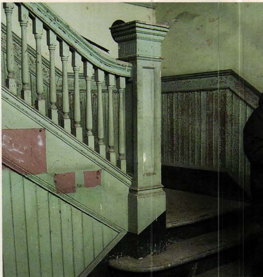
Above: The staircase's oak wainscoting and turned posts remained intact beneath peeling paint. Photo: courtesy of Quinn Evans | Architects
