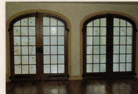
These elliptical arched-top french doors with double pane insulated glass were fabricated by Illingworth Millwork.
