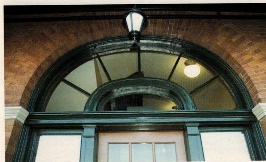
New ruddy mortar has been inserted between vintage ironspot bricks over a restored arched window.
