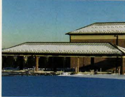
Large, forward-mounted polycarbonate snowguards from SnoBlox were used to prevent dangerous movement of snow and ice on this metal roof.
