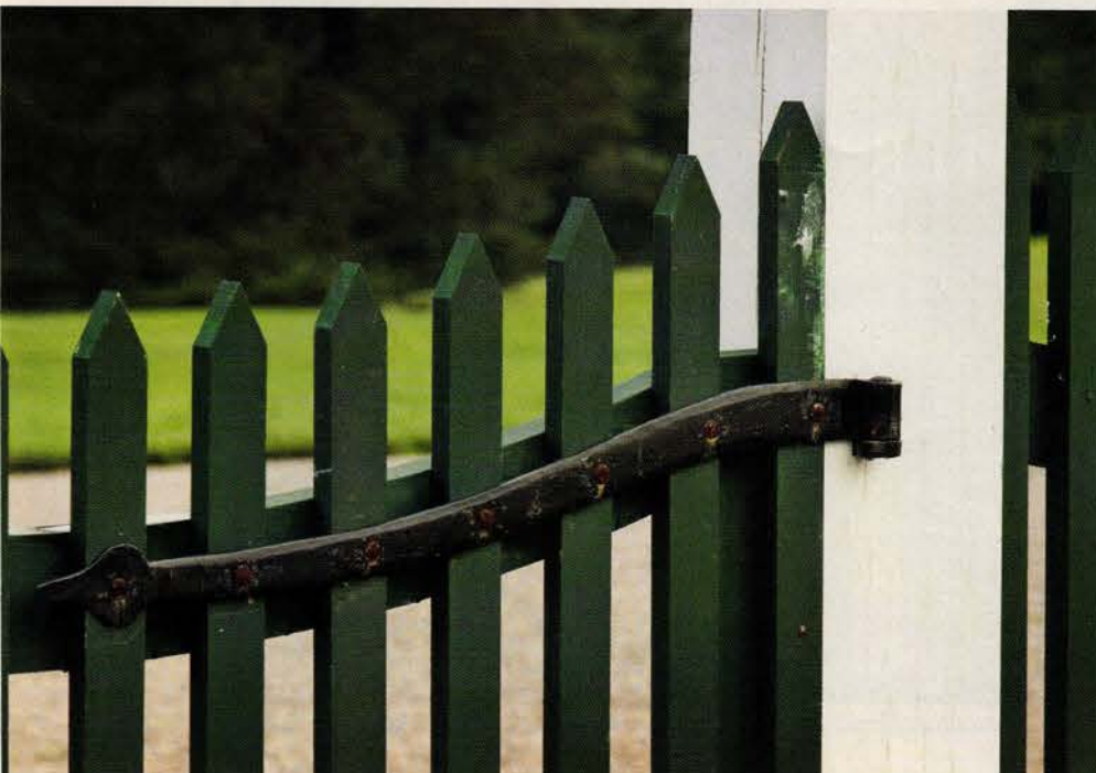
This entry gate hinge and hand-forged nails were manufactured to follow the gate form.
