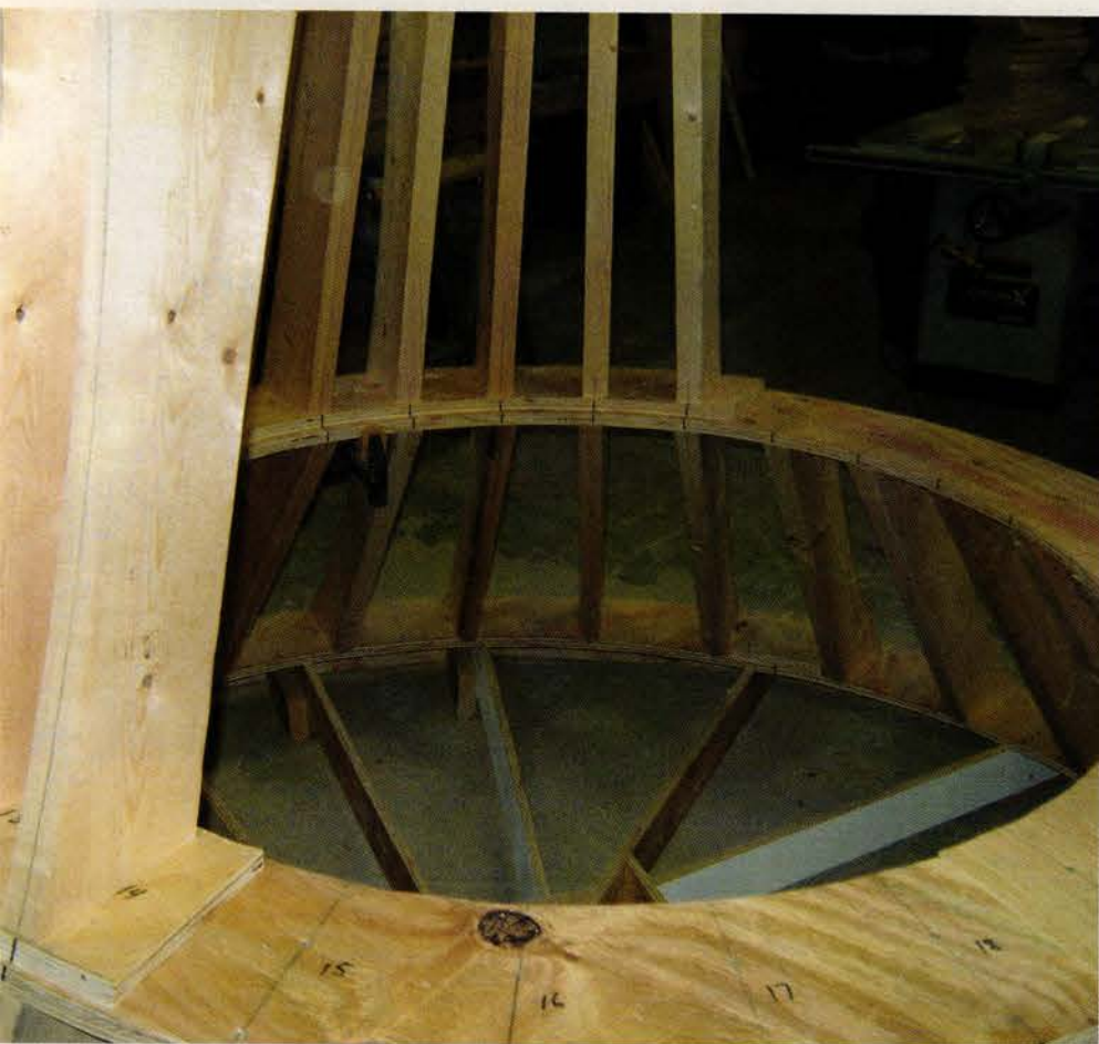
Wood rafters were all individually cut to accommodate the convex and concave surface of the bell-shaped roof design. The pieces were also carefully numbered to ensure correct installation when the base was taken apart to transport it to the rooftop.
