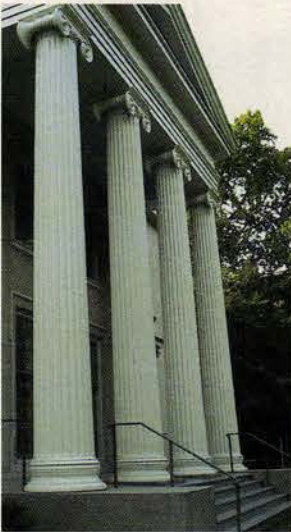
Fagan Design replicated this 30-in.-dia. x 20-ft.-tall fluted column (foreground) to match existing columns.
