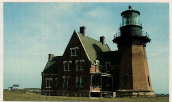
In 1993, the Southeast Lighthouse was hauled away from an eroding cliff, and then its nonprofit owners fundraised for a few years to solve structural and cosmetic problems. Porch gingerbread was missing, chimneys truncated, tower windows boarded up, and granite coping failing. Photo: courtesy of Dr. Gerald F. Abbott, Southeast Lighthouse Foundation
