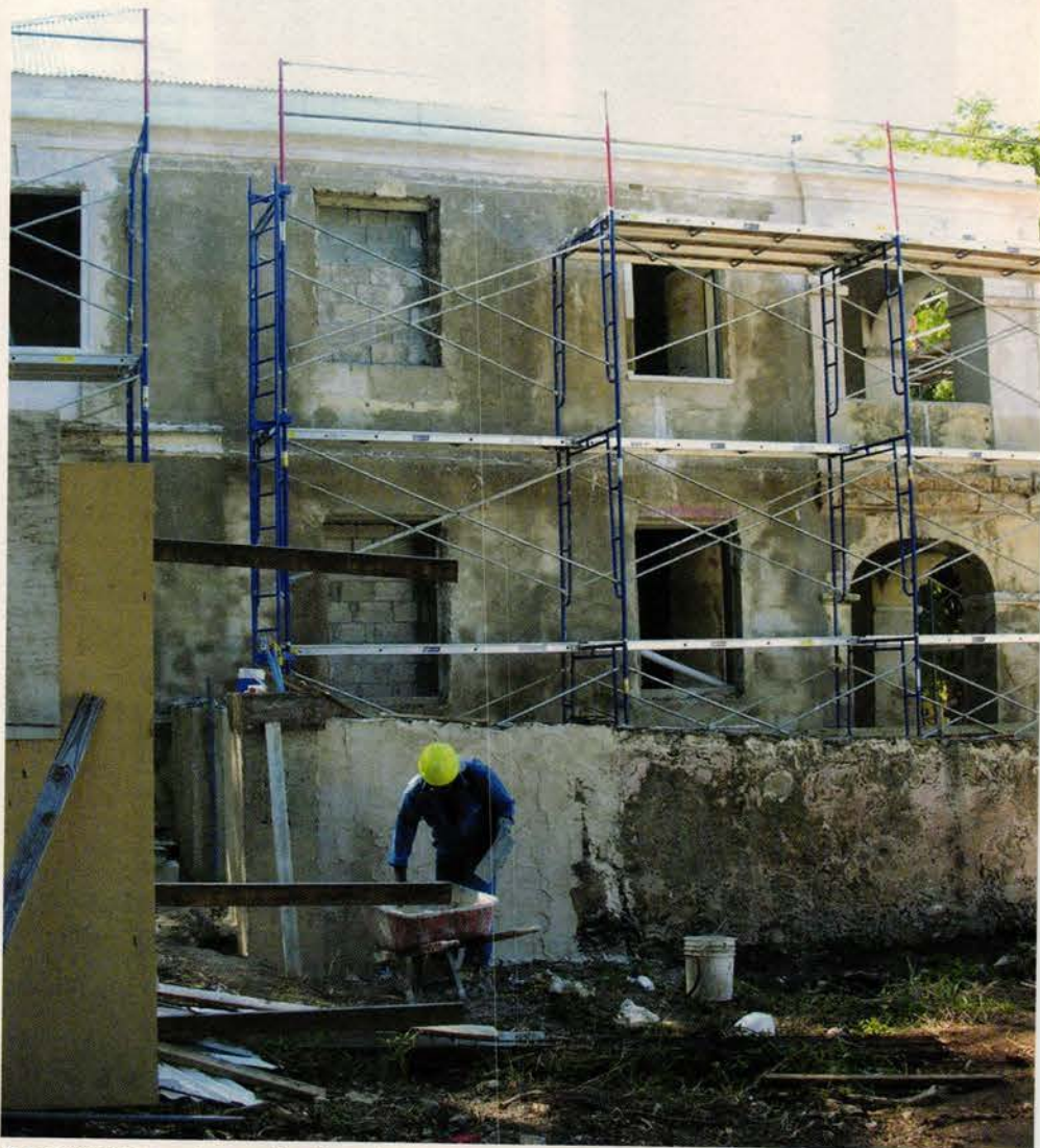
A construction worker applies lime plaster to the outbuilding.
