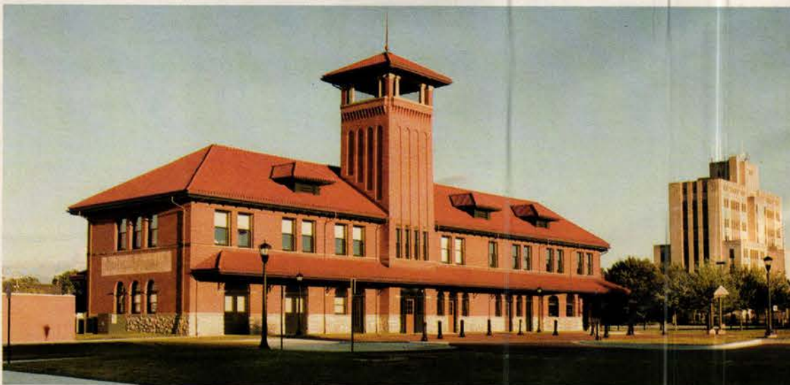
The tower roof was craned onto the rebuilt tower, built of tapered, corbelled, load-bearing masonry with slit windows and fluted recesses.
