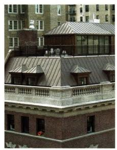
NIKO fabricated the copper dormers and mansard roof and also installed the copper penthouse for this NYC building
