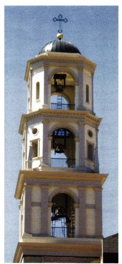
Manufactured primarily of aluminum by Munns Manufacturing, the bell tower holds three bells that are hand rung. Photo: Munns Manufacturing
