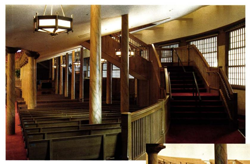
Two new exit stairs help move crowds from the balcony to the main hall and aid fire safety. The detailing matches the balcony railing and adjacent features.
