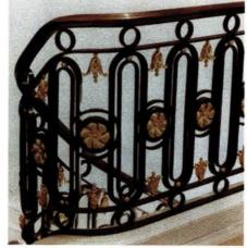
This stair balustrade, fabricated by Schwartz's Forge & Metalworks, has gilded repousse leaf work and a custom bronze cap rail.
