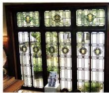
An interior storm from Climate Seal provides insulation while protecting the appearance of this historic
