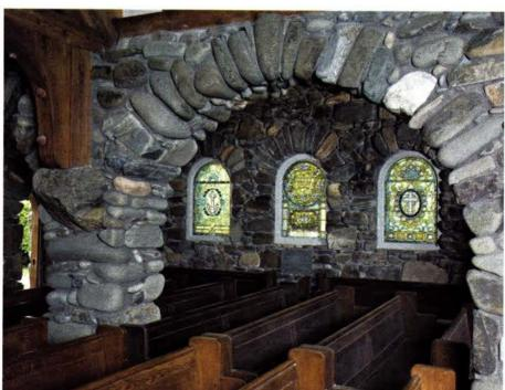
Above: When repointing the stone in the interior, a dark mortar was used so that it would be less visible. The church's stained-glass windows were restored by Phoenix Studio in Portland, ME.
