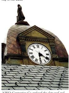
NIKO Contracting Co. replaced the slate roof and sheathed the clock-tower dome in copper on the Hancock County Courthouse in Findlay, OH.
