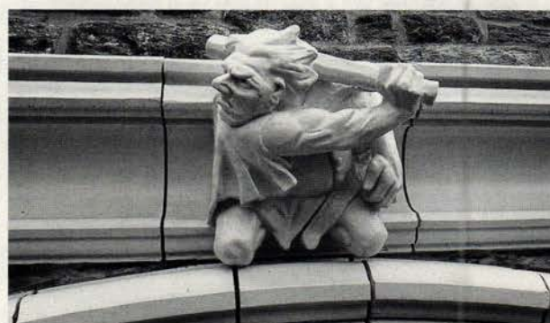
This terra-cotta gargoyle was fabricated by Gladding, McBean for Wingate Hall at City College of New York to replace one that was missing.
