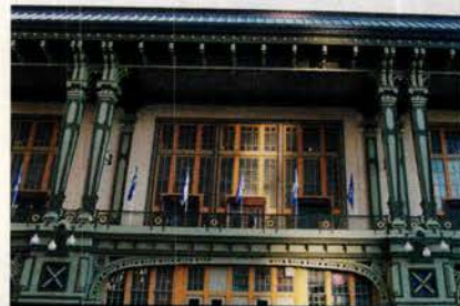
Allen Architectural Metals replicated and restored the cast-iron façade and railings for this 140,000-sq.ft. 1909 Beaux-Arts landmark building in New York City. Click on No. 1023
