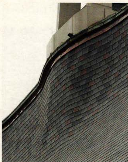
Composite slate roofing from InSpire Roofing was used to rejuvenate this 85-ft.-tall, 140-ft.-wide roof. Click on No. 1932
