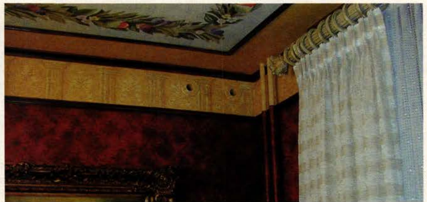
Unico's small-duct, high-velocity HVAC system takes less than 1/4 the space of a traditional system, making it ideal for historic buildings.
