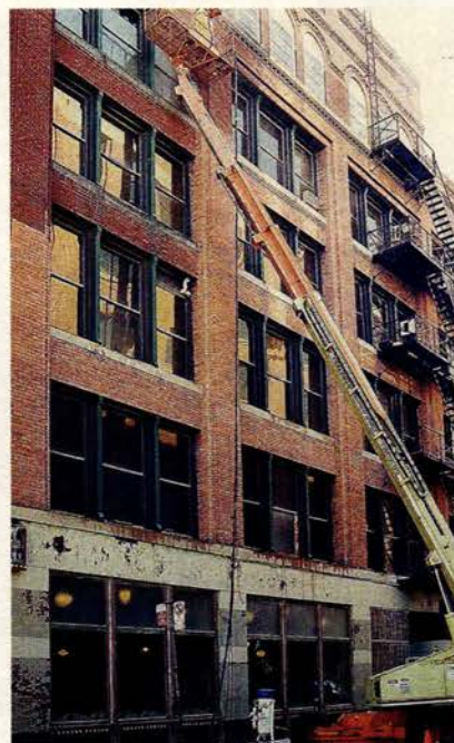
ArmaKleen Co. used Armex, a baking soda-based media, to clean the Boydell Building in Detroit, MI.
