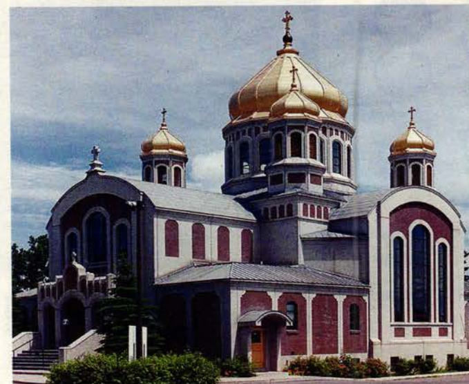
The original exposed concrete domes of St. John the Baptist Church in Ottawa were clad with pre-painted sheetmetal by Heather & Little . Click on No. 2470
