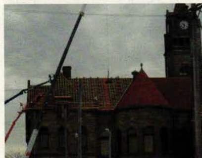
Team Fritz Clay Roof Tiles replaced the original red clay tile roofing for the historic City Hall in Bay City, MI; the tile was manufactured by Creton AG in Germany. Click on No. 2015
