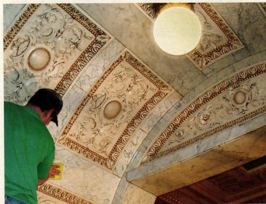
EverGreene Architectural Arts developed the methodology to clean tobacco-stained Italian marble in the three-story-tall double grand staircase of the Allen County Courthouse in Fort Wayne, IN. Click on No. 2460
