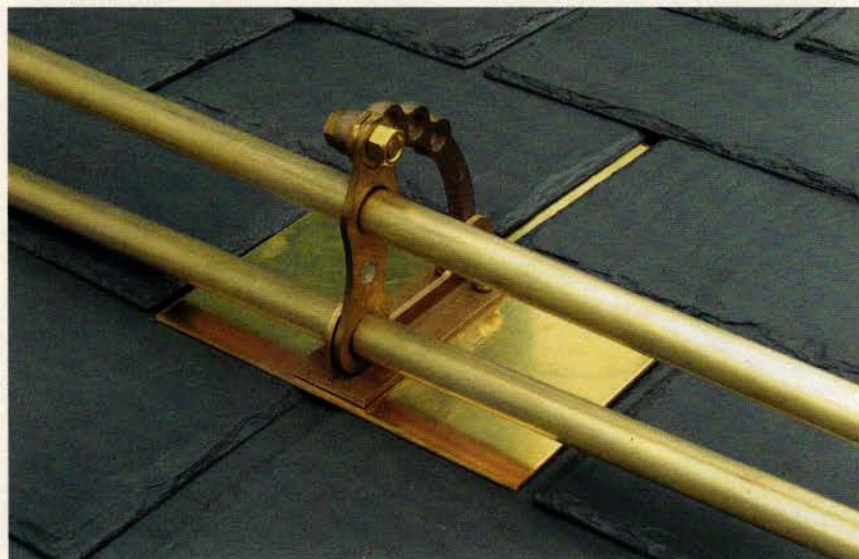
Alpine SnowGuards' model # 502 brass two-pipe snowguard is shown on a synthetic slate roof. Click on No. 145
