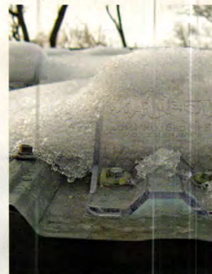
Designed for metal roofs, the Ice Jax II clear polycarbonate snowguard from Snoblox holds 6,388 lbs. of snow when screw mounted.
