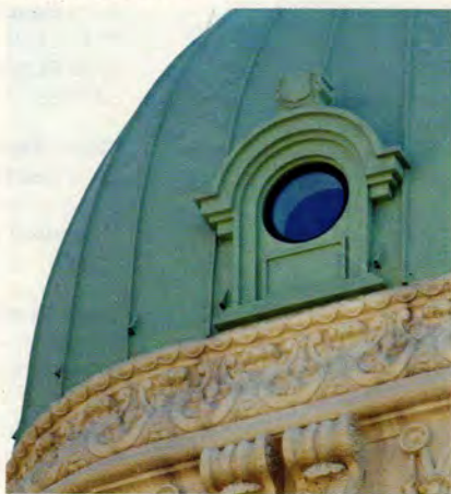
Gotham Metalworks fabricated this precision plasma cut replication domed roof for a NYC landmark building.
