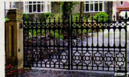
This iron gate for a 12-ft. opening was cast in one piece by Wiemann Metalcraft; it was installed on in-ground hydraulic operators.
