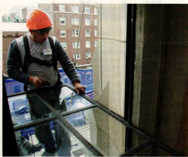
After the Columbia windows were restored in the shop, they were put back in the building where workers installed and putty-glazed the glass. Seekircher worker Omar Hernandez is shown here glazing one of the windows.
