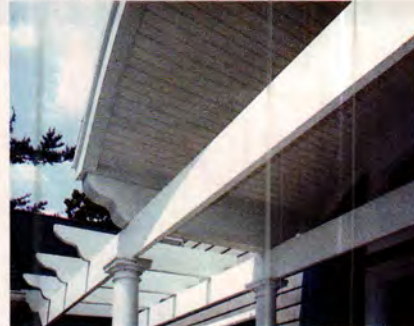
This custom pergola from Goodwin Associates uses girders and cross rafters of reinforced board that is maintenance-free and rot-resistant.
