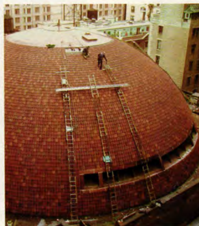
The dome of the New York City Center was originally finished in Ludowici Roof Tile in 1923; it was restored with roof tile from the same company in 2004.
