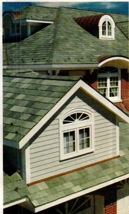
TruSlate roofing from GAF combines traditional slate with a high-tech waterproofing material.
