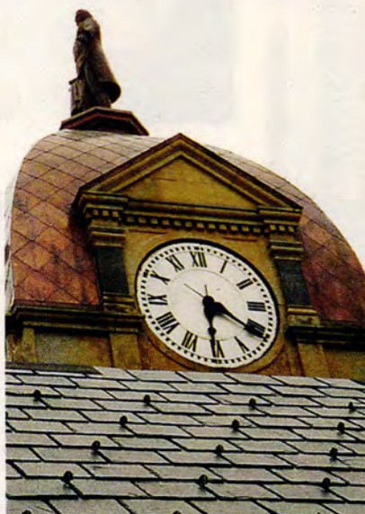
NIKO replaced the slate roof and sheathed the clock-tower dome in copper on the Hancock County Courthouse in Findlay, OH.
