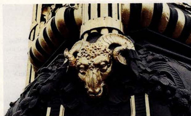
This copper ram's head, fabricated by Heather & Little , is part of the restoration work done on San Francisco City Hall.
