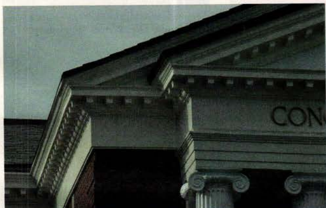
Architectural Fiberglass Corp. restored the cornice for the Temple Beth Shalom in New York City.
