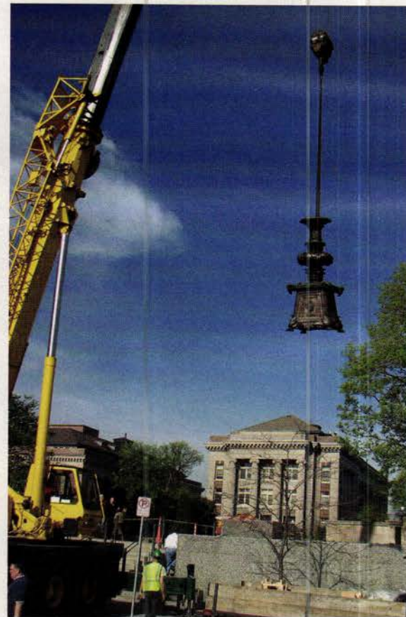
St. Louis Antique Lighting Co. utilized a crane with a 100-ft. boom to lower exterior standards weighing nearly a ton each onto the wing walls of the University of Minnesota's Northrop Hall. Photo: Gary H. Behm, IES
