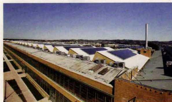
The Ford Motor Co. Assembly Plant in Richmond, CA, built in 1930 and placed on the National Register of Historic Places in 1988, has a 1-megawatt high-efficiency SunPower solar power system on its roof. SunPower designed the system to take advantage of Ford's original saw-tooth roof design, positioning solar arrays on south-facing tilted angles that are perfect for maximizing energy production. The system generates nearly all of the electricity required by the building tenants, but cannot be seen from the ground. Photo: courtesy of SunPower
