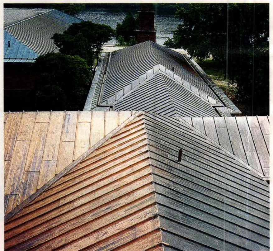
NIKO Contracting installed this batten-seam and flat-lock copper roof.
