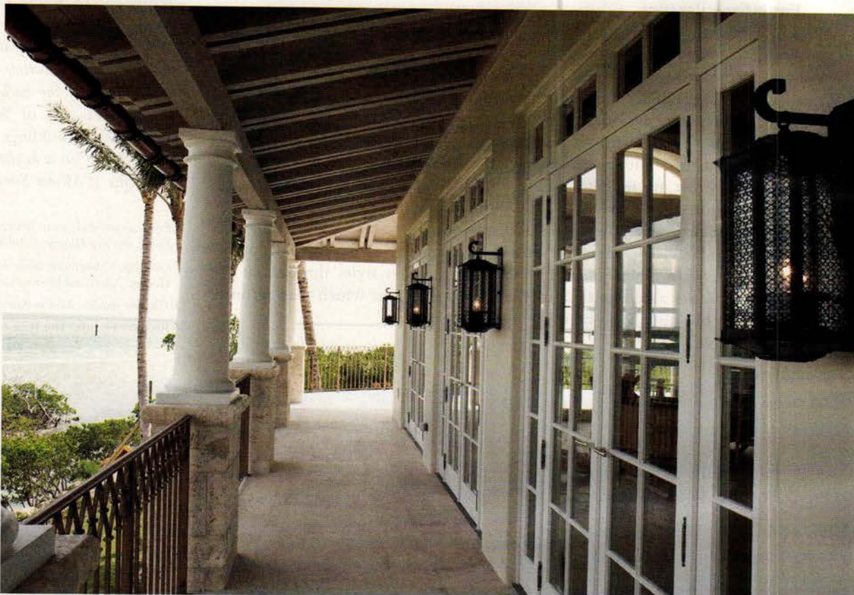
These hurricane-resistant lanterns were fabricated in bronze by Remains Lighting for a location near the Atlantic; the lacy grille work was cut from fine brass sheets. Photo: courtesy of Remains Lighting
