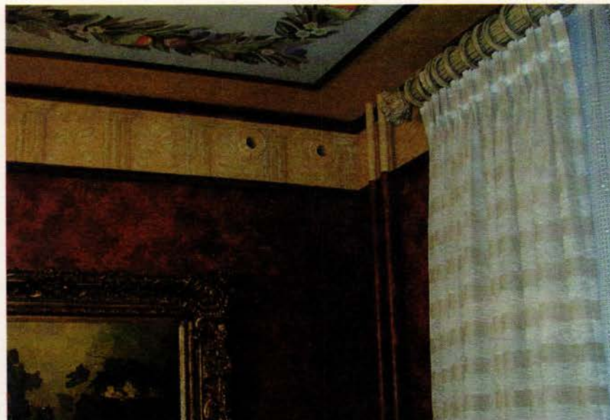
Unico's small-duct, high-velocity HVAC system takes up less than a quarter of the space of a traditional system, making it ideal for historic buildings.
