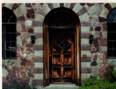
HeartWood Fine Windows & Doors made this 2¼-in. thick mortise-and-tenon solid-wood door of sawn white oak to replicate the original door made 100 years ago.
