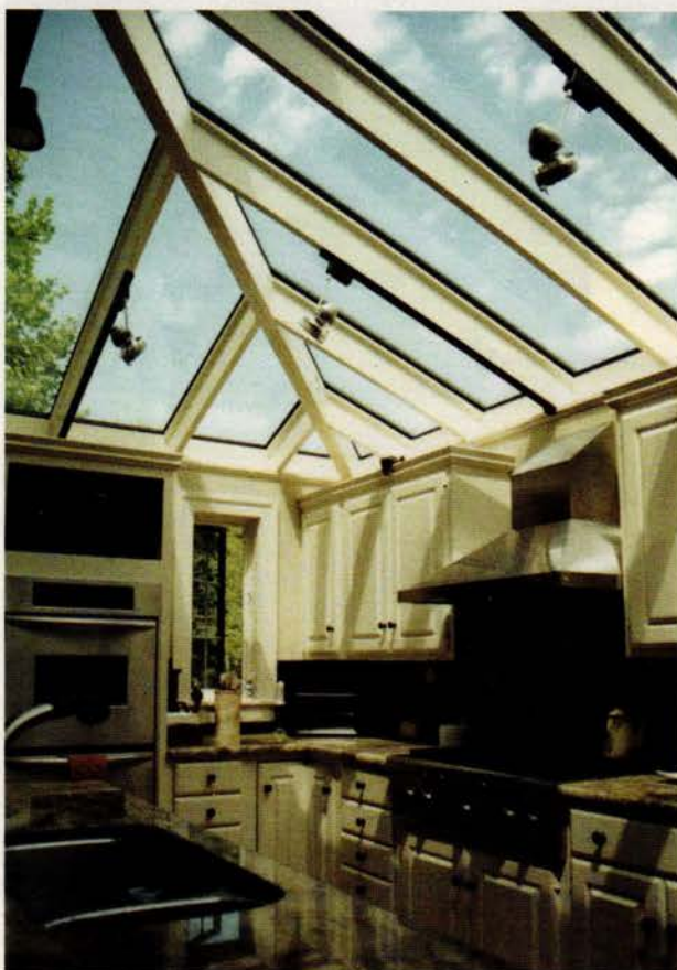
This mahogany frame hip corner skylight glass roof system with state-of-the-art glazing was designed, fabricated and installed by Glass House, LLC.
