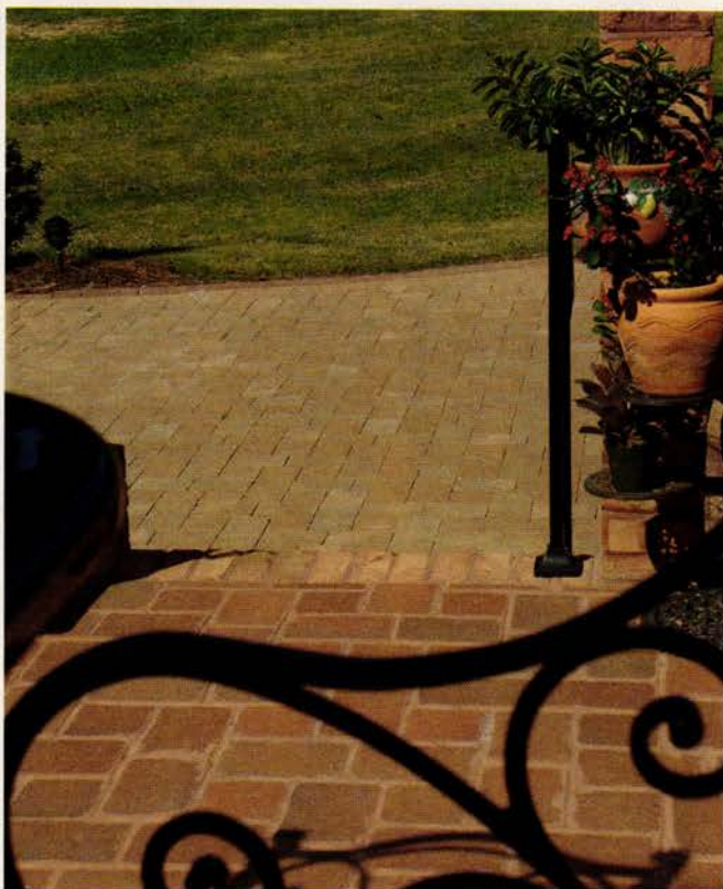
Pine Hall Brick's CityCobble pavers are tumbled after firing, giving them a cobbled look; the pavers exceed ASTM standards for strength and durability and will not fade.
