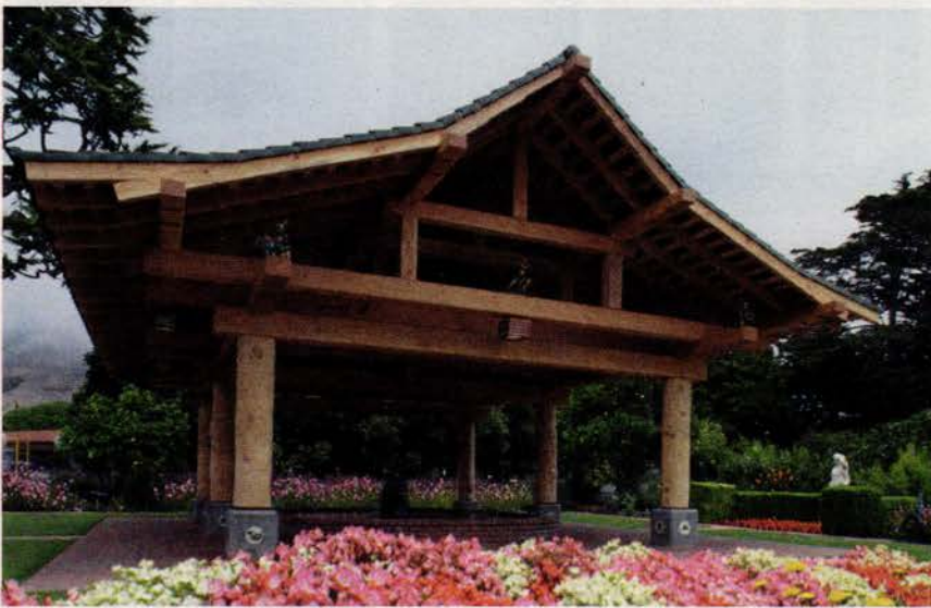
This Douglas fir pagoda-style timber frame was built in Shell Beach, CA, by Pacific Post & Beam as a koi pond cover; it features mortise-and-tenon joinery and a tile roof.
