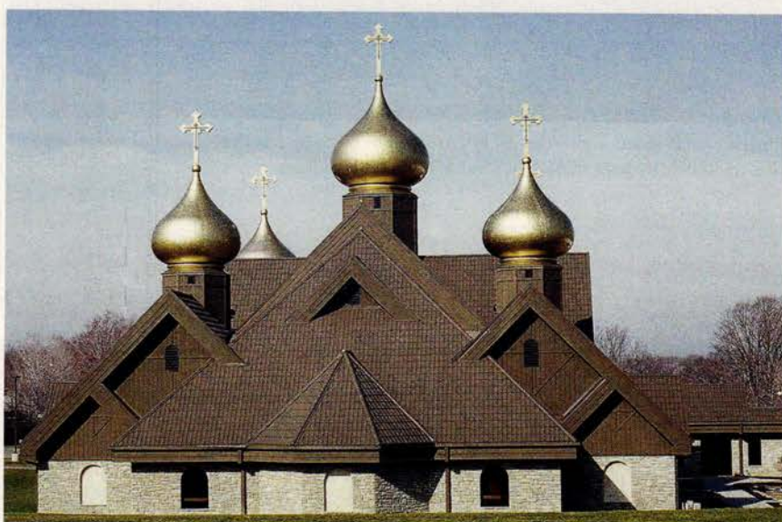
Five onion-style golden domes were custom manufactured and installed by Architectural Fiberglass, Inc. on the Holy Trinity Church in Parma, OH; one measures 18x32 ft. and the other four are 15x26 ft.
