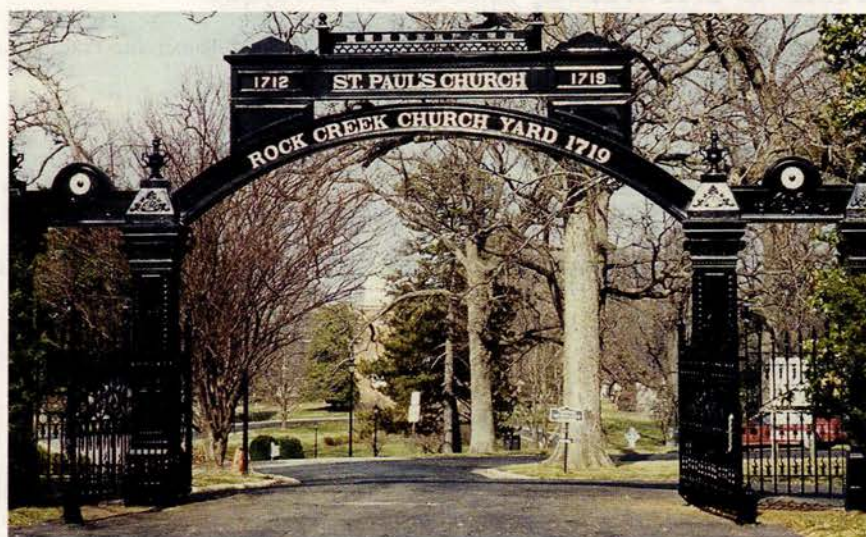
Architectural Iron restored this massive cast- and wrought-iron main gate for the Rock Creek Cemetery in Washington, DC.
