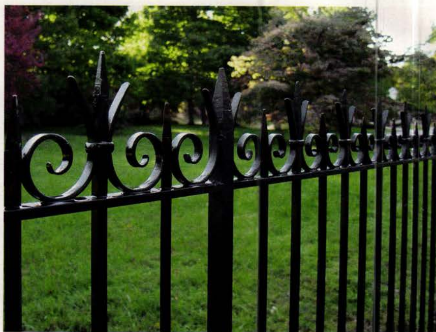
This custom fence was designed and fabricated by Wiemann Metalcraft using solid-bar steel; to ensure longevity, it was galvanized before urethane coating was applied.
