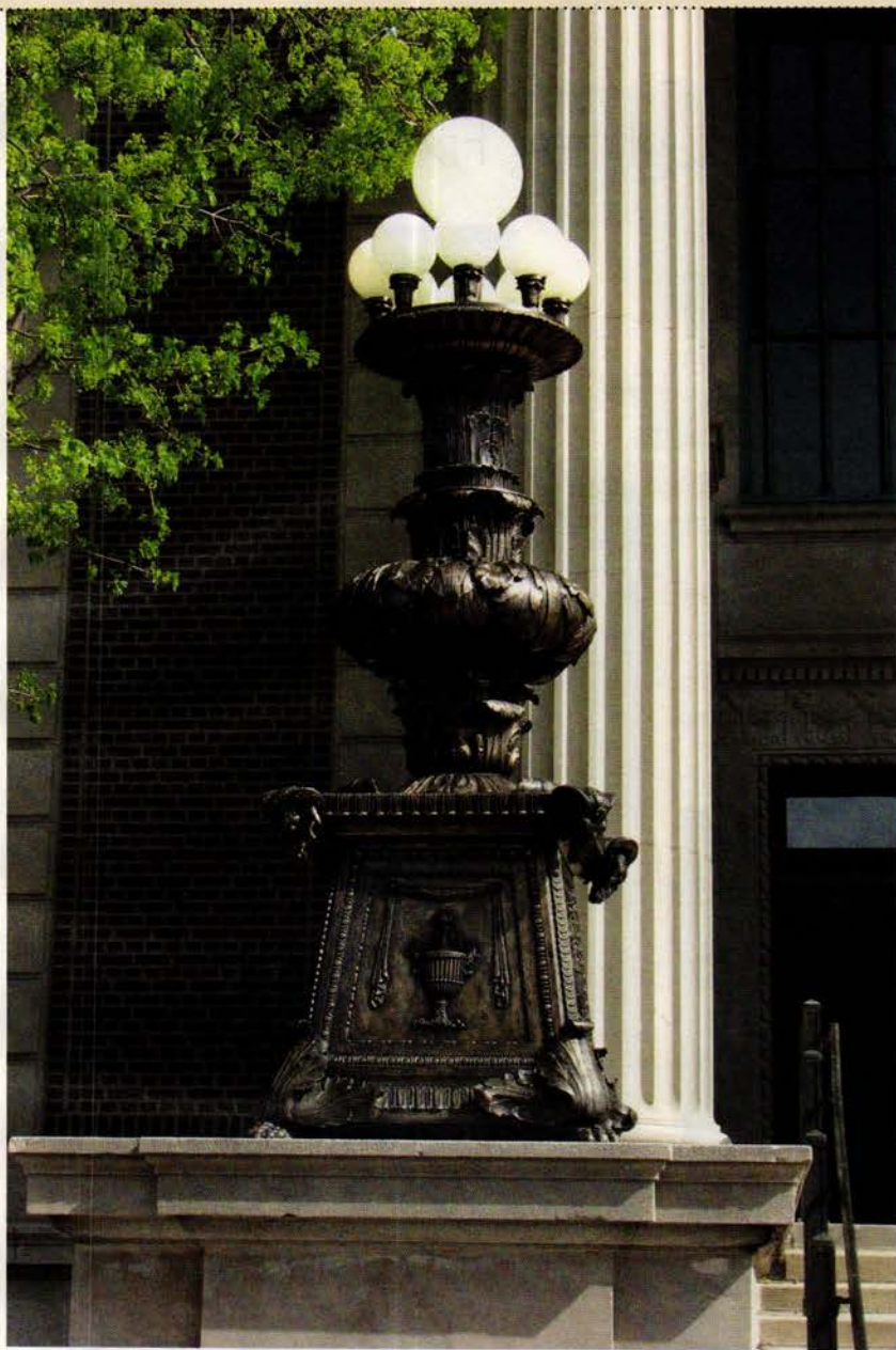
Above: The exterior standards for the University of Minnesota were cast from bronze using the 'lost wax' method; they were replicated from original drawings by St. Louis Antique Lighting Co. Photo: Gary H. Behm, IES
