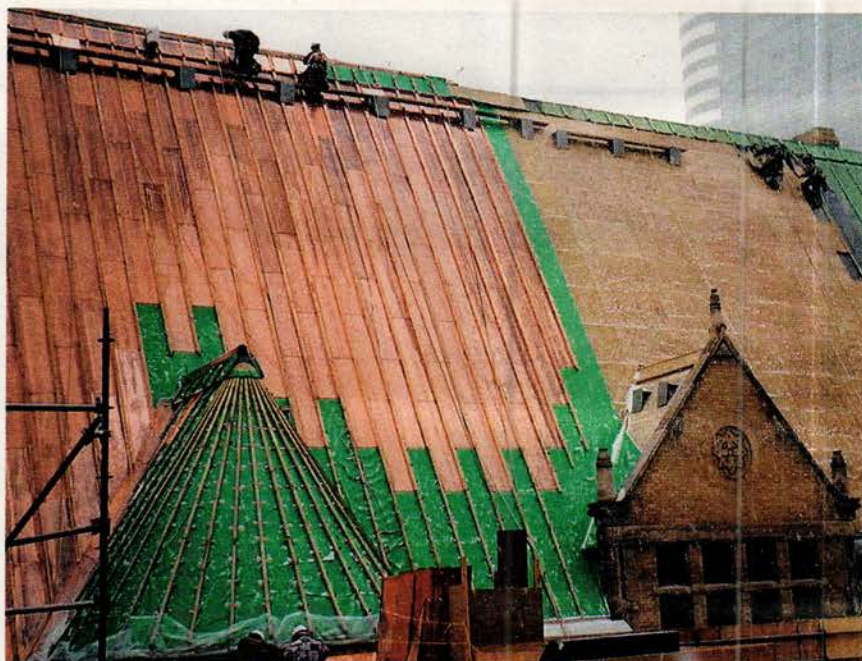
Heather & Little's restoration of the Toronto Old City Hall required 113,900 sq.ft. of copper roofing, cornices, gutters and sheet-lead work.
