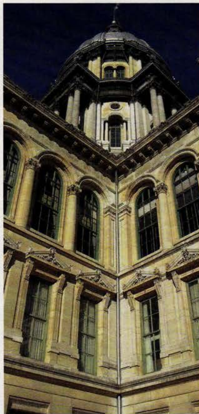
Re-View restored the wood windows and manufactured historically correct wood window replicas for the Illinois State Capitol project.
