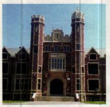
On Staten Island, NY, Graciano Corp. completed extensive historic masonry conservation at Wagner College's Main Hall; it included restoration, waterproofing and exterior cleaning of the 1929 precast-concrete building, as well as rebuilding parapets and copings, reconstructing the top half of two five-story Gothic-style turrets, and replacing the dome that surmounts one of the turrets.
