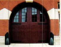
The renovation of this historic firehouse included eco-friendly strap hinges and back plates (37% recycled steel in content and coated with a no VOC powder coat) from Richards-Wilcox.
