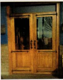
Kayne & Son fabricated the forged hinges and thumblatches for the renovated doors to the Jack of the Wood pub in Asheville, NC.
