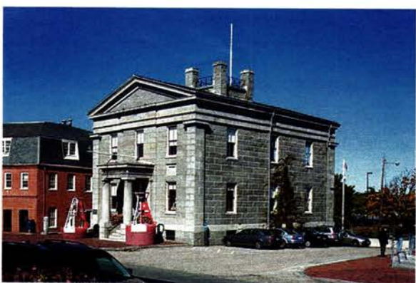
Architectural Components restored the double-hung windows for the Customs House Maritime Museum in Newburyport, MA; the windows feature laminated single-pane glass and are counter-balanced with weights and pullies. Call for more information.
