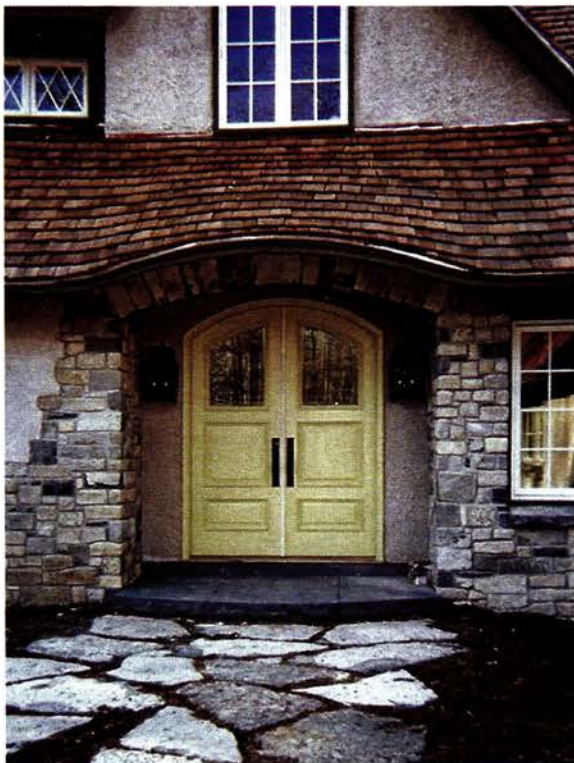
Illingworth Millwork built this custom mahogany radius arch-top double entryway door unit; it incorporates double-pane insulated glass with a bevel edge. Click on no. 1696
