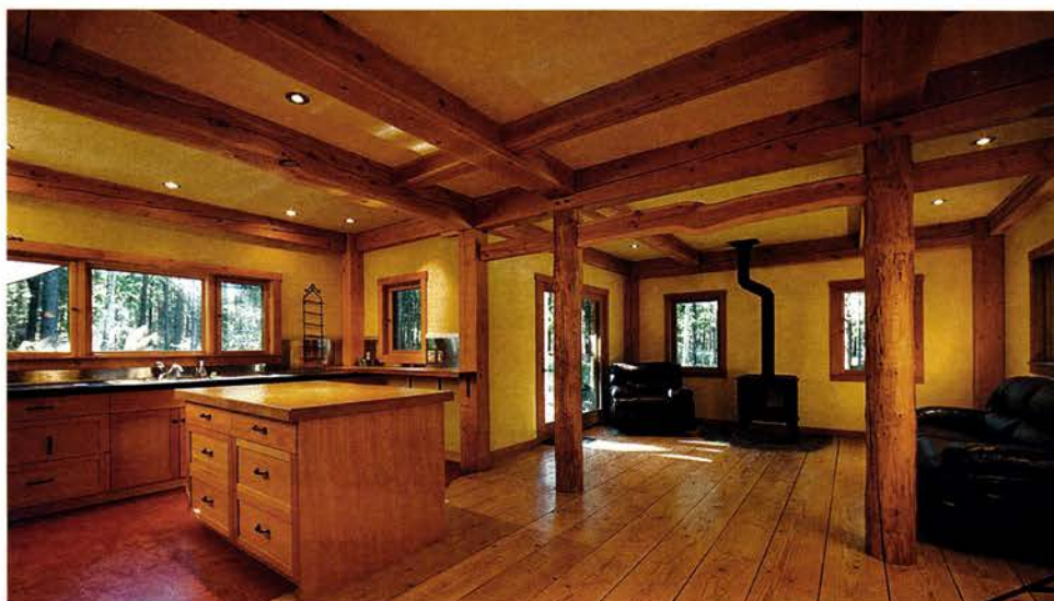
This timber-frame structure features Douglas fir and western red cedar from Bear Creek Lumber .
