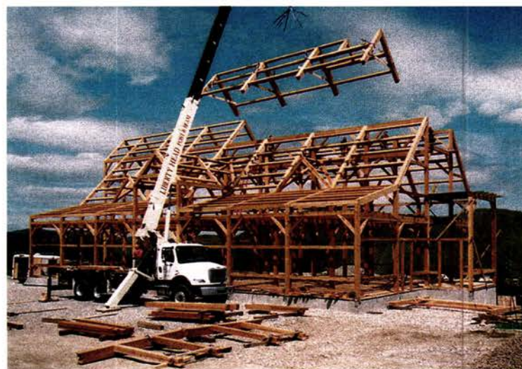
Liberty Head Post & Beam built this barn from recycled Douglas Fir timbers in Huntington, VT; it also incorporates renewable solar energy technologies.
