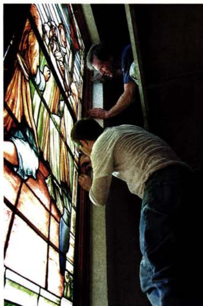
Conrad Schmitt Studios created and installed these new traditionally styled stained-glass windows; the installation was facilitated by the use of wide sashes, parting stops and easily removable trim. Click on no. 1841
