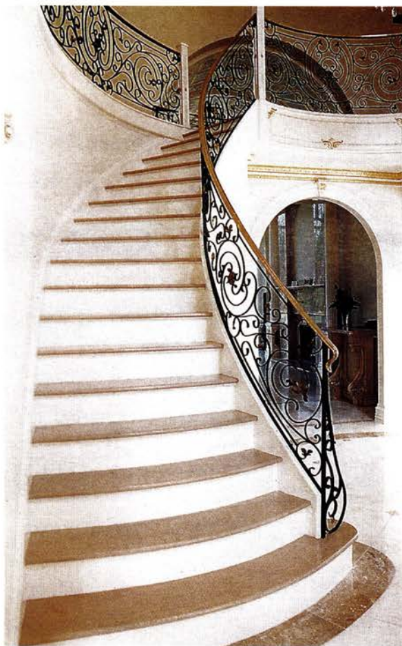
This railing, forged by Fine Architectural Metalsmiths , includes patinated antique gold leaves and rosettes and a top rail of polished bronze. Click on no. 2640
