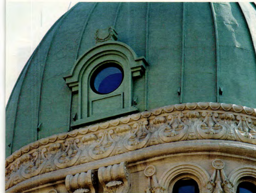
Gotham Metalworks fabricated this precision plasma-cut replication domed roof for a NYC landmarked building.
