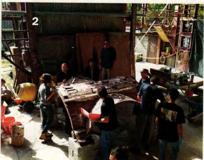
1. At a two-day workshop held at A. Ottavino stone yard during the APTI conference in October 2013 in NYC, a team of craftspeople built two Guastavino vaults. Here they are working on vault #1. All photos: Ken Follett unless otherwise noted
