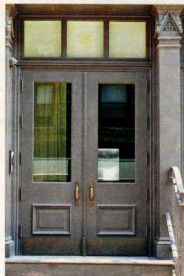
This custom SoHo entry was manufactured by Artistic Doors & Windows to identically match the landmark details from 1898.
