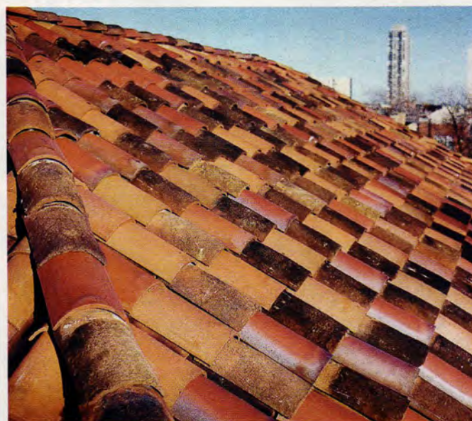
TOP: Tile Roofs supplied the salvaged red French tile and custom-made fittings for this old train depot in Fithian, IL. Photos (both): Tile Roofs, Inc.
