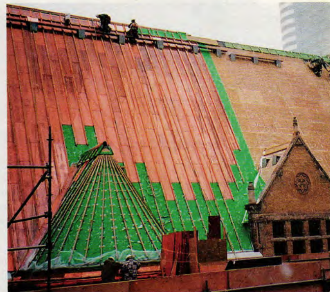
TOP RIGHT: NIKO Contracting installed the batten-seam and flat-lock copper roof of the Kingswood School in Bloomfield Hills, MI. Photo: NIKO Contracting
