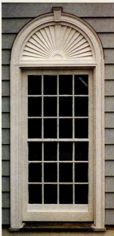
This reproduction 12/12 window with fan was manufactured by Architectural Components.
