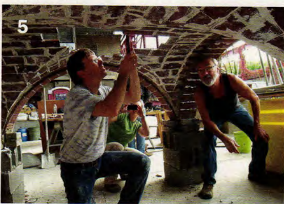
2. The team starts work on vault #2, a barrel vault with two lunettes.
