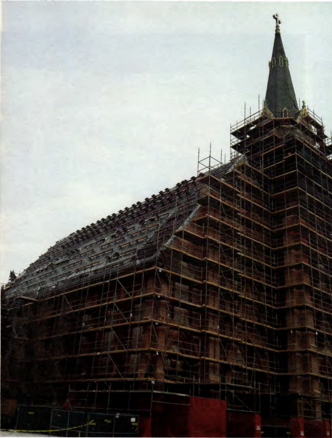
TOP: Ludowici's 18- and 13-in. Spanish "S" Tile was used for this building. The color is Terra-Cotta Impressionist. Photo: Ludowici Roof Tile
