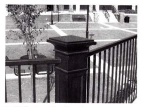
This custom cast-iron stanchion was fabricated by O.K. Foundry.
