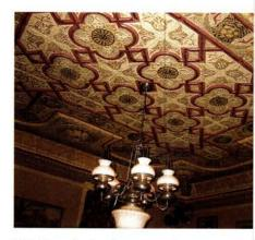
This Oriental-style ceiling was created using pressed-tin panels from W.F. Norman Corp.
