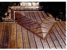
NIKO installed this batten-seam and flat-lock copper roof for an historic building.
