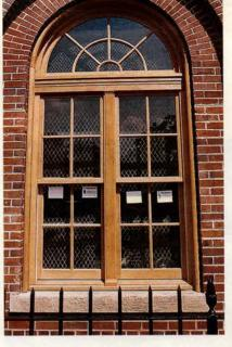
This double-hung window unit with a fixed-arch fan was constructed by Artistic Doors & Windows with mortise-and-tenon joinery.
