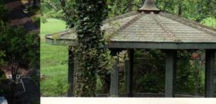
This gazebo features W.F. Norman Corp's style A shingles with its continuous hip finish and a custommade finial on top.
