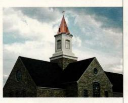
This prefabricated steeple with a copper spire and cross was fabricated by Munns Manufacturing for the Horizon Community Church in Cincinnati, OH.
