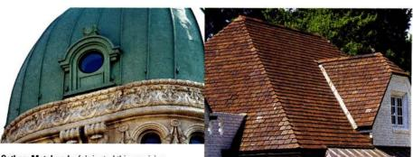
Gotham Metalworks fabricated this precision plasma-cut replication domed roof for a N.Y.C. landmarked building.
