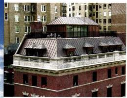
NIKO fabricated the copper dormers and mansard roof and also installed the copper penthouse for this building in New York City.
