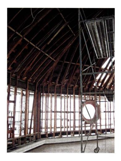
ABOVE: Now restored, the 44-ft. tall upper rotunda was completely rebuilt. The badly damaged decorative plaster was restored and lighting was enhanced by creating a light box where the original skylight had been.
