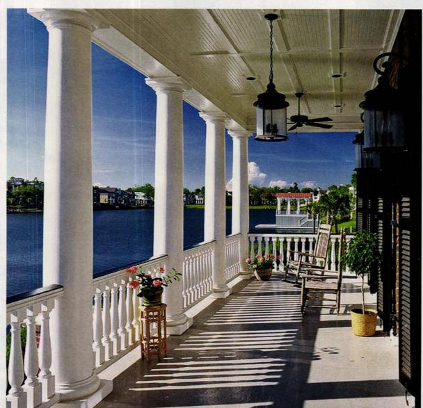
FAR LEFT: The MeltonCraft CPVC columns are crafted from cellular PVC and come in L sections for easy assembly around structural supports.
