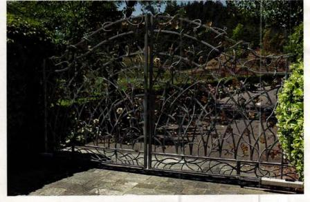
Designed and fabricated by Wiemann Metalcraft, this wrought-iron gate features repousse and gilded-brass leaves and roses.
