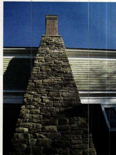
Reclaimed stone from a historic reservoir was paired with antique Purington Street pavers from Gavin for this chimney in Iowa City, IA.
