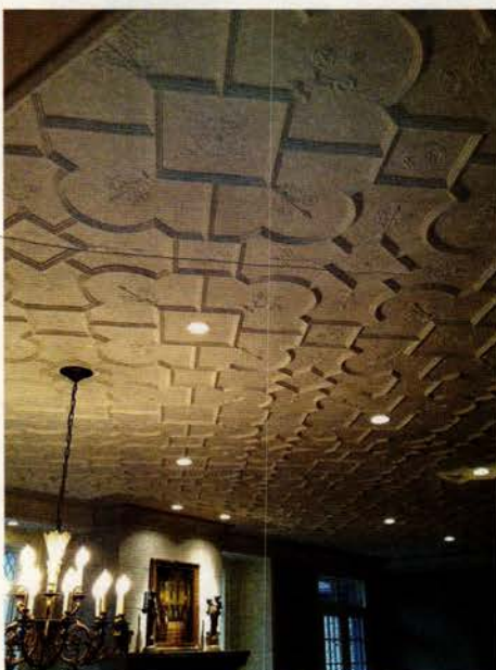
This Old English ceiling was created using hand-cast plaster panels from Decorators Supply.
