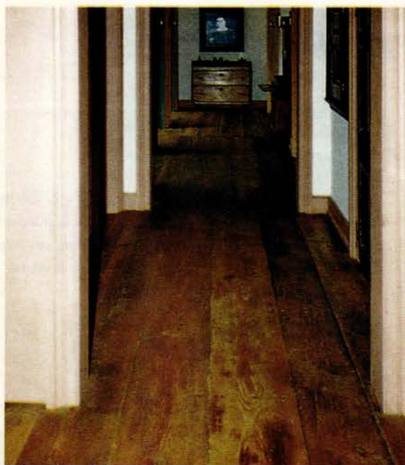
Resawn flooring from Sylvan Brandt is cut from old beams to match the grain and character of antique floors.
