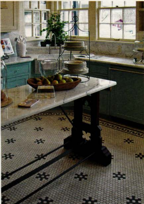
This historically accurate floor was created using 1-in. hexagon unglazed porcelain tile and 3/4-in. square border tile from American Restoration Tile.
