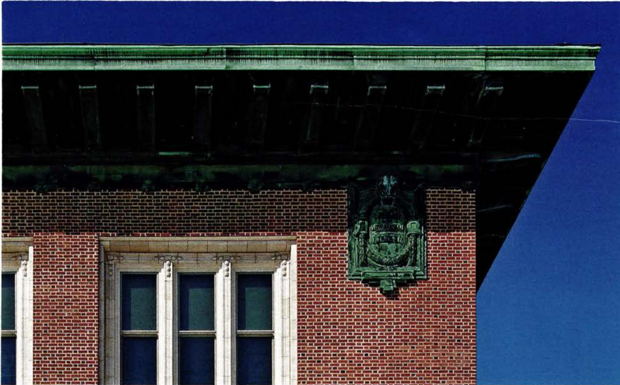
LEFT: An in-depth study was conducted to examine the comparative efficacy of whether to restore or replace existing windows. As maintenance cost was the primary driver, UIUC elected to replace windows with wood-clad aluminum windows. Photo: Dave Burk at Hedrich Blessing
