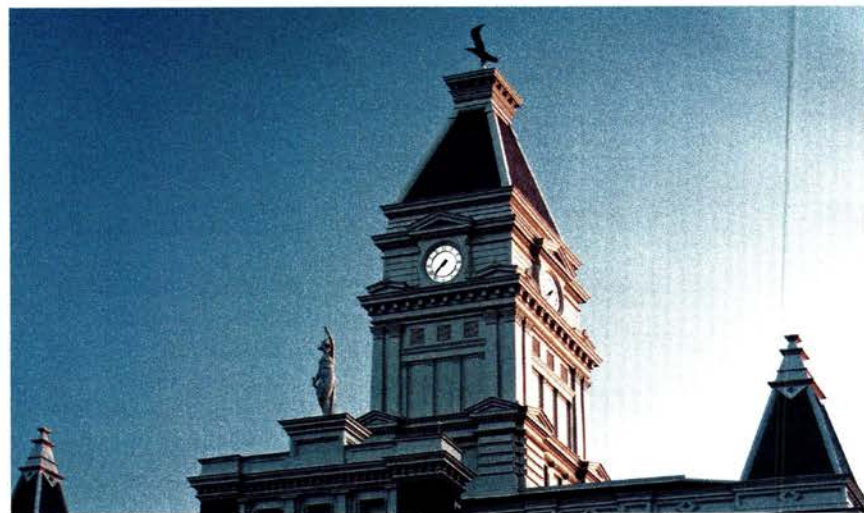
Campbellsville Industries fabricated the clock tower, clock, decorative cornice, modillions, paneled railing and corner pediments for the restoration project at Montgomery County Courthouse in Clarksville, TN.
