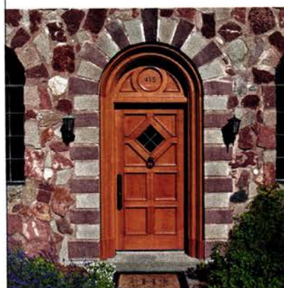
HeartWood Fine Windows & Doors fabricated this 2 1/4-in. thick mortise-and-tenon solid-wood door out of saun white oak to replicate the original door made 100 years ago.
