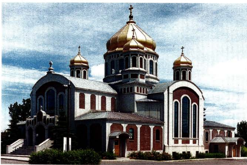
The original exposed concrete domes of St. John the Baptist Church in Ottawa, ON, Canada, were clad with pre-painted sheetmetal by Heather & Little.
