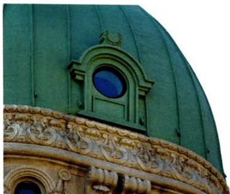
Gotham Metalworks fabricated this precision plasma-cut replication domed roof for a NYC landmark building.
