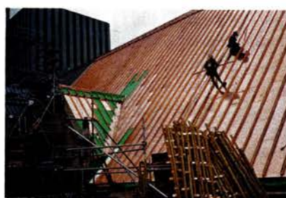
Heather & Little restored the copper roofing for Toronto's City Hall.
