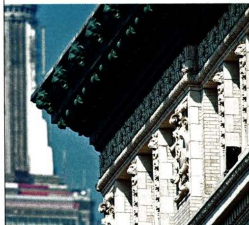
This ornate cornice was fabricated by Gotham Metalworks for an historic building.
