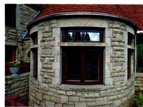
HeartWood supplied the replacement windows for this 100-year-old gatehouse in Rochester, NY; they are made of quarter-sawn white oak and bent glass.
