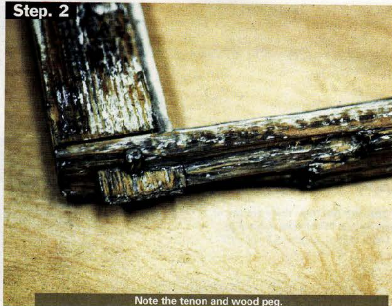
Note the tenon and wood peg.
