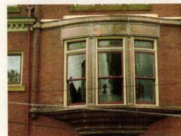
NIKO Contracting Co. fabricated and installed this custom copper radiused bay window system.
