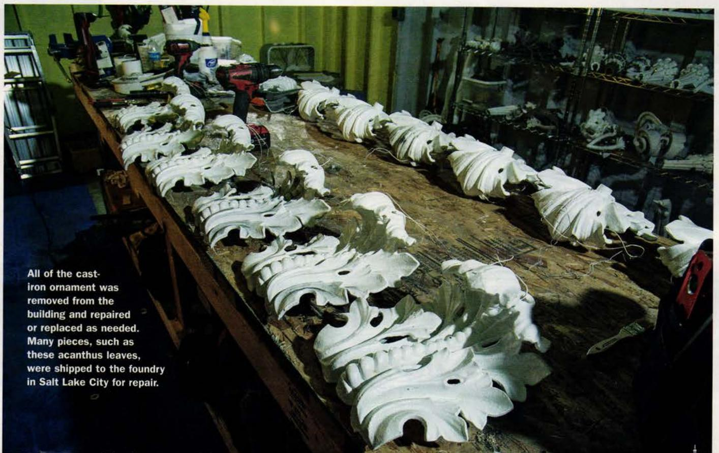
All of the cast-iron ornament was removed from the building and repaired or replaced as needed. Many pieces, such as these acanthus leaves, were shipped to the foundry in Salt Lake City for repair.
