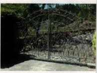
Designed and fabricated by Wiemann Metalcraft, this wrought-iron gate features repousse and gilded-brass leaves and roses.
