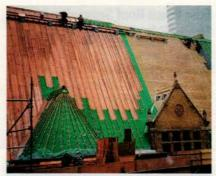
Heather & Little's restoration of the Toronto Old City Hall required 113,900 sq.ft. of copper roofing, cornices, gutters and sheet-lead work.
