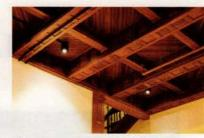
This custom wood paneled ceiling/trim was created by Heritage Restoration using a mixture of new and restored wood sections.
