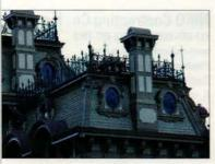
en Architectural Metals fabricated this al roof for the Stanford Mansion in California
