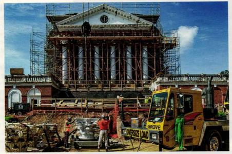
LEFT: Temporary steel shoring was erected to support the portico roof structure during the removal and replacement of the marble column capitals. The copper sheet metal cornice installed by Stanford White following the disastrous 1895 fire, was removed, stripped of paint, refinished and reinstalled on restored cast-iron framing brackets. The existing north marble stair was dismantled, cleaned, repaired and re-installed above a new waterproof membrane protecting the building construction below.
