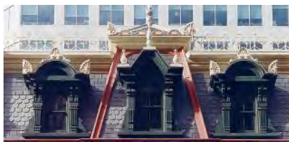
Custom finials from W.F. Norman were incorporated into the restoration design of this historic building in Toronto.
