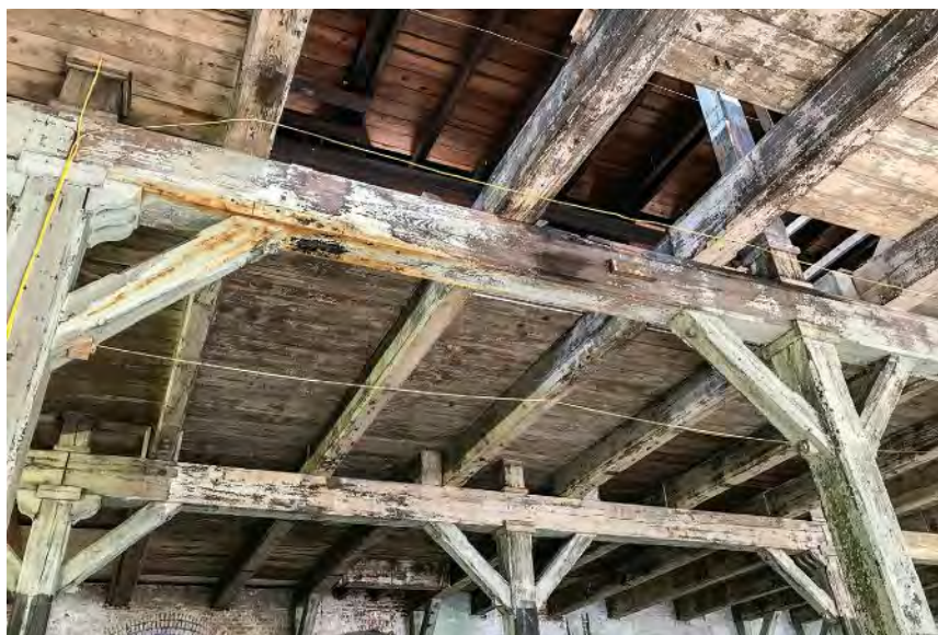
Classic 19th-century mill construction of heavy timbers supports the second floor but with ample capacity for a new life in a new purpose.
