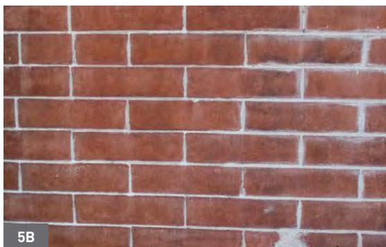
5B A narrow mortar joint was partially repointed, using too thick of a saw cut, resulting in widening of the joint.
