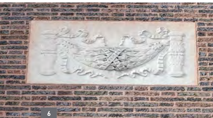
6 Unstable colorant was used in the mortar, resulting in staining of the stone work.
