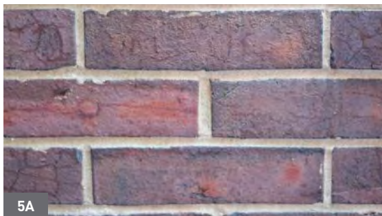
5A Note the nicks at the tops and bottoms of vertical joints where a masonry saw nicked the bricks, and the chips along the edges where poorly executed removal of the mortar led to damage.
