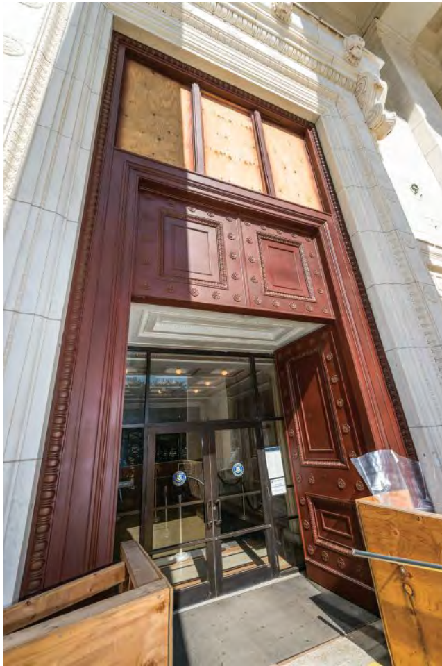
Several original bronze exterior doors had been replaced in years past. New doors were perfectly reproduced in bronze to match an existing original pair (left).
