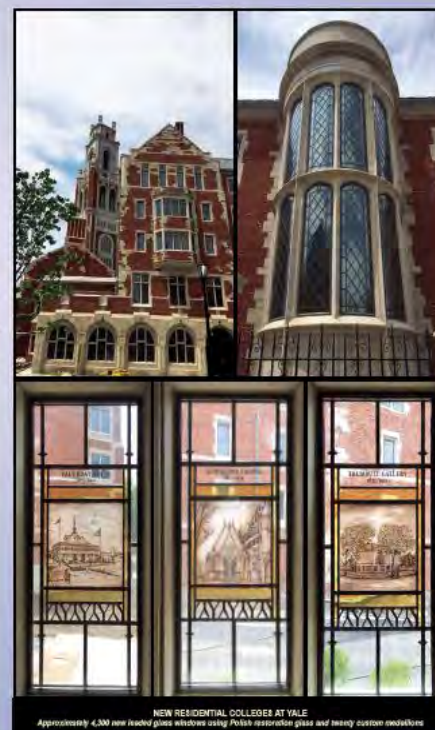
NEW RESIDENTIAL COLLEGES AT YALE Approximately 4,300 new leaded glass windows using Rohlf's restoration glass and many custom medallions
