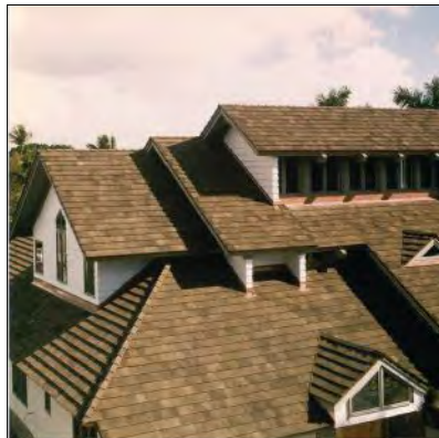
This building features light-weight ceramic tile with the look of cedar by Ludowici .
