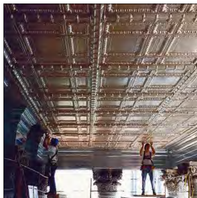
Niko Contracting replicated and installed the pressed-metal ceiling panels and cornice for the South Carolina State House in Columbia, SC.
