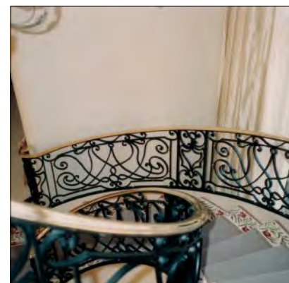
This forged-iron railing and polished-bronze cap rail were designed, fabricated, finished and installed by Wiemann Metalcraft .
