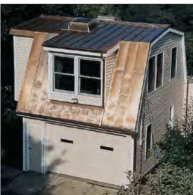
NIKO Contracting installed the copper standing-seam roof on this carriage house.
