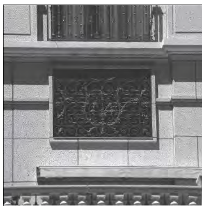
Historical Arts & Casting manufactured this 4x7-ft. cast-aluminum return-air grille with a painted finish for the Grand America Hotel in Salt Lake City, UT.
