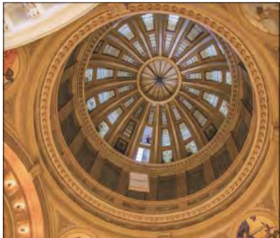
Conrad Schmitt Studios removed, conserved, re-leaded and reinstalled the stained-glass of the South Dakota State Capitol; the glass in the rotunda dome and the glass in the barrel-vaulted ceiling went through the extensive conservation process.
